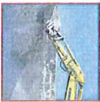
AQ-4 removing layer of concrete from bridge, mounted on a Hitachi 30 ton excavator
