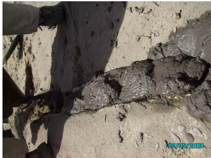
Figure 5.7: Paste backfill placement in fracture
