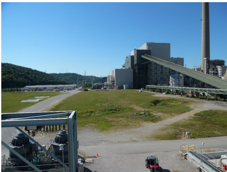
CCRT Project Area Looking South
