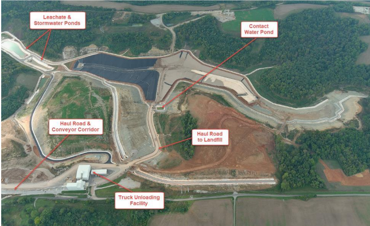
CCR Landfill Overview – View Looking North October 2021
