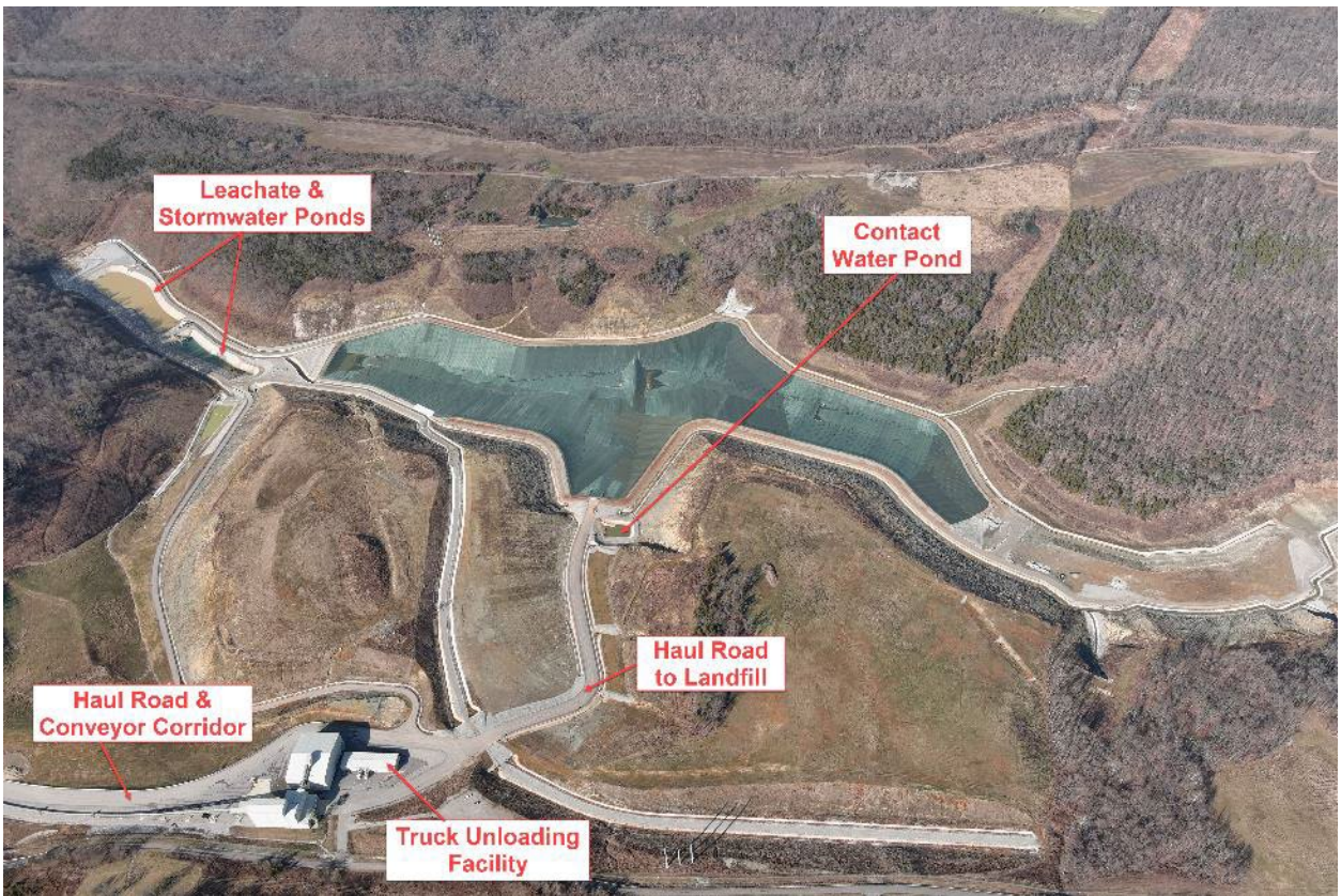
CCR Landfill Overview – View Looking North December 2022
