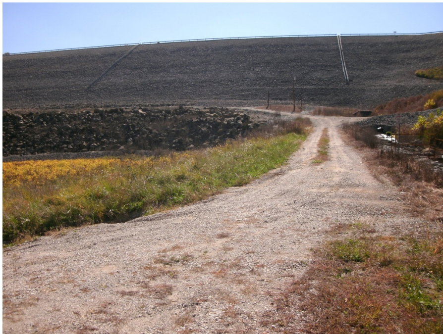
Plate 3.10. Overview of the Dam within the APE (photo taken north of the dam).
