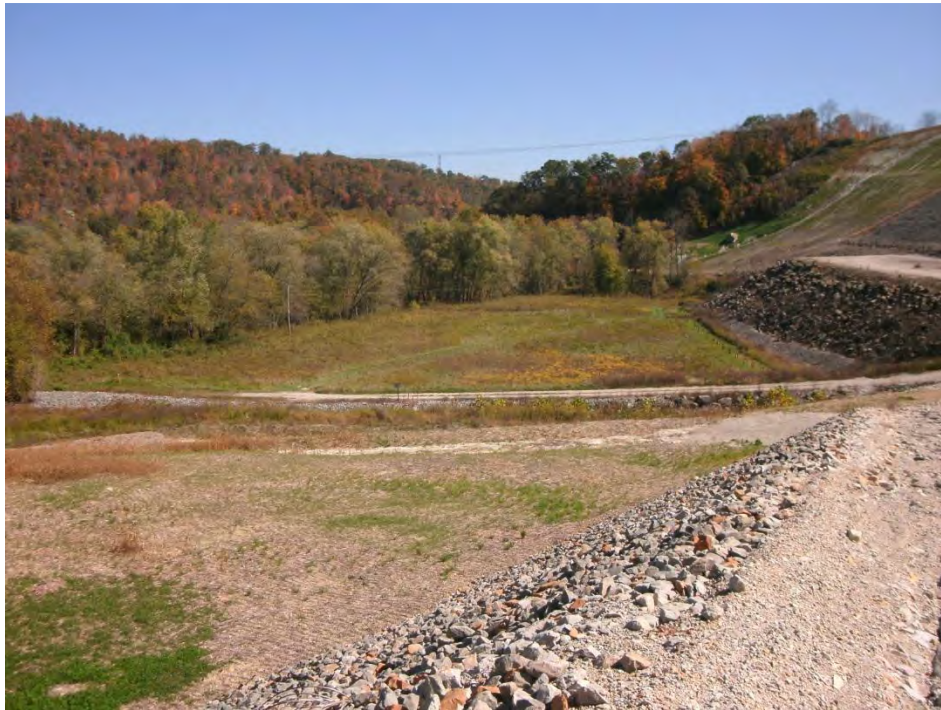
Plate 3.11. Overview of the APE just north of the Dam.
