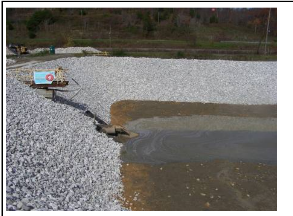
Decant structure (platform near top of slope) and pond drain (pipe near bottom of slope) from south Bottom Ash Pond into south Clearwater Pond.
