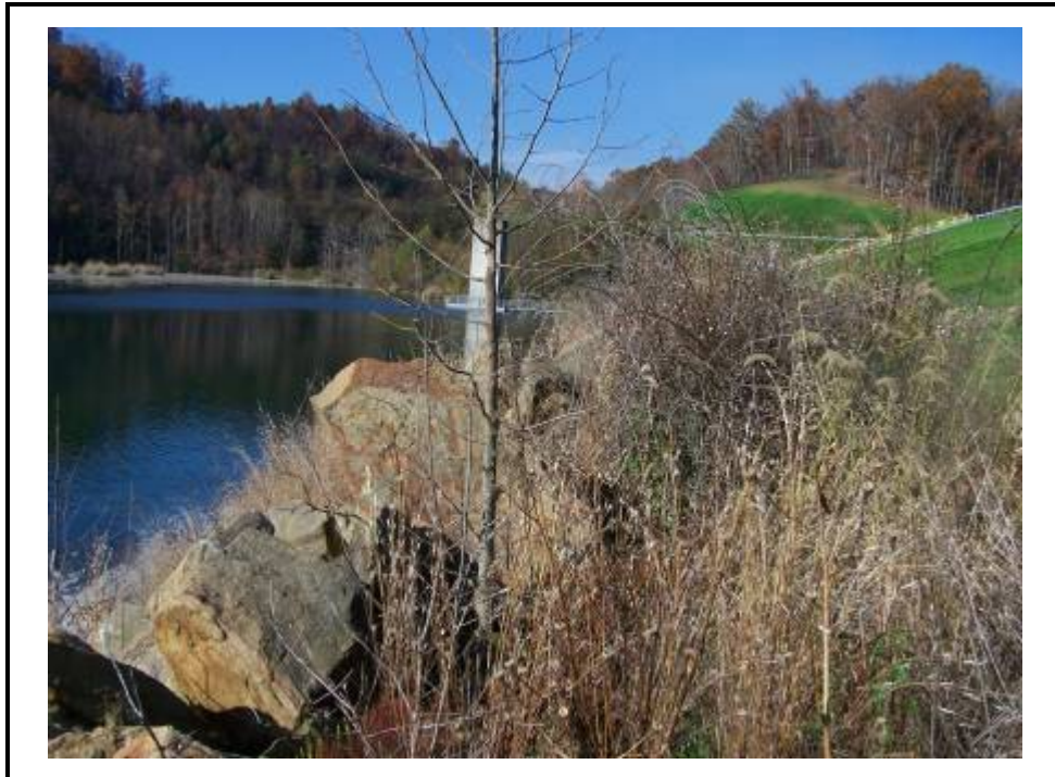
Brush and small trees in rip rap along the water line have been sprayed with herbicide at Horseford Dam.
