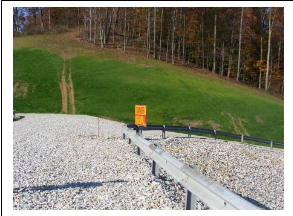
West abutment of Horseford Creek Dam, looking west.
