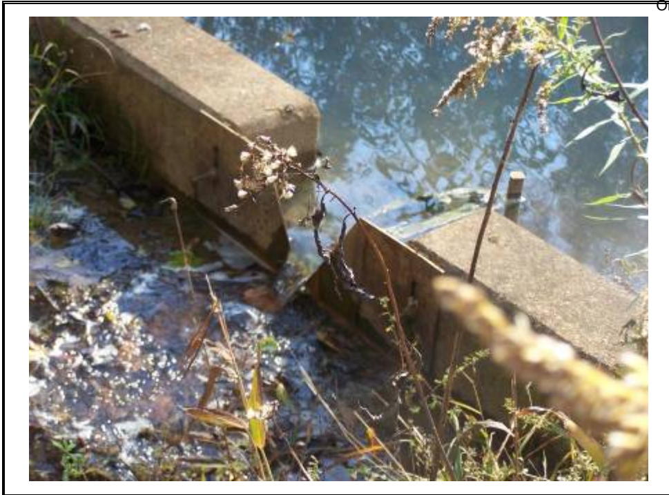
Monitoring weir at east abutment and toe drain discharge area.
