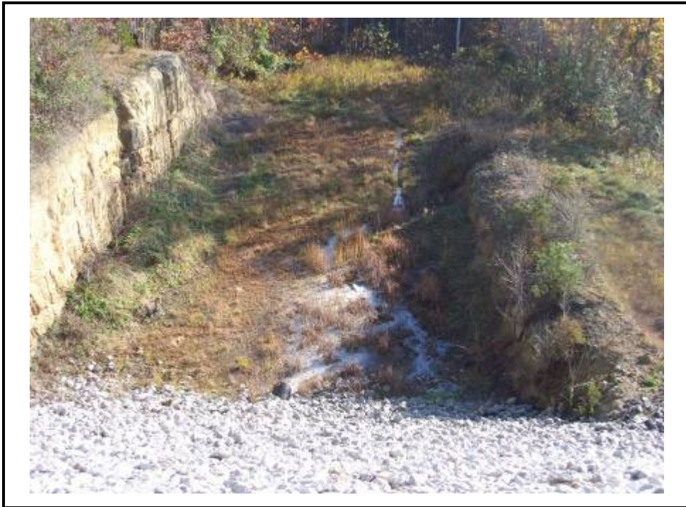
Original emergency spillway. Seepage drain at approximate midpoint of channel.
