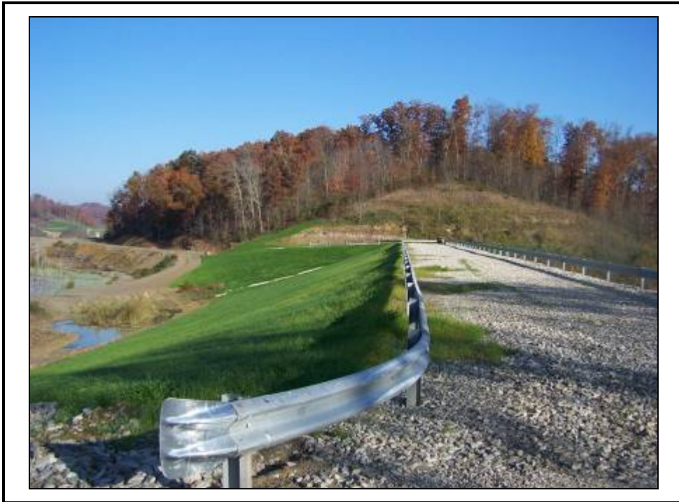
Crest and upstream slope of Saddle Dam, looking north.
