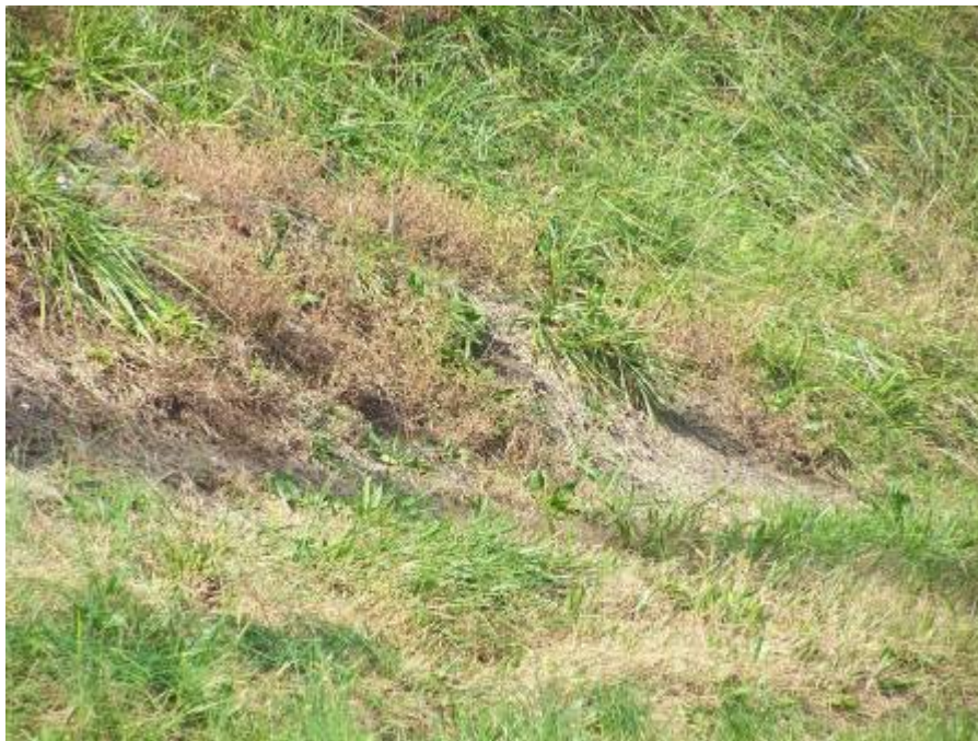
Minor sloughing or erosion on downstream slope of East Dike.
