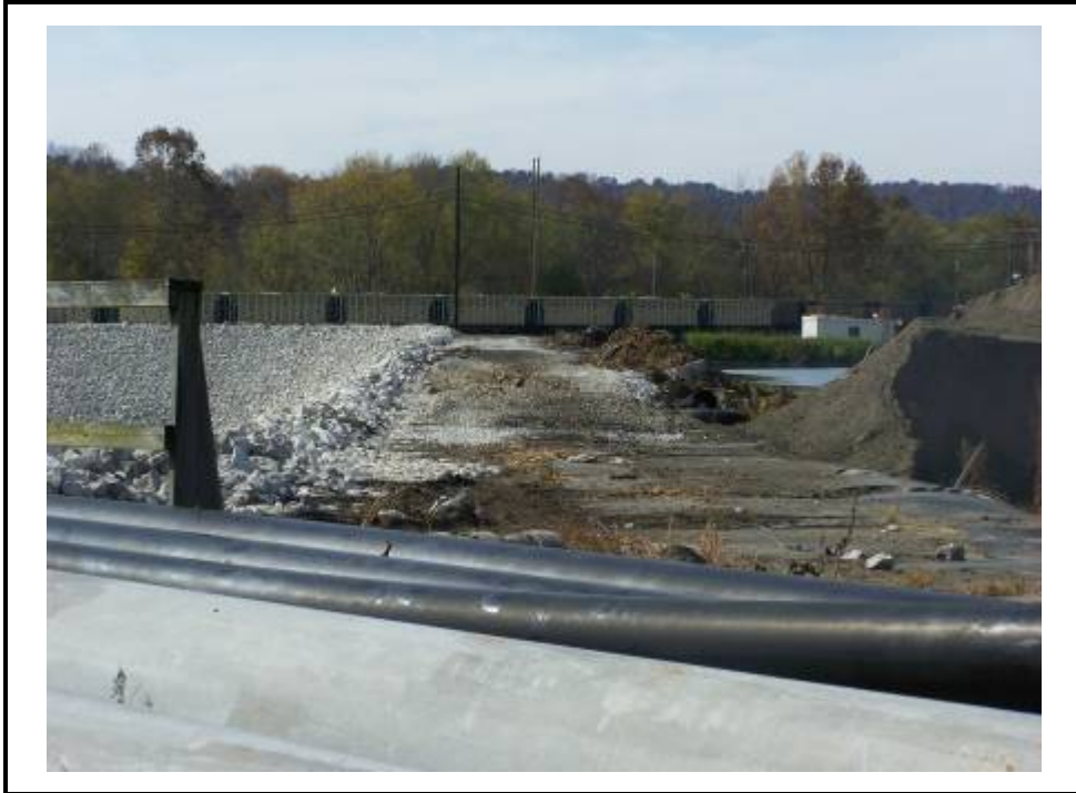
Crest of Splitter Dike between south Bottom Ash and south Clearwater Ponds.
