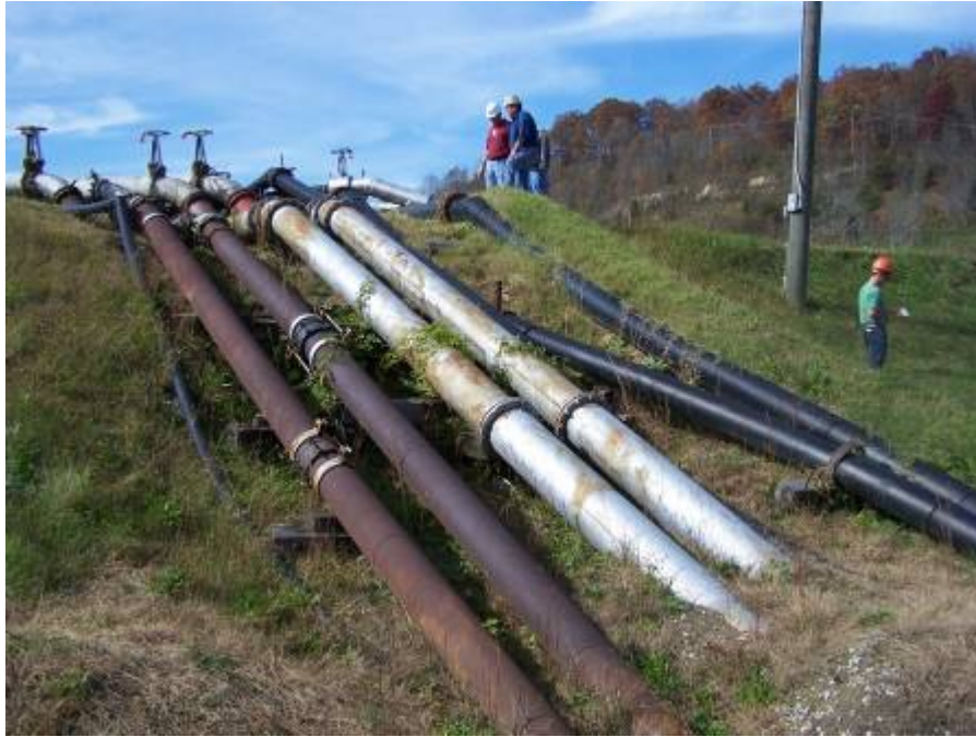
Sluice lines on downstream slope of East Dike.
