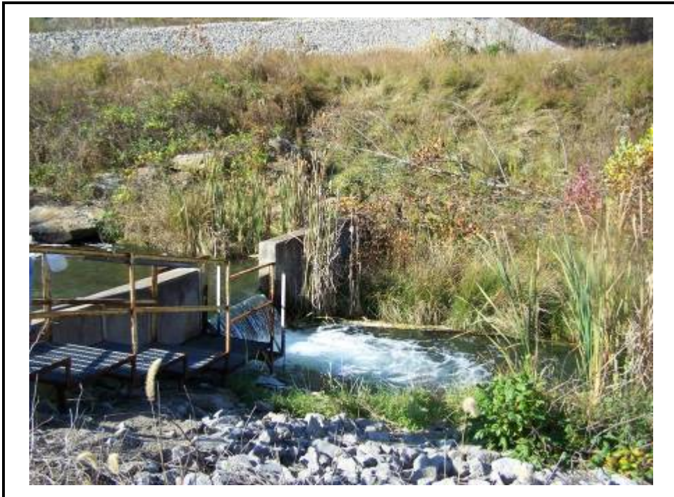
Stilling basin and NPDES outfall for Horseford Creek Dam outlet.
