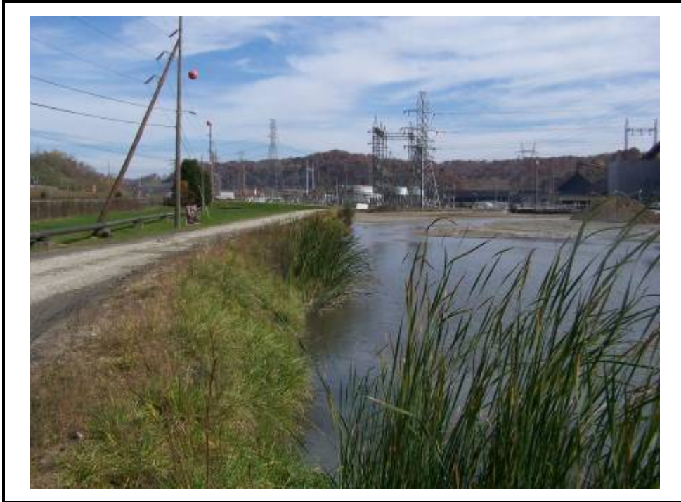
Upstream slope of North Dike at the Bottom Ash Complex adjacent to north Bottom Ash Pond, looking east.
