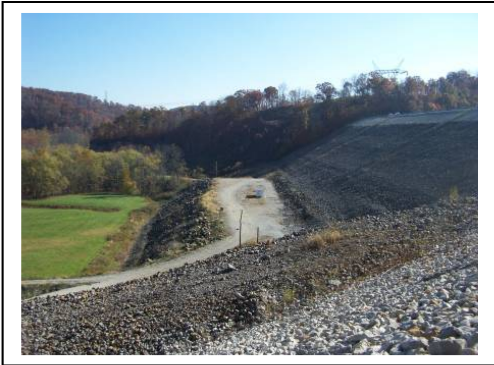
Downstream slope and buttress of Horseford Creek Dam, looking east.
