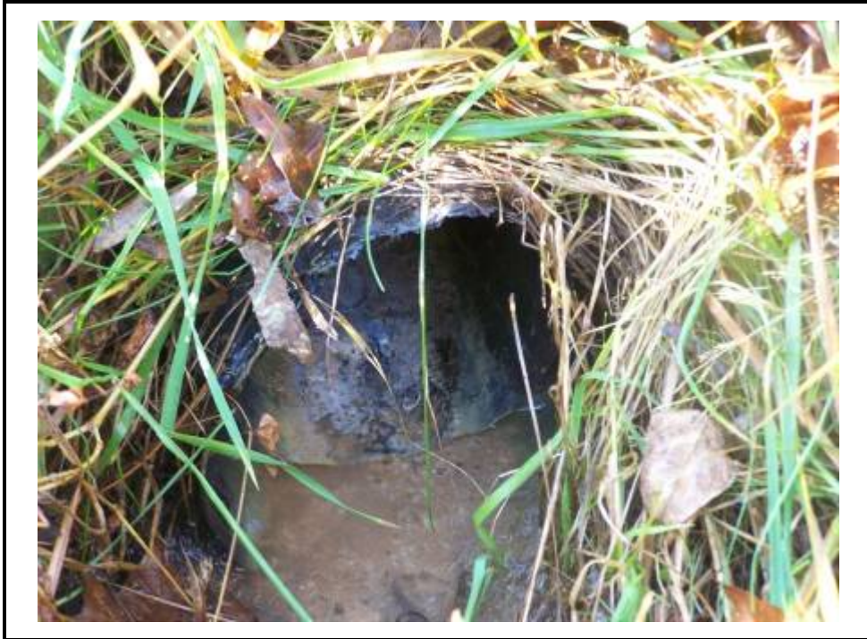
Toe drain outlet after clearing vegetation.
