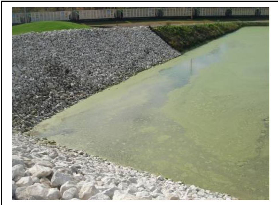
Upstream slope of South Dike of Bottom Ash Complex at south Clearwater Pond, recently placed rip rap protection at east end.
