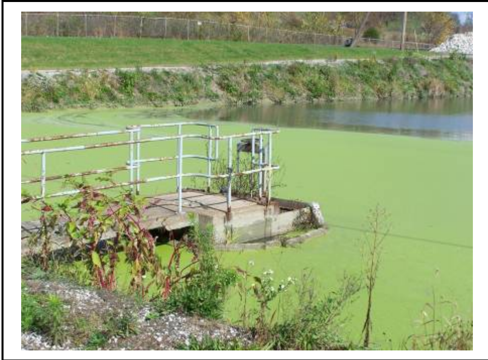
Discharge structure from north Clearwater Pond to Reclaim Pond and upstream slope of North Dike of Bottom Ash Complex. Note crest of North Dike slopes down to the west.
