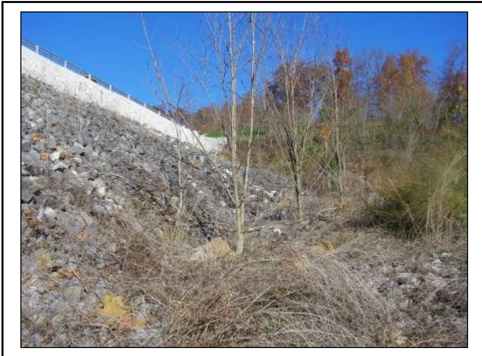
Close-up of trees in north downstream groin.
