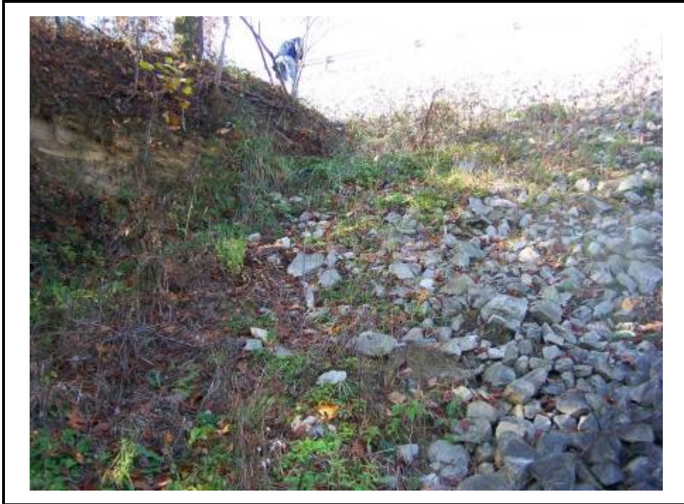
South groin of downstream slope and abutment at Saddle Dam.
