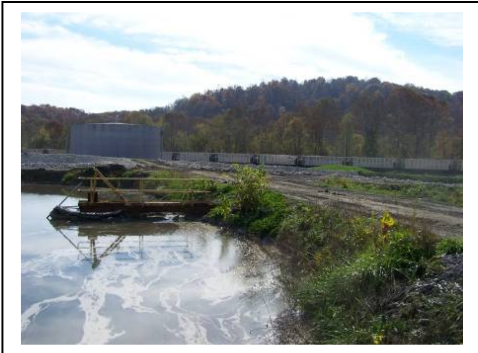
East slope of Splitter Dike between north Bottom Ash and Clearwater Ponds and decant structure.
