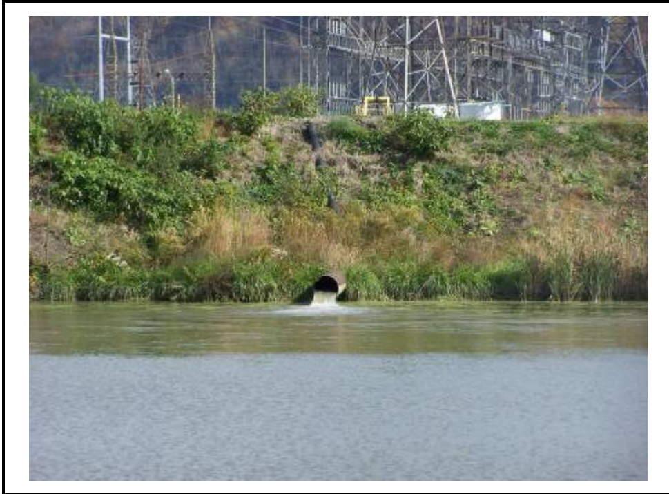
West slope of Splitter Dike between North Bottom Ash and Clearwater Ponds showing discharge pipe from North Bottom Ash Pond.
