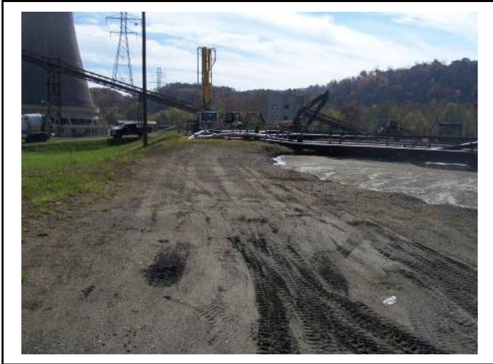
Crest of East Dike of the Bottom Ash Pond, looking south.
