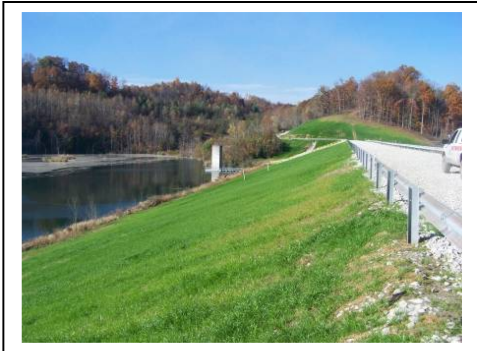
Upstream slope of Horseford Creek Dam, looking east.
