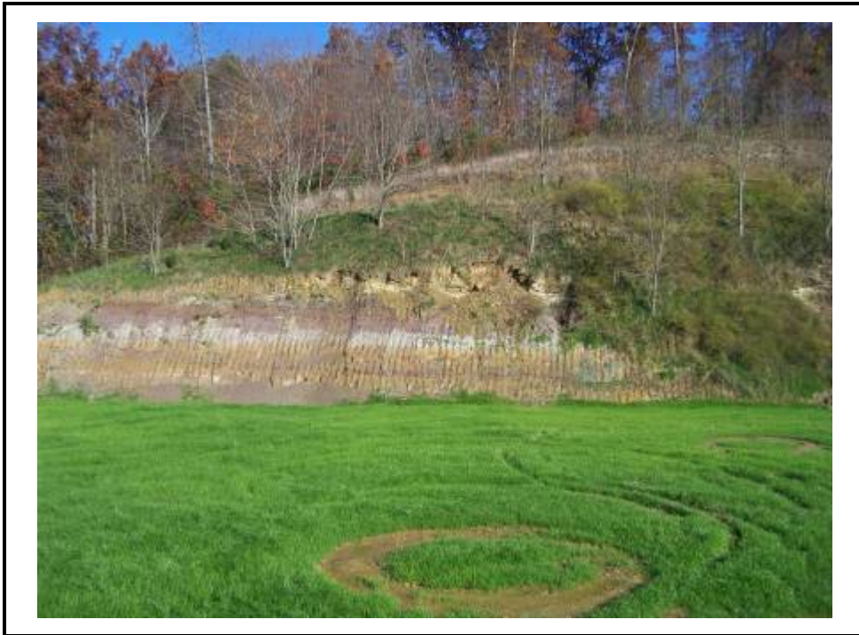
North abutment contact of “new” emergency spillway.
