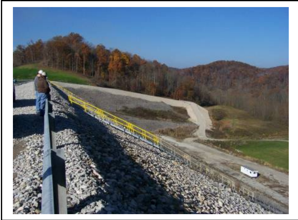
Downstream slope Horseford Creek Dam, looking west.
