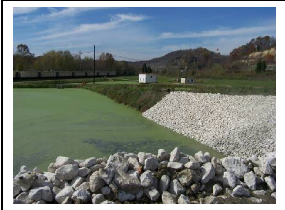
South side of Splitter Dike between south and north Clearwater Ponds.
