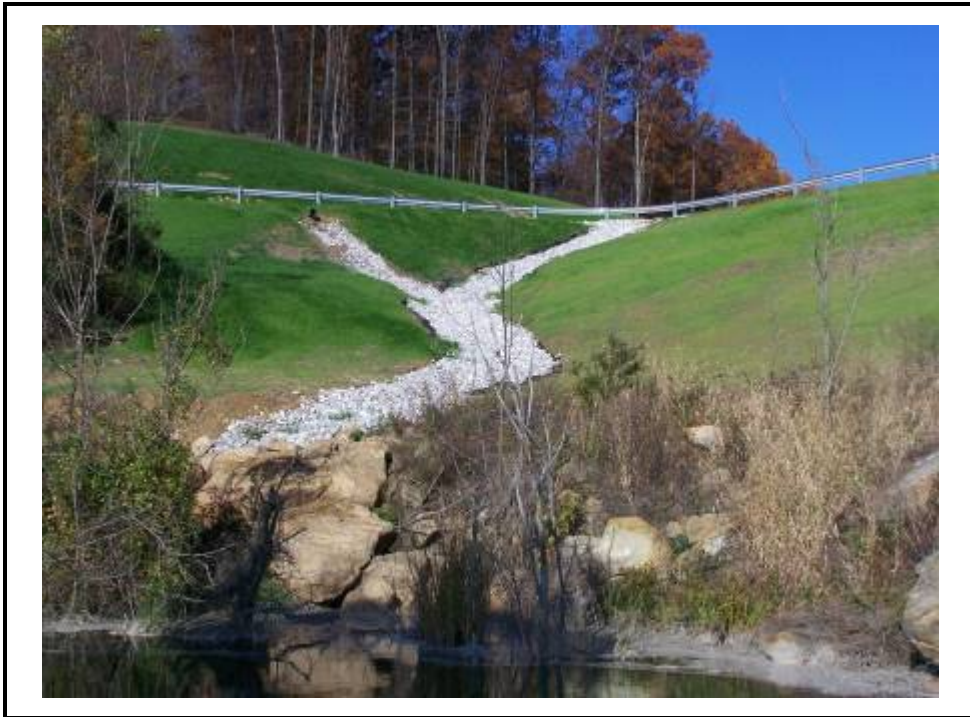
Upstream west abutment groin and large rip rap at Horseford Creek Dam.
