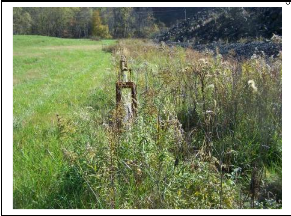
Relief wells part of Horseford Creek Dam toe drain system. Area in taller grass is wet from seepage.
