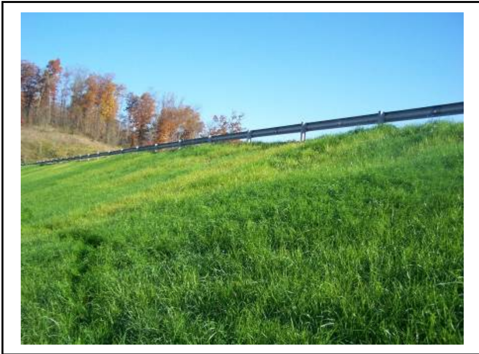
Irregularity to grading at upstream slope/crest intersection on Saddle Dam.
