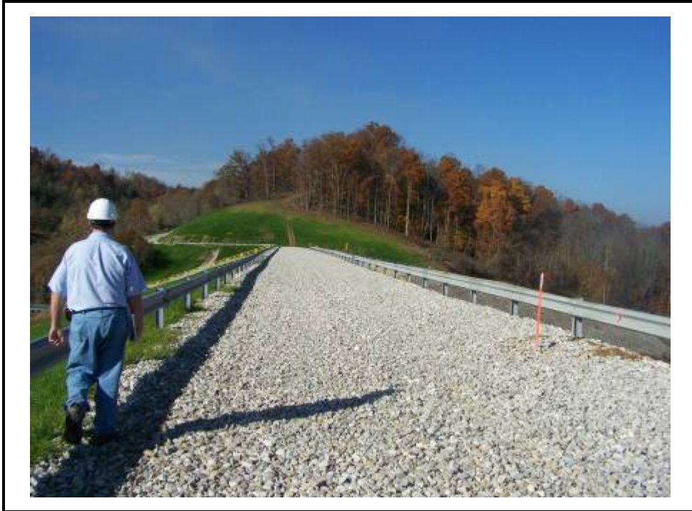
Crest of Horseford Creek Dam, looking east.
