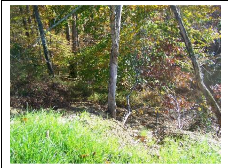
Downstream condition of "new" emergency spillway.
