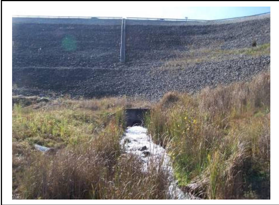
Discharge pipe at toe of Horseford Creek Dam. Stairs on slope provide access to instrumentation.
