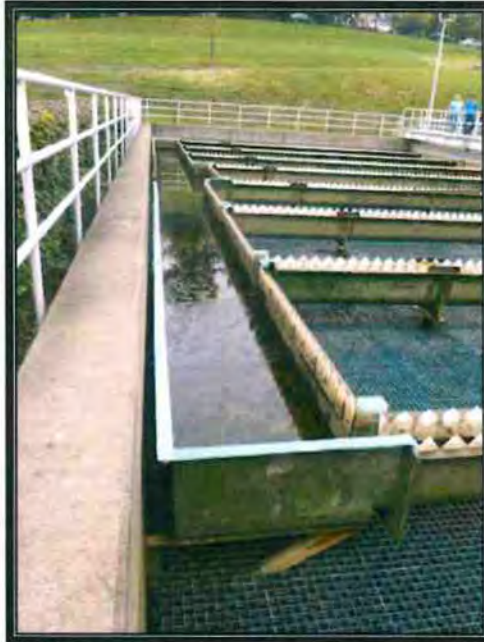
Photo 10 - Basin #1 Clarifier Effluent Channel
