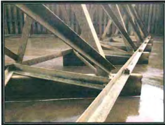
Photo 15 - Basin #2 / #3 Clarifier Sludge Rake (Typ.) Photo 16 - Basin #2 / #3 Effluent Sluice Gate Operators (Typ.)
