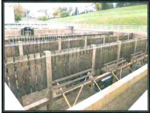
Photo 2 - Basin #1 Flocculation Zone
