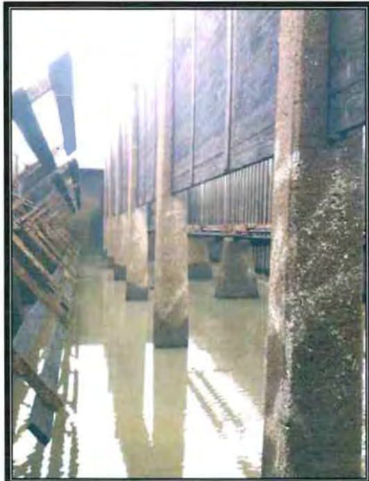
Photo 19 - Basin #1, #2, #3 Baffle Wall (Typ.)
