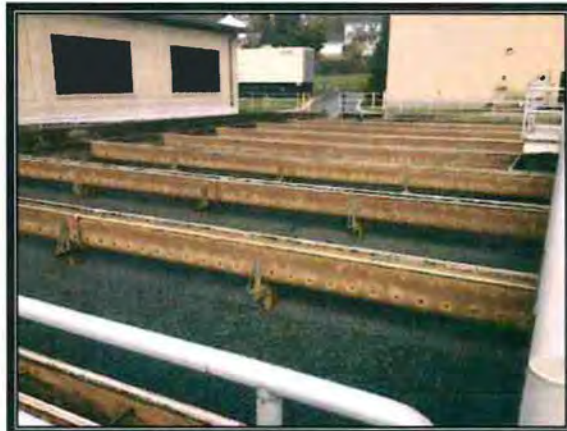
Photo 12 - Basin #2 / #3 Tube Settlers (Typ.)
