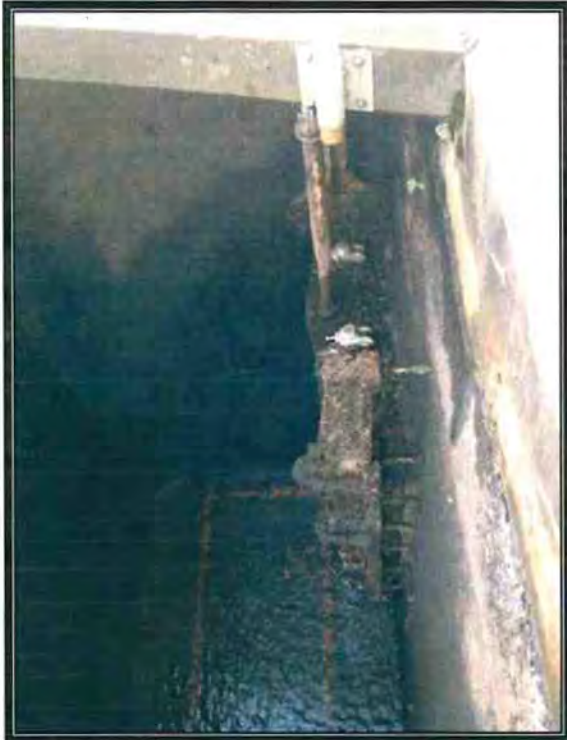
Photo 17 - Basin #2 / #3 Effluent Sluice Gate (Typ.)
