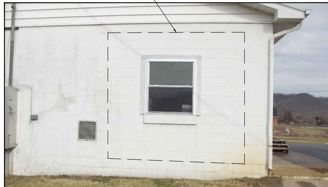
DEMOLITION - OUTSIDE VIEW
