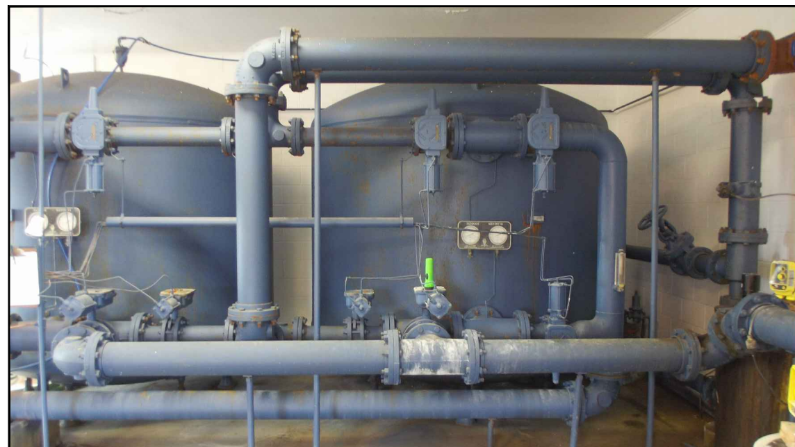
DEMOLITION - FILTERS AND PIPING
