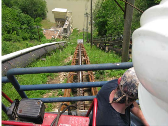
Tram and Intake
