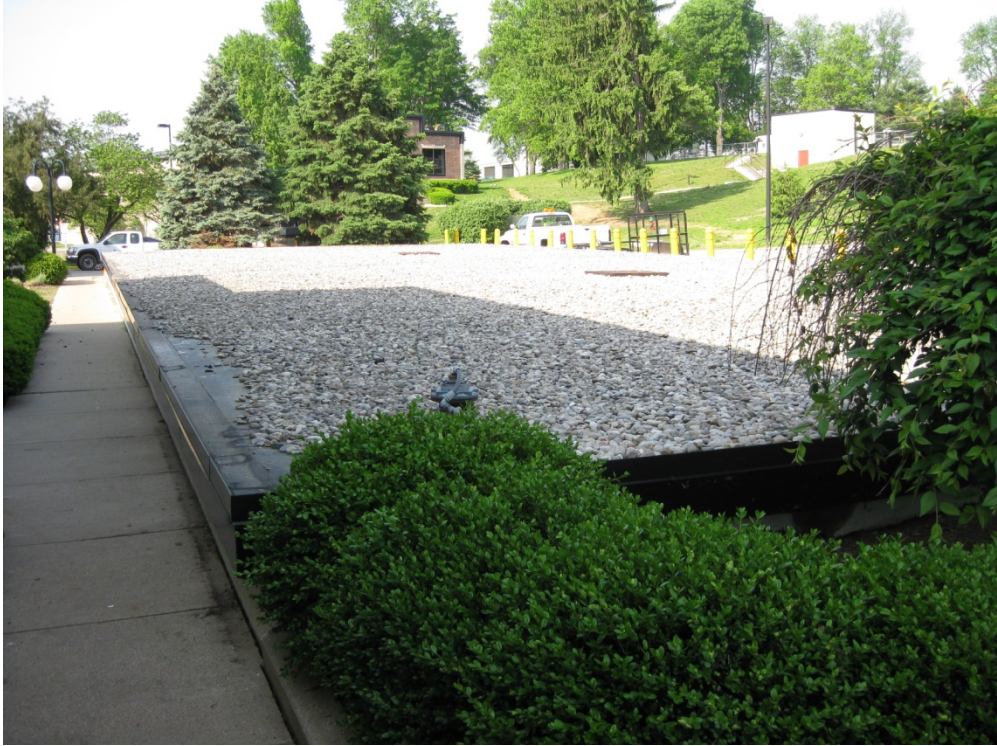
Richmond Road Station – Clearwell #2
