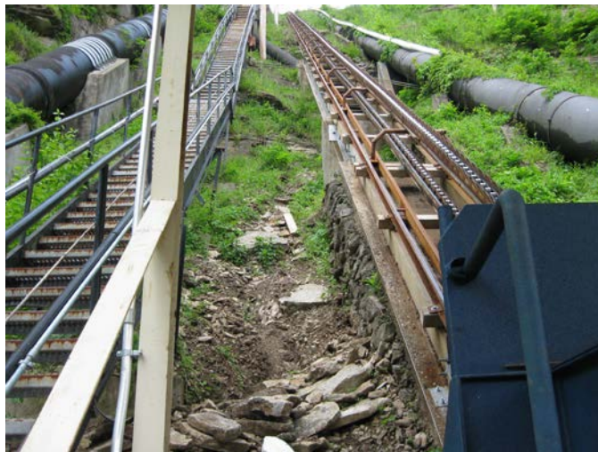
Raw Water Lines
