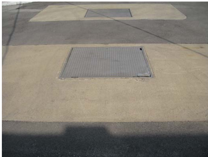
Valve Vault Clearwell to “tank over the hill”
