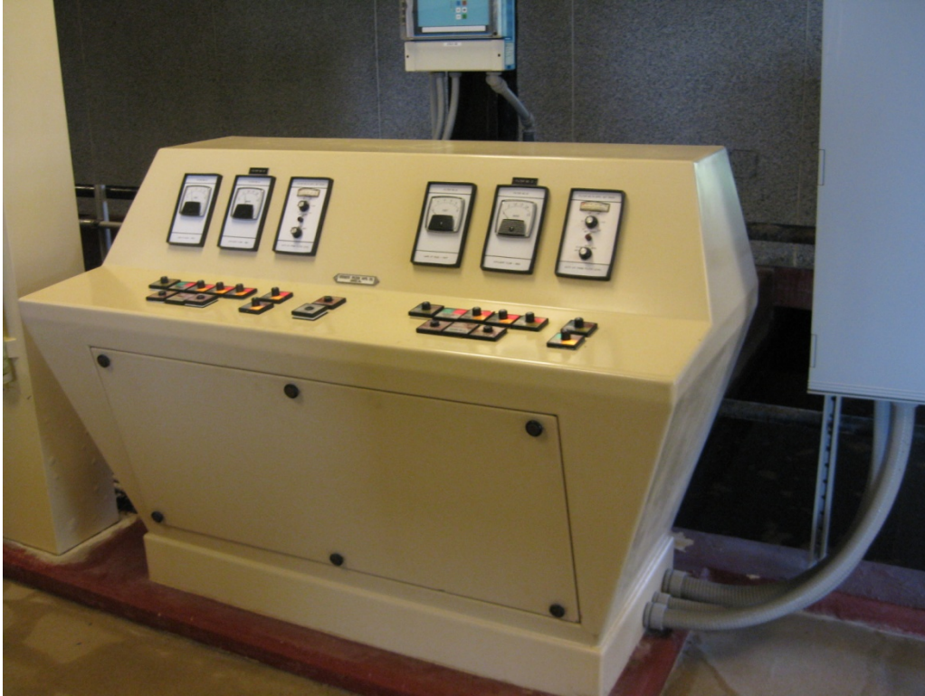
Richmond Road Station - Filter Controls
