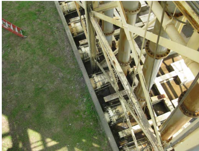
Raw Water Discharge Piping
