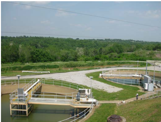
Waste Water Basins & Sludge Lagoons
