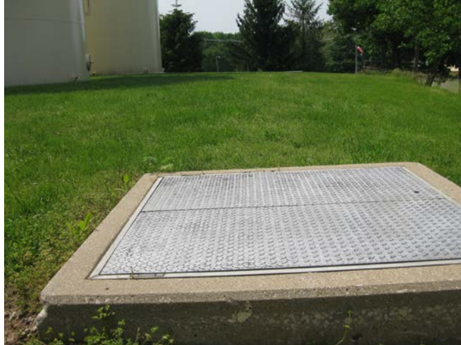
Valve Vault Rapid Mix to Hydrotreator
