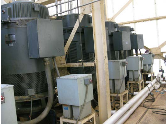
Raw Water Pump Motors
