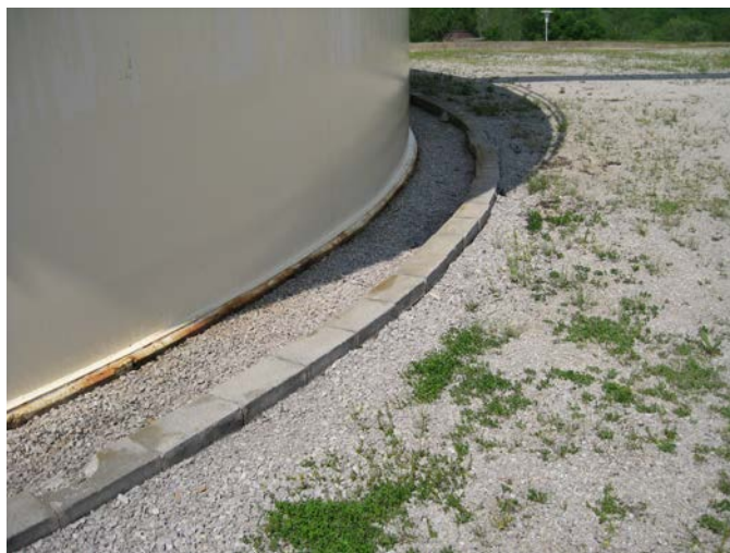
Ring Foundation Hydrotreater
