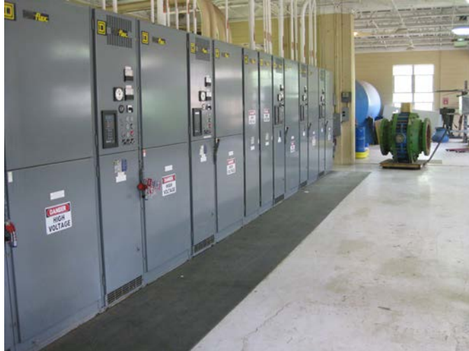
Raw Water Switchgear
