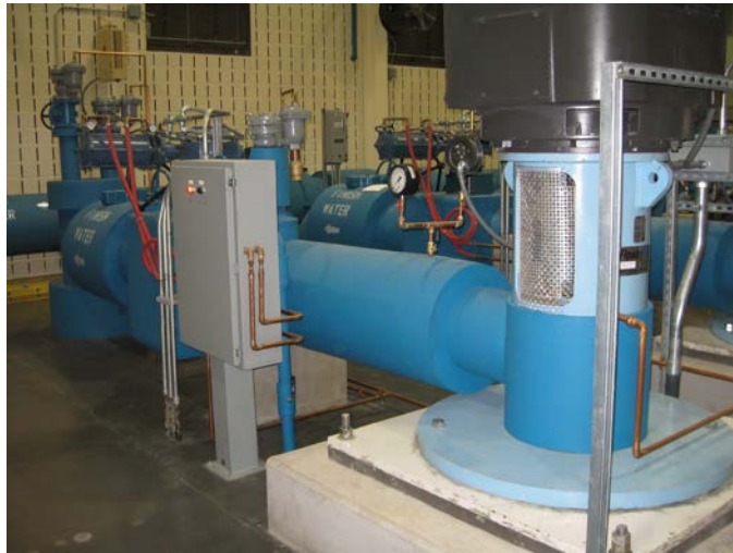
High Service Pumps
