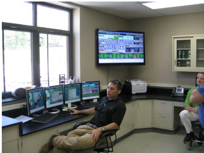
Main Control Room
