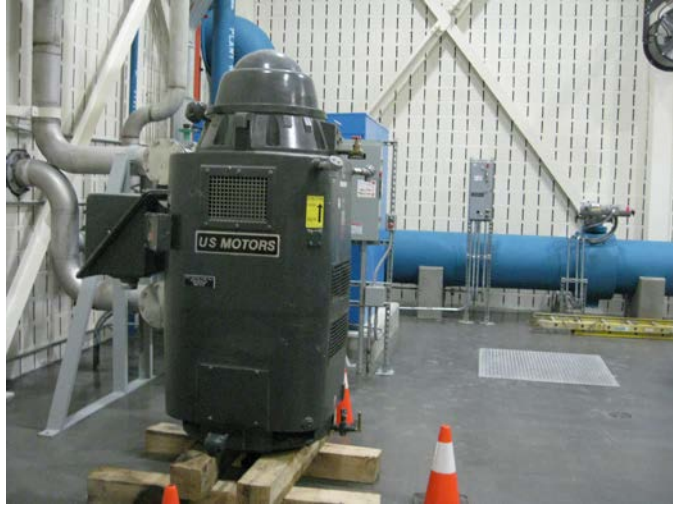
High Service Pumps
