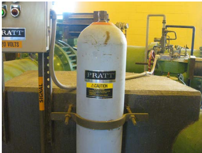
Raw Water Transfer Pumps
