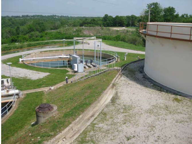
Waste Water Basins
