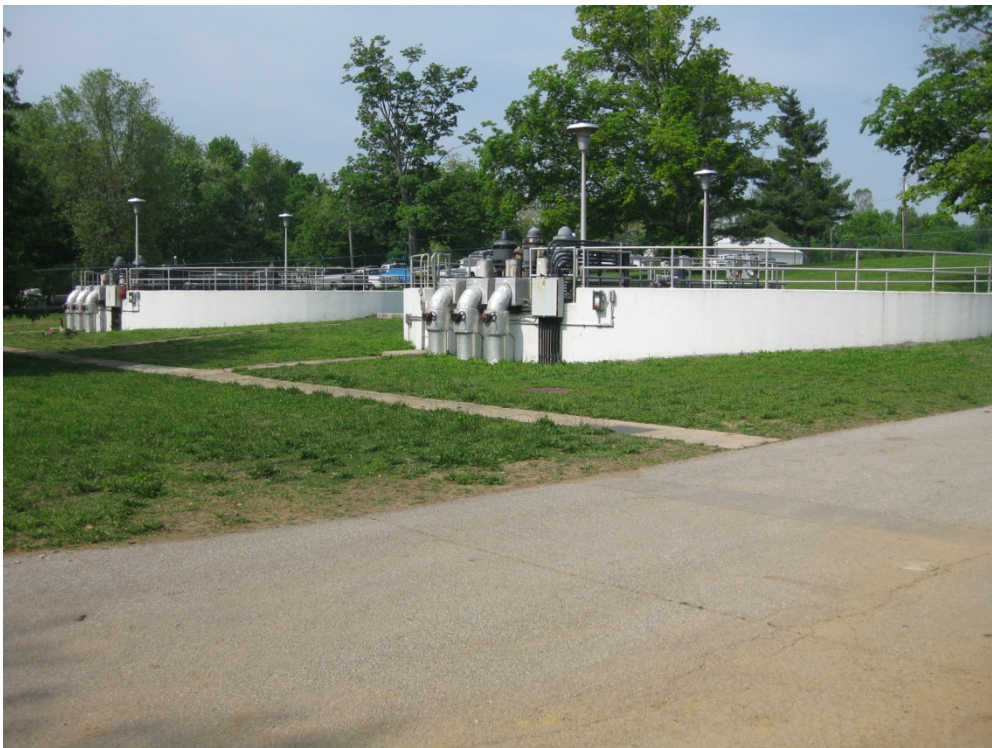
Richmond Road Station – Washwater Holding Tanks
