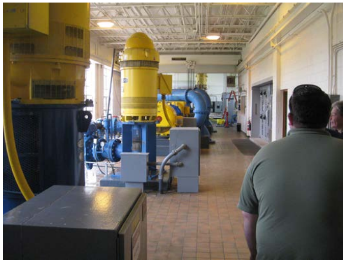
High Service Pumps
