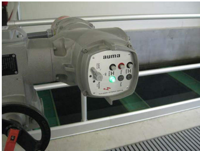
Filter Influent Valve
