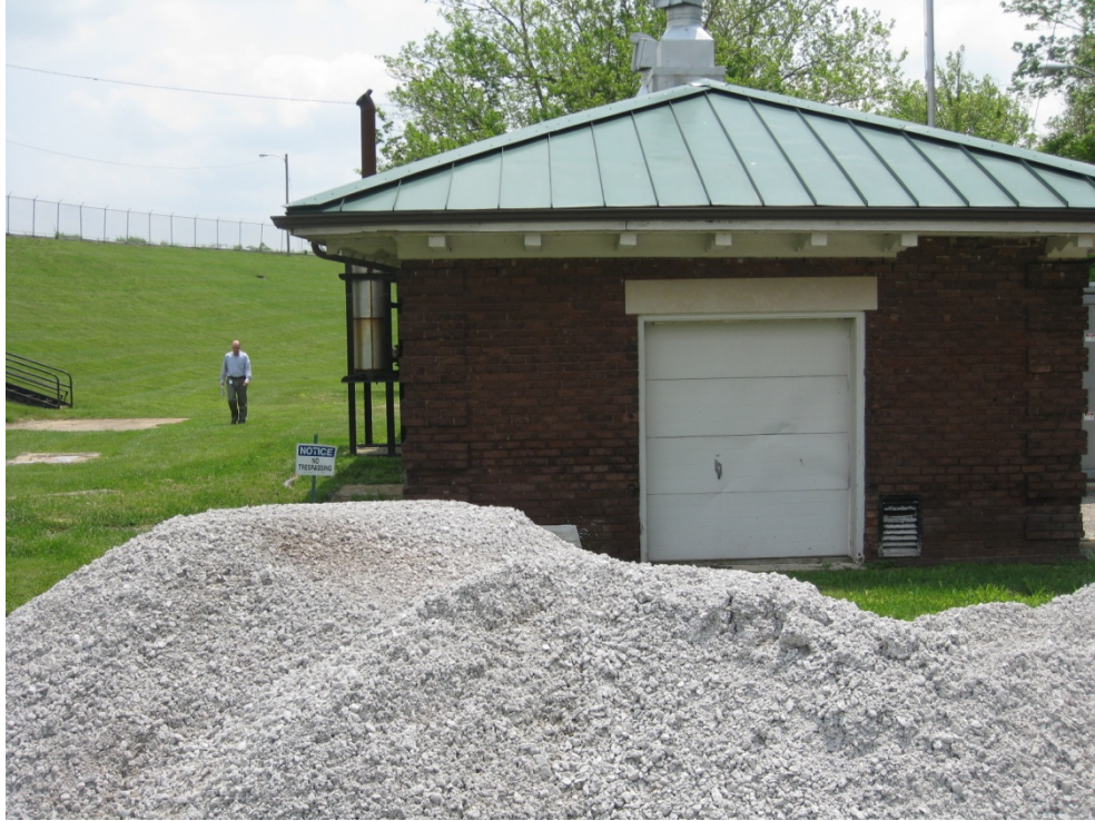
Jacobson Reservoir – Pump Station to Richmond Road Station
