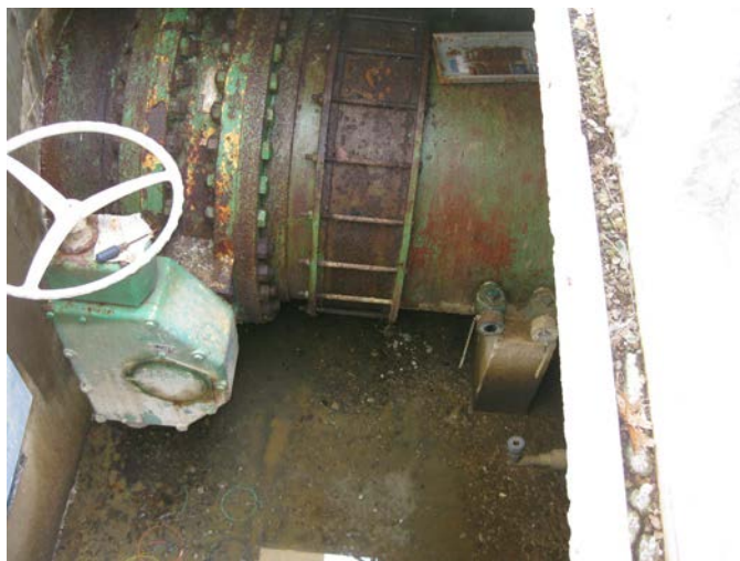
Valve Vault Rapid Mix to Hydrotreator
