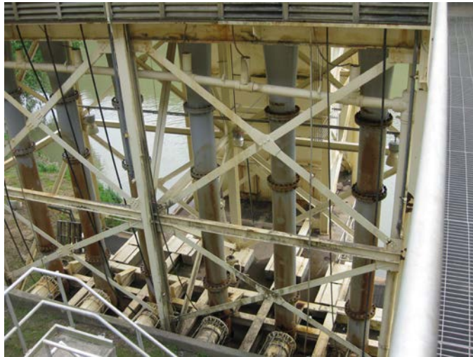
Raw Water Pump Shafts
