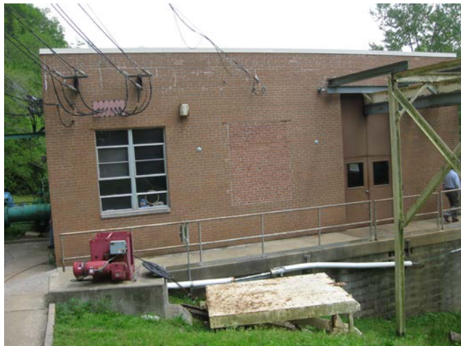
Raw Water Pump Station Electric Building
