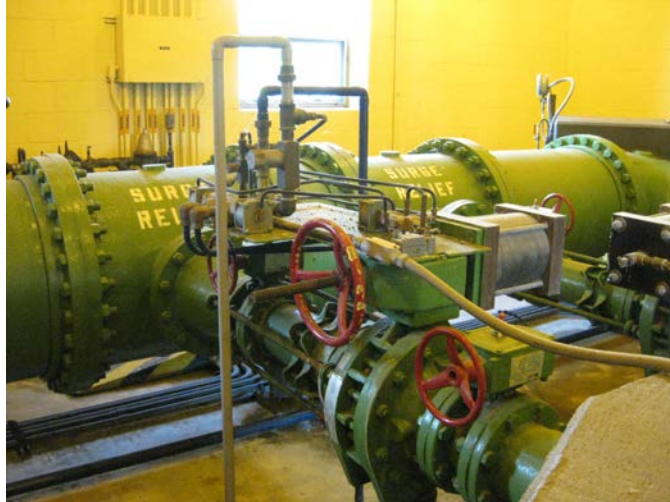
Raw Water Transfer Pumps
