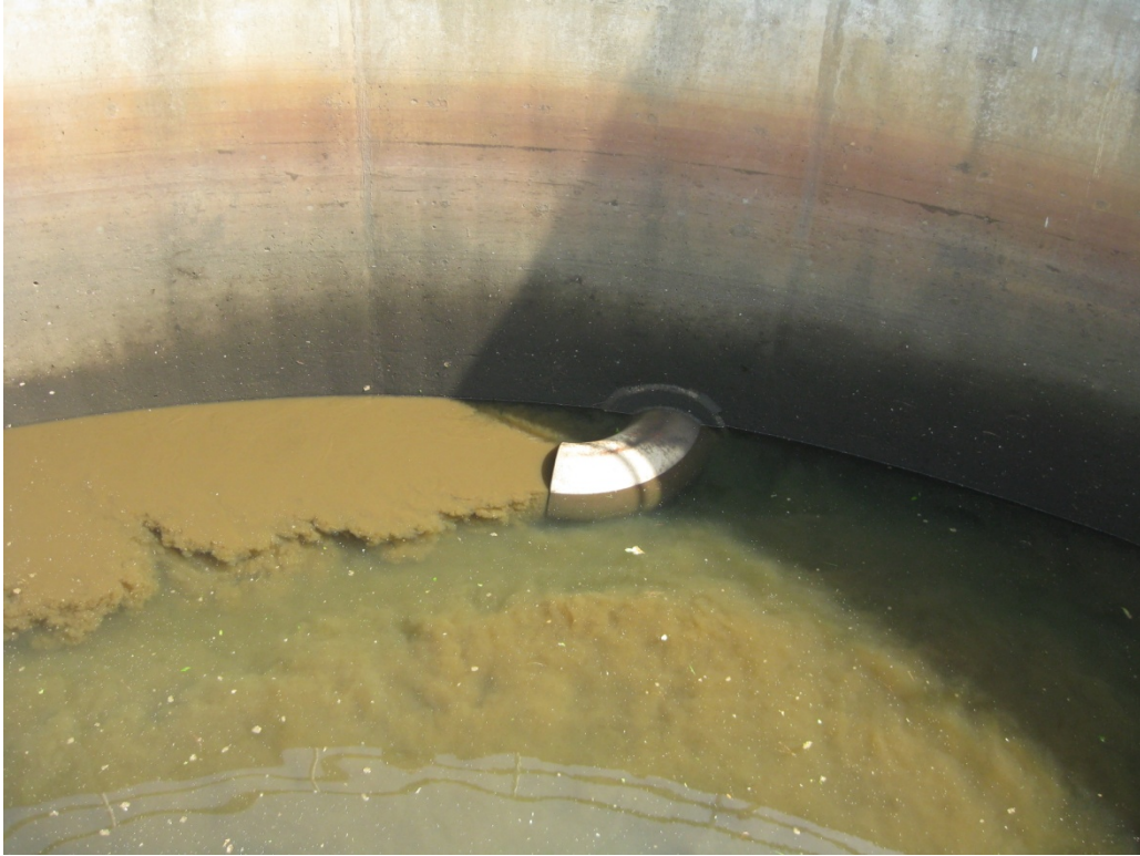
Richmond Road Station – Influent to Washwater Tank
