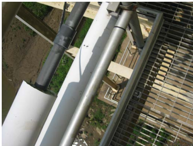
From Raw Water Pump Platform
