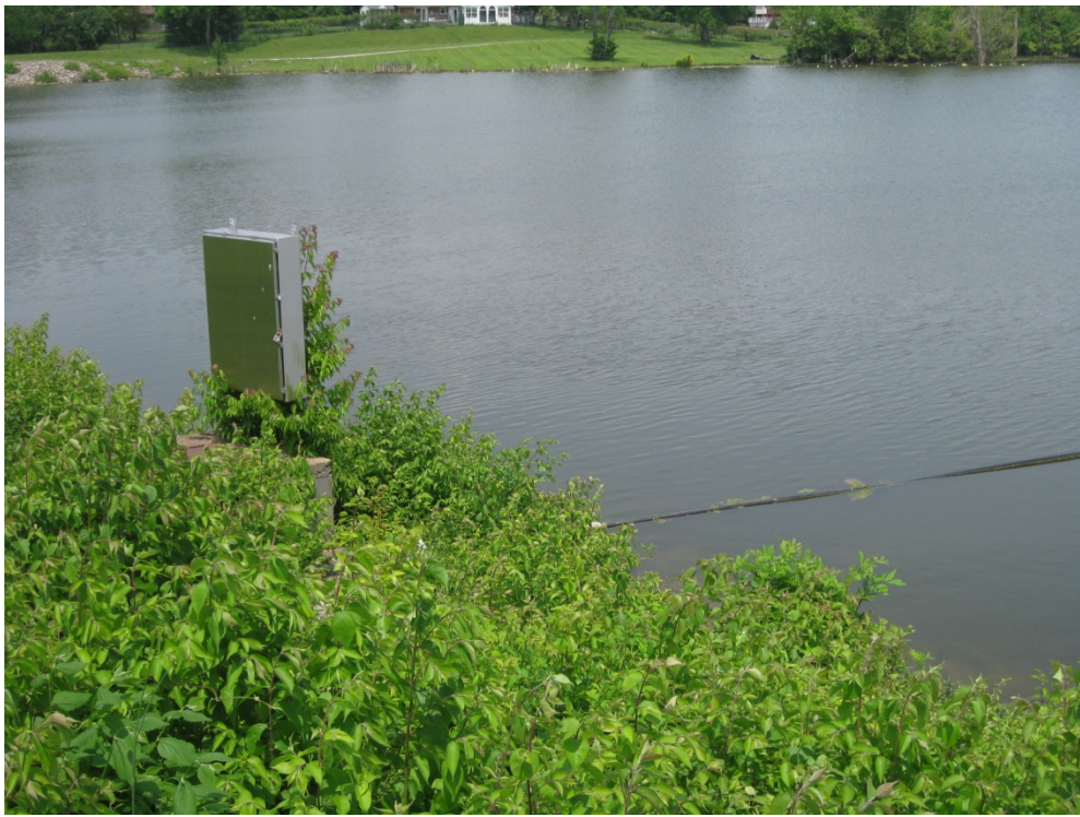
Jacobson Reservoirs – Aeration System
