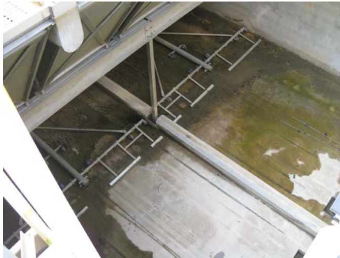
Plate Settler Basin Sludge Rakes
