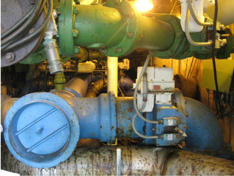
Richmond Road Station – Filter Piping Gallery
