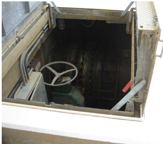
Valve Vault Rapid Mix to Hydrotreator
