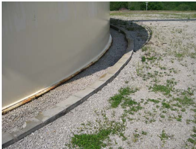
Ring Foundation Hydrotreater
