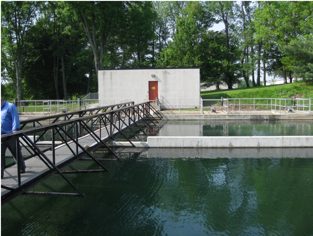
Richmond Road Station – Sedimentation Basins
