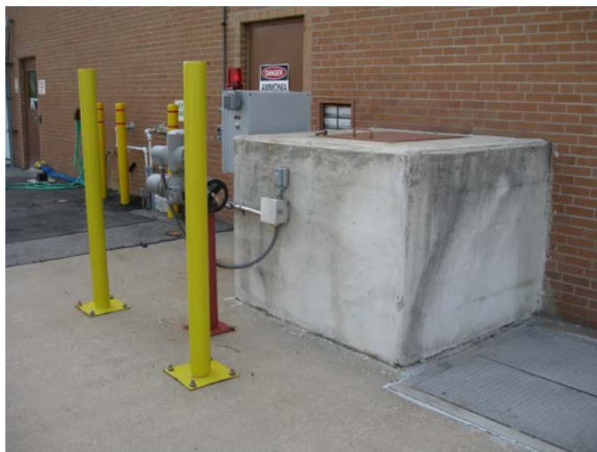
Chlorine Room Vacuum
