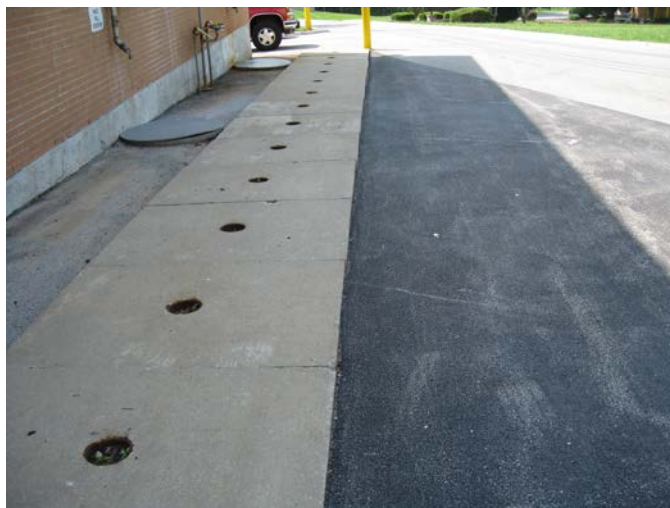
Chemical Feed Trench
