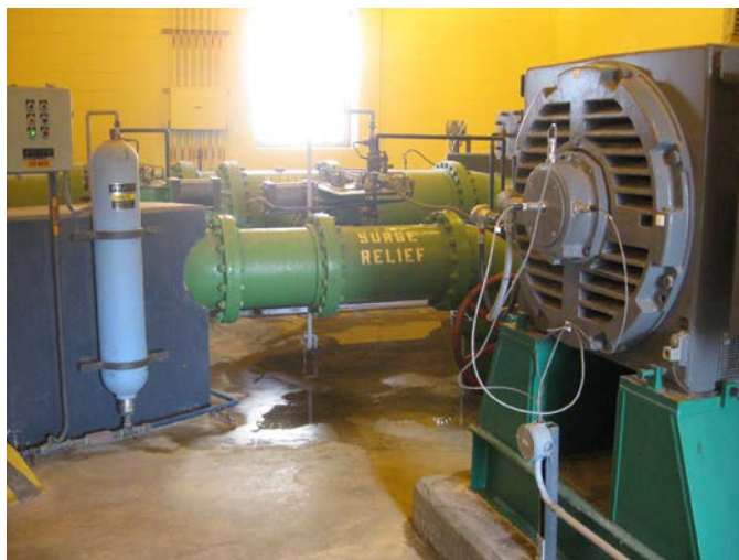
Raw Water Transfer Pumps
