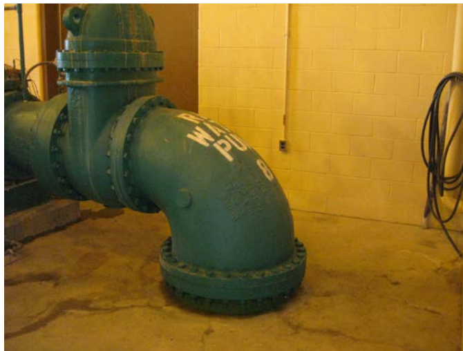
Raw Water Transfer Pumps
