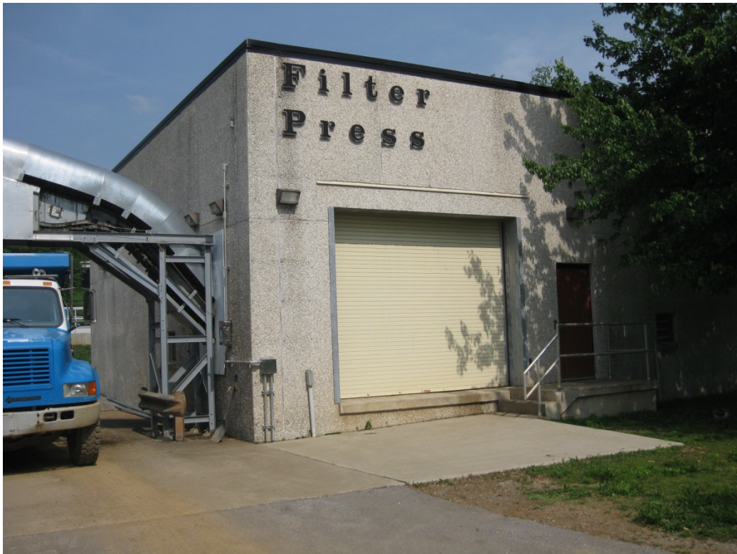
Richmond Road Station – Filter Press Building
