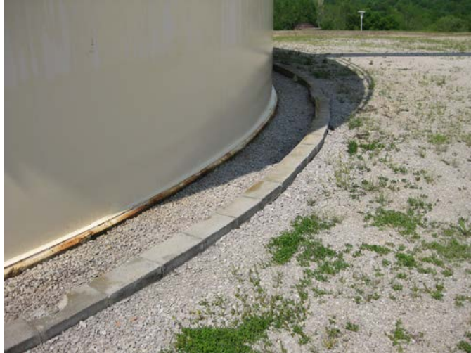
Ring Foundation Hydrotreater
