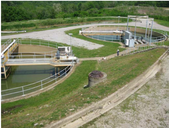
Waste Water Basins & Sludge Lagoons
