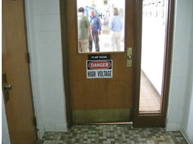
High Service Pumps
