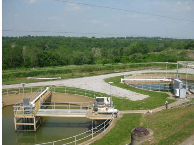
Waste Water Basins & Sludge Lagoons
