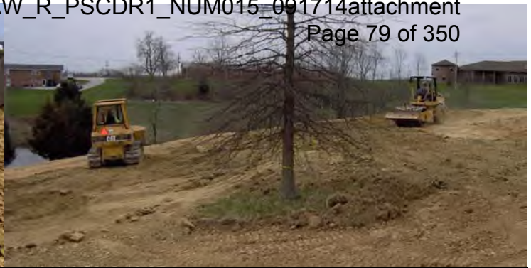
Construction of Two New Water Towers
