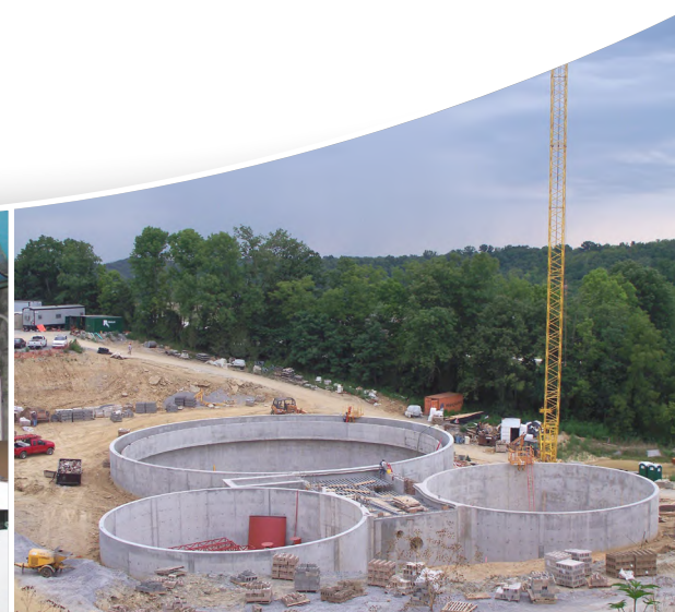
Kentucky River Station II WTP
