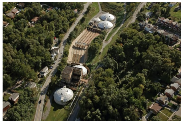
Figure 1: Gannett Fleming conducted a complete evaluation of the existing 60 mgd Hays Mine WTP.
