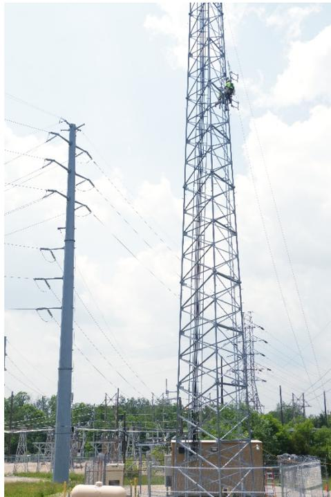
FIGURE 8 - RF MESH COLLECTOR INSTALLATION ON COMMUNICATIONS TOWER
