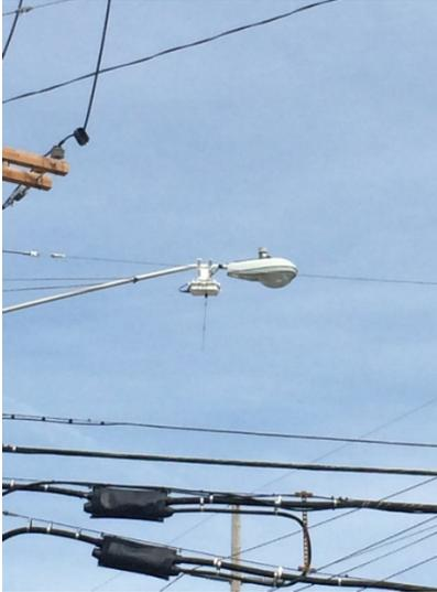
FIGURE 11 - RF MESH ROUTER INSTALLATION ON STREET LIGHT
