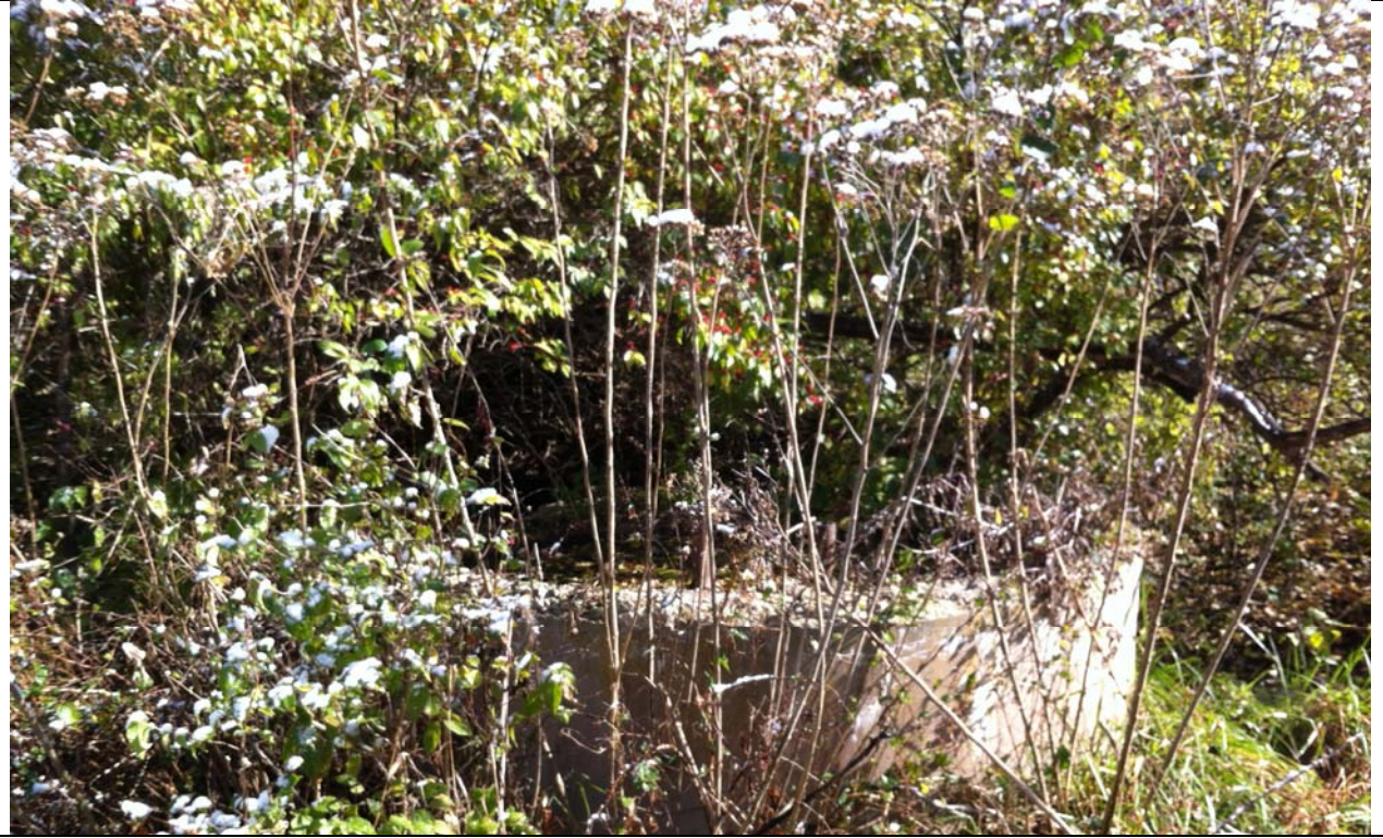
Photograph 17 - concrete spring structure at stream 1 / wetland 3
