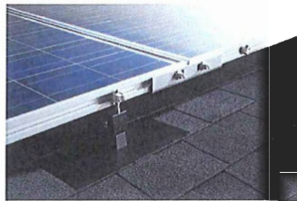
Figure 8. Zep Solar Roof Mount
