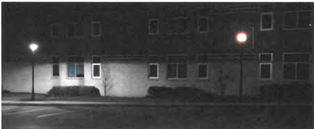
This picture from Madison County shows an LED replacement (left) of a typical exterior metal halide fixture (right). Note the amount of light cast on the building with the LED
