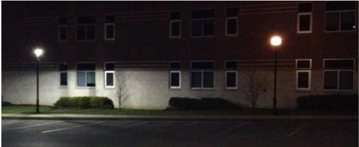
This picture from Madison County shows an LED replacement (left) of a typical exterior metal halide fixture (right). Note the amount of light cast on the building with the LED providing an additional safety benefit.
