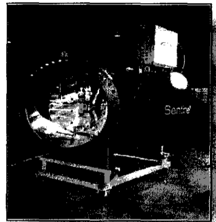
GCWW is implementing a 240-mgd UV treatment facility
