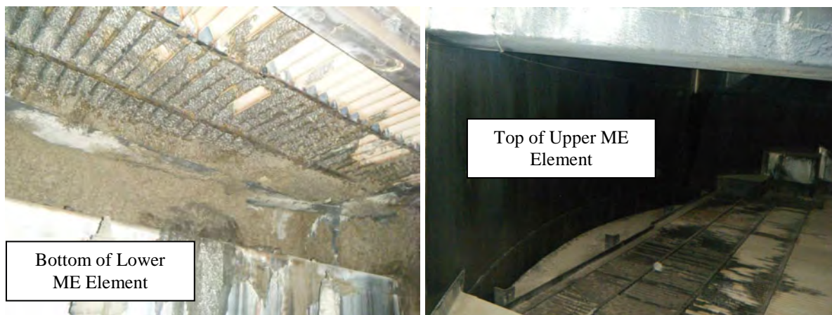
Figure 8. Photos of Existing Unit 4 Mist Eliminator Elements
