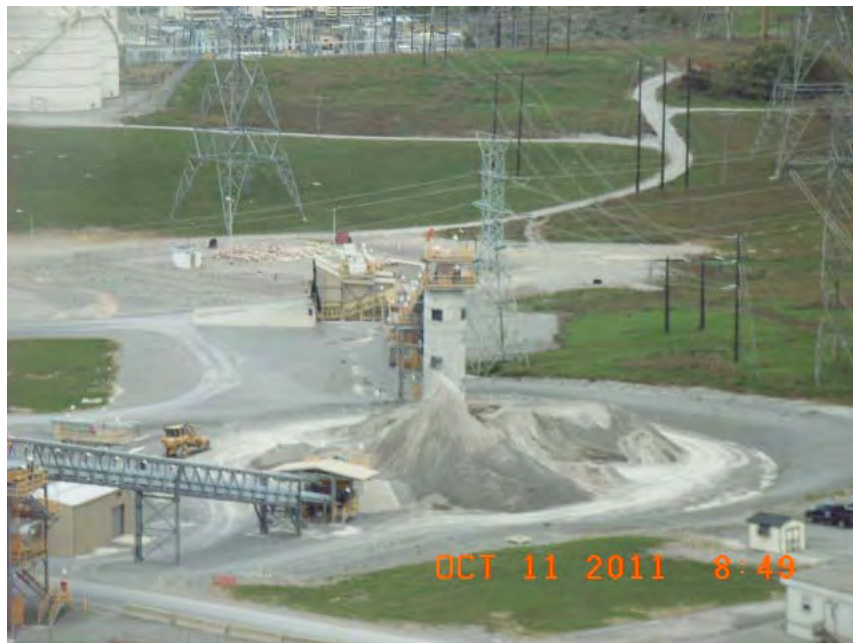
Limestone Loading Facility at Brown Generating Station
