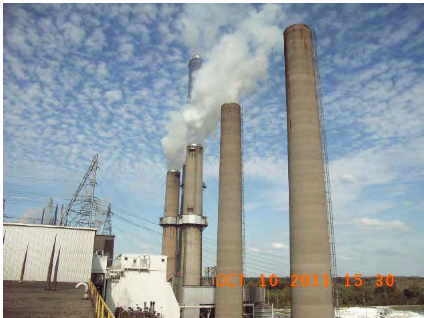
Stacks at Cane Run Generating Station
