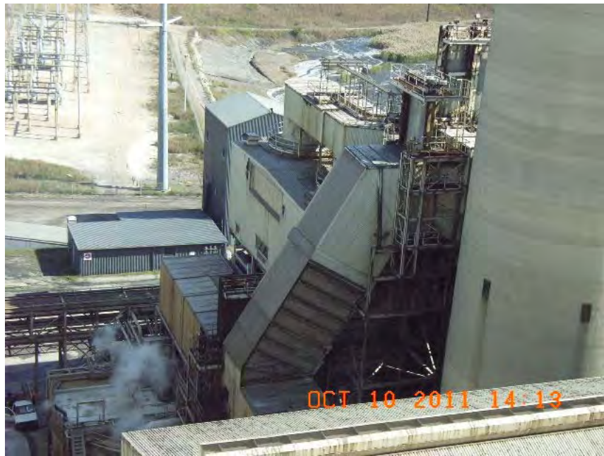
Unit 4 FGD at Mill Creek Generating Station
