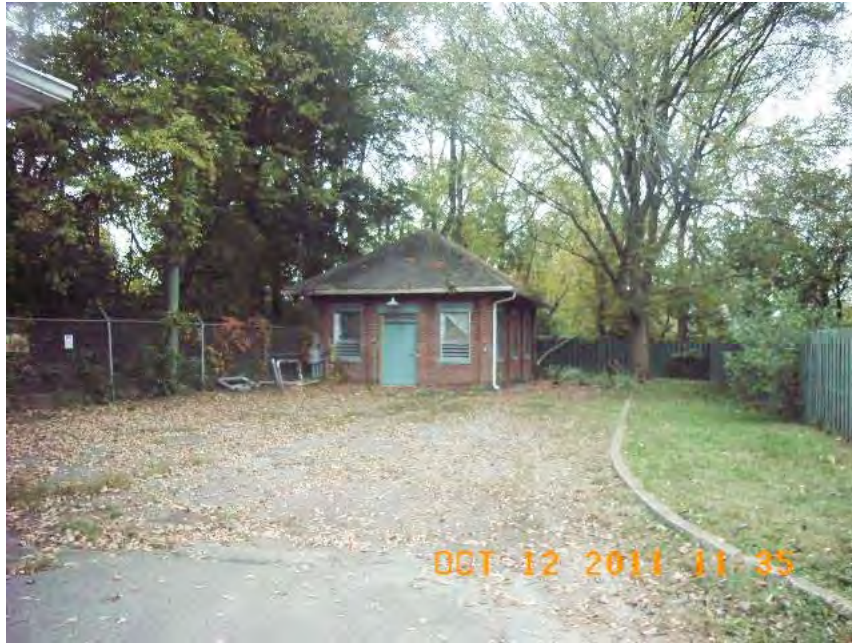
Storeroom/Generator Building at Cannon's Regulating Station
