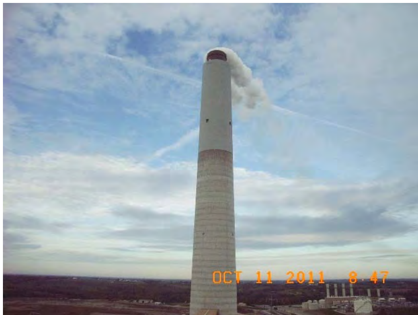
Scrubber Stack at Brown Generating Station
