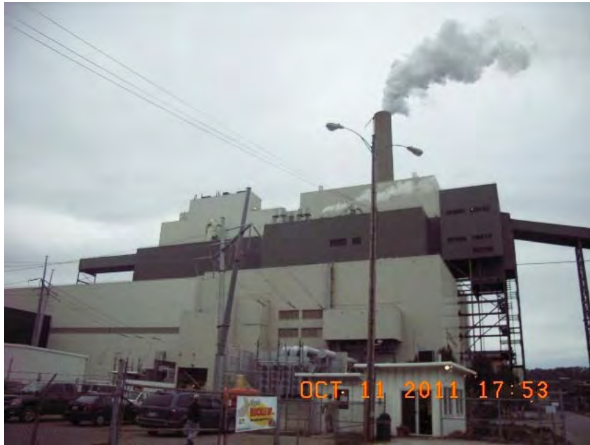
Trimble County Generating Station
