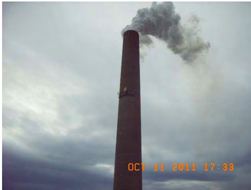
Scrubber Stack at Trimble County Generating Station
