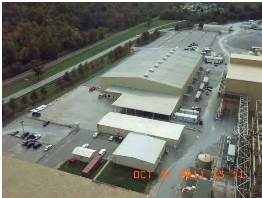
Maintenance Building at Ghent Generating Station
