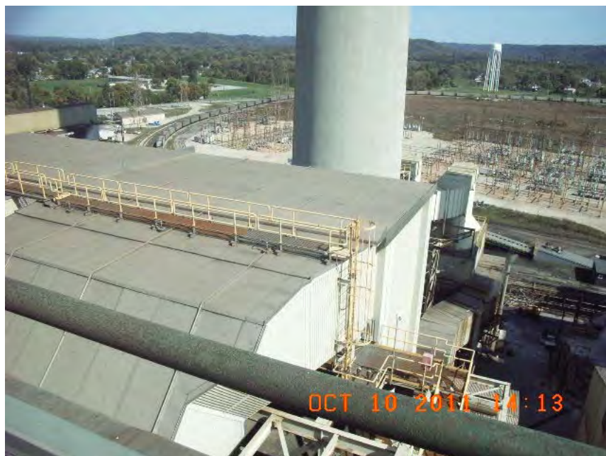
Unit 3 SCR AND FGD at Mill Creek Generating Station
