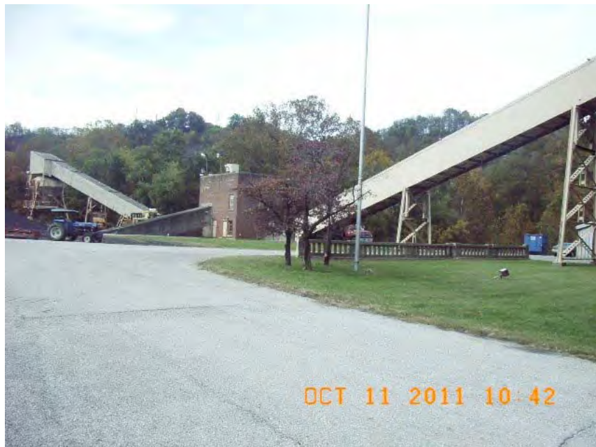
Coal Handling Equipment at Tyrone Generating Station
