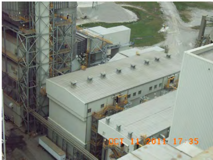
Unit 2 Precipitator and Baghouse at Trimble County Generating Station
