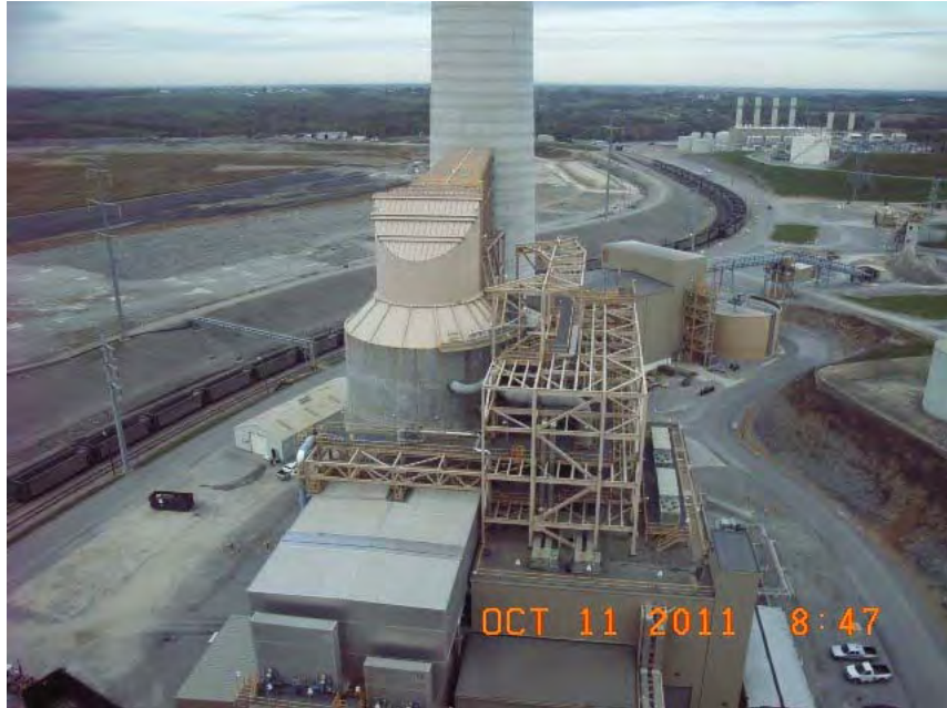
Scrubber at Brown Generating Station
