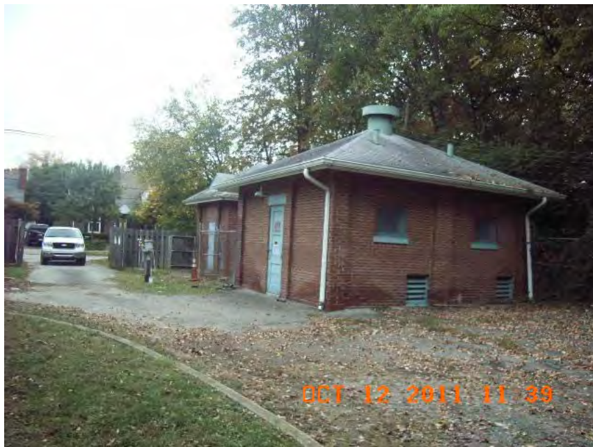
Measurement and RTU Buildings at Cannon's Regulating Station
