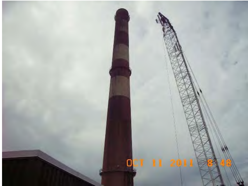
Unit 3 Stack at Brown Generating Station
