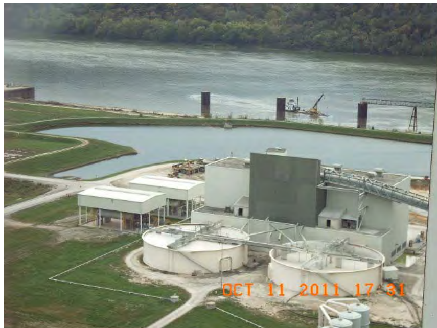
Limestone Facility at Trimble County Generating Station
