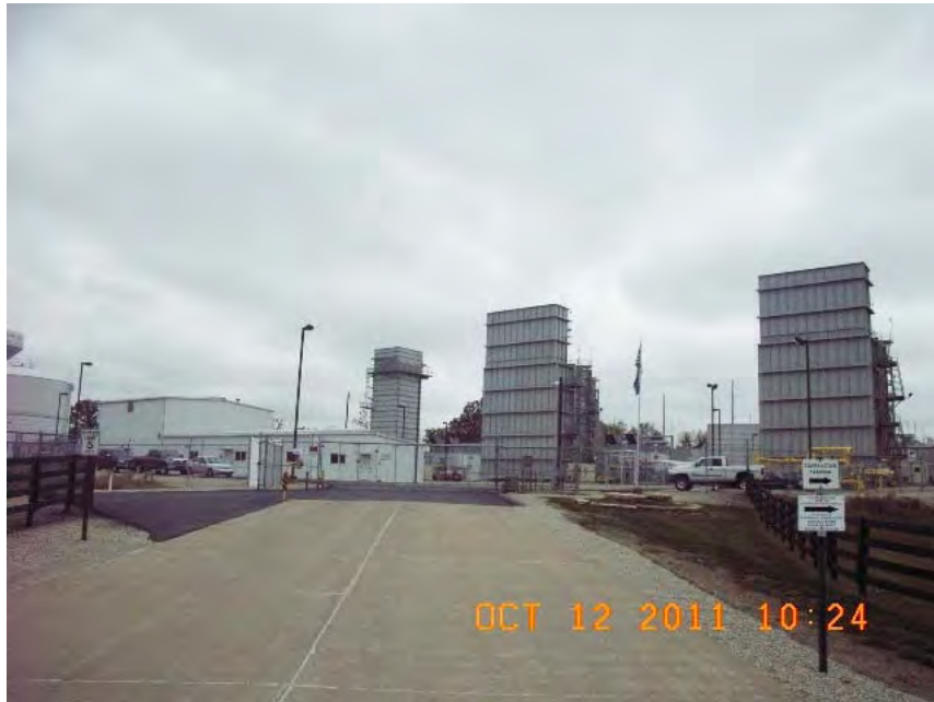
3 Combustion Turbines Soon to be Acquired LS Power (Bluegrass Generation)
