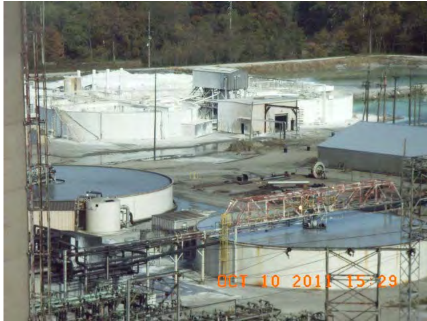
Thickeners and Lime Facility at Cane Run Generating Station
