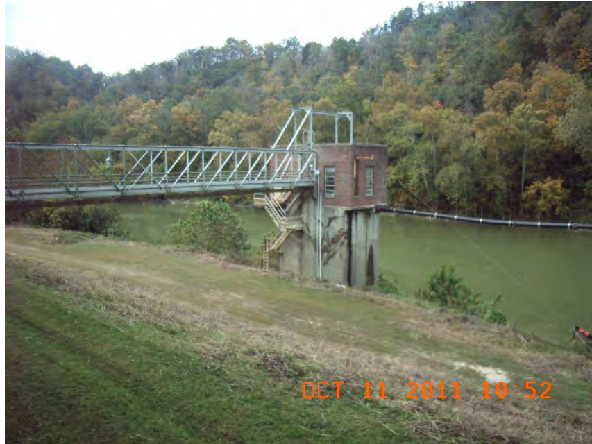
Unit 1 & 2 Intake at Tyrone Generating Station
