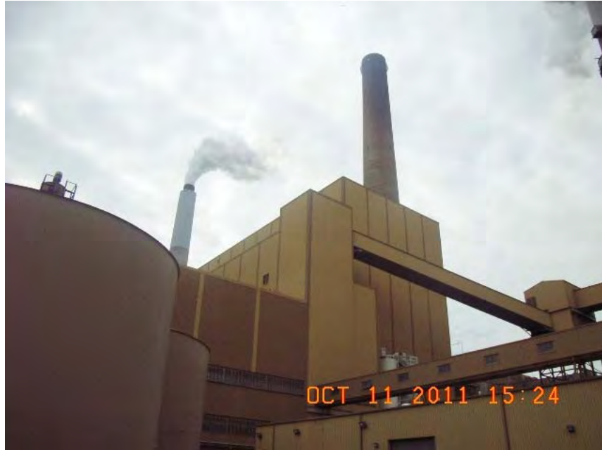
Units 3 & 4 at Ghent Generating Station
