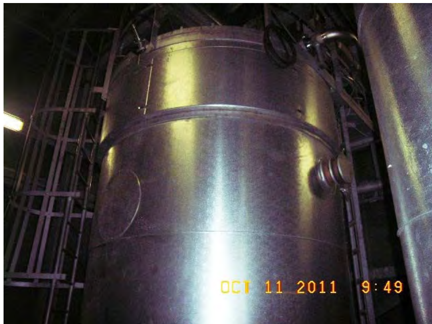
Unit 5 Burner at Brown CT Generating Station
