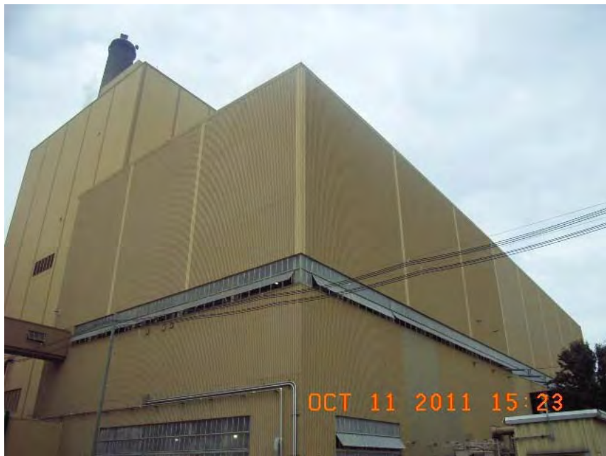
Units 1 & 2 at Ghent Generating Station
