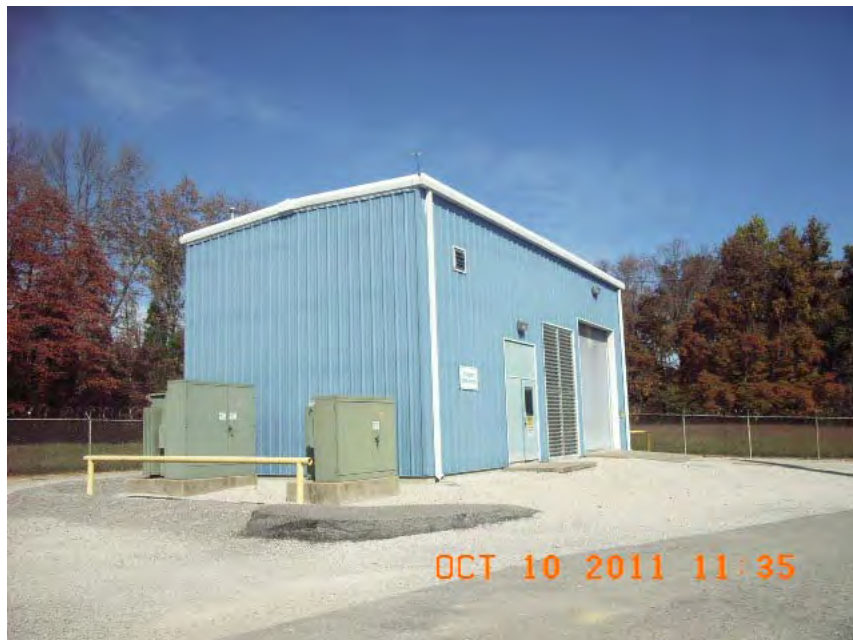
Emergency Generator Building at Muldraugh Compressor Station
