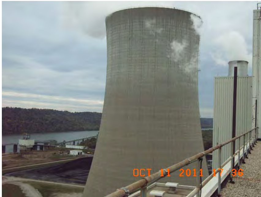
Cooling Tower at Trimble County Generating Station
