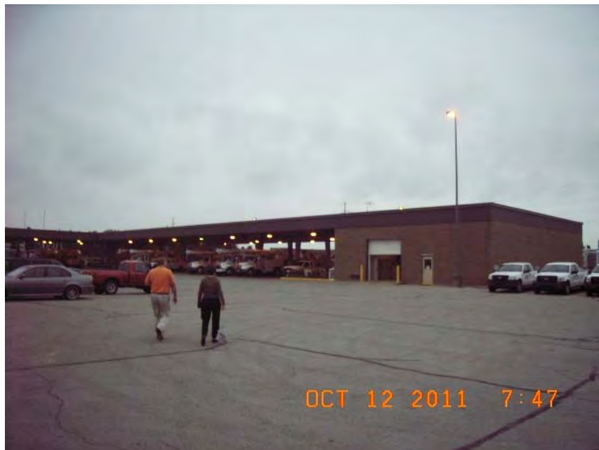
Vehicle Bays at East Service Center
