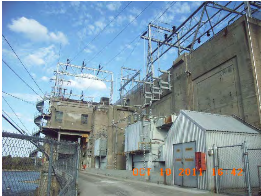
Powerhouse at Ohio Falls Hydro Plant
