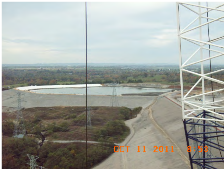
Ash Pond at Brown Generating Station
