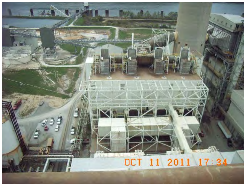
Unit 1 Scrubber at Trimble County Generating Station
