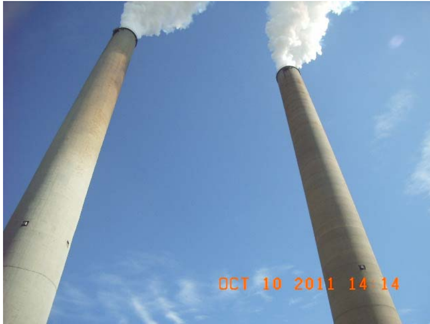
Stacks 3 & 4 at Mill Creek Generating Station
