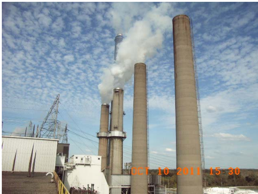
Stacks at Cane Run Generating Station
