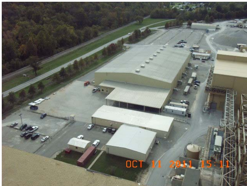
Maintenance Building at Ghent Generating Station
