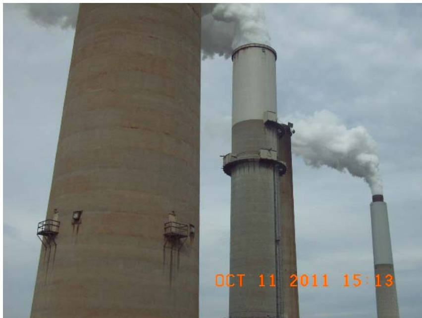
Stacks at Ghent Generating Station
