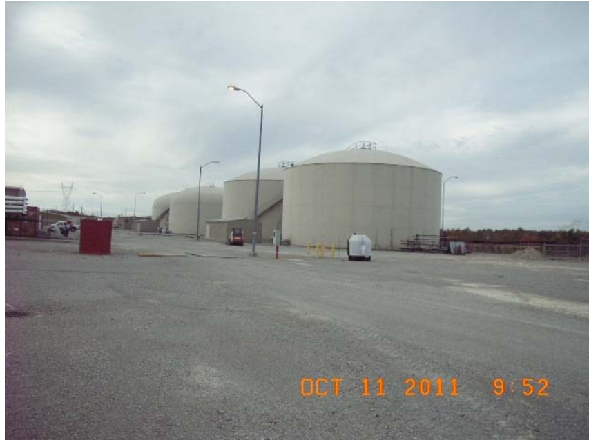
Low NOx Water Tanks at Brown CT Generating Station
