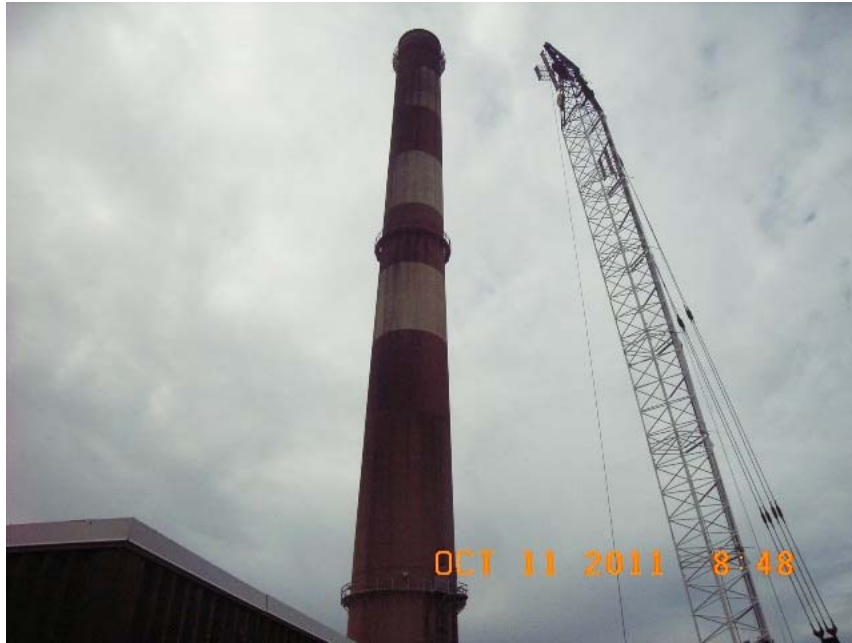
Unit 3 Stack at Brown Generating Station
