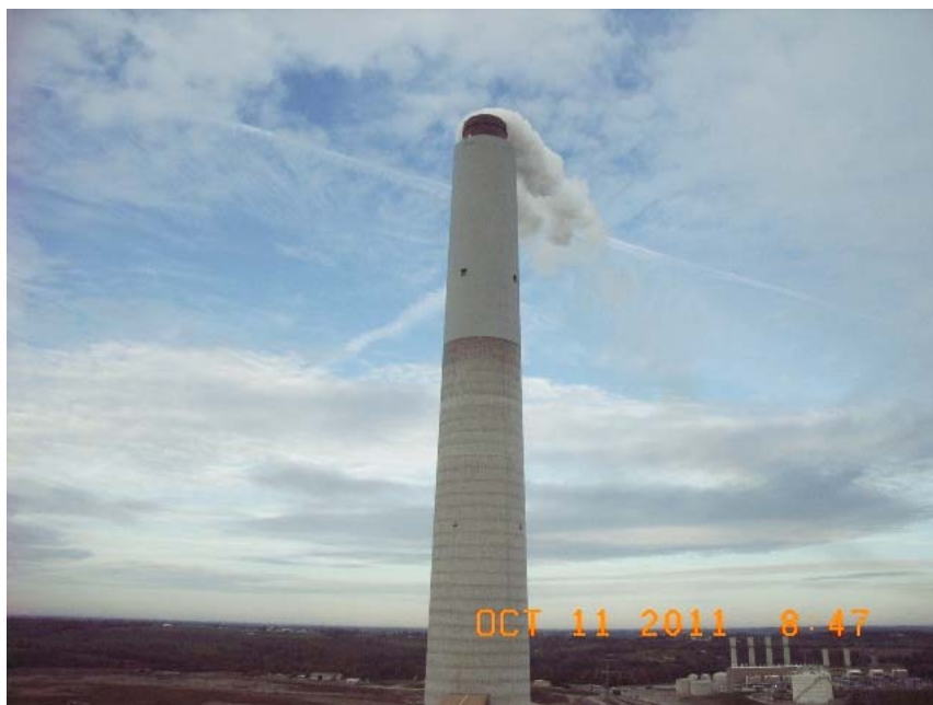
Scrubber Stack at Brown Generating Station
