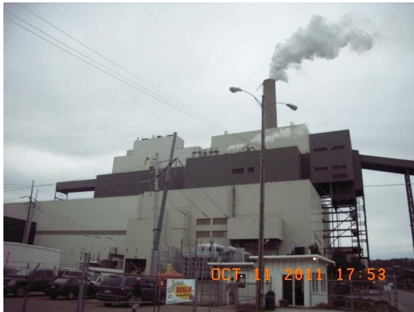
Trimble County Generating Station
