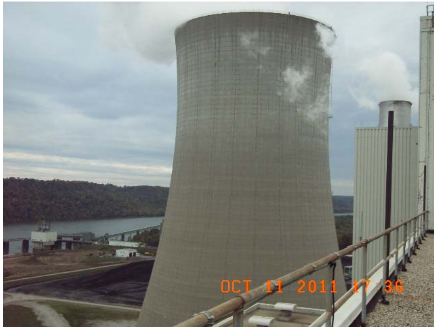
Cooling Tower at Trimble County Generating Station
