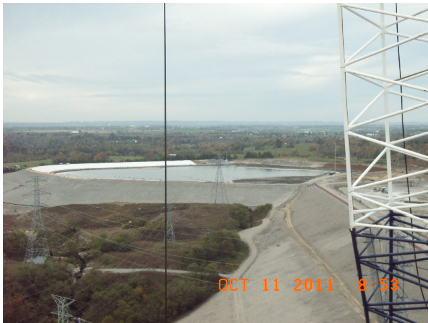
Ash Pond at Brown Generating Station
