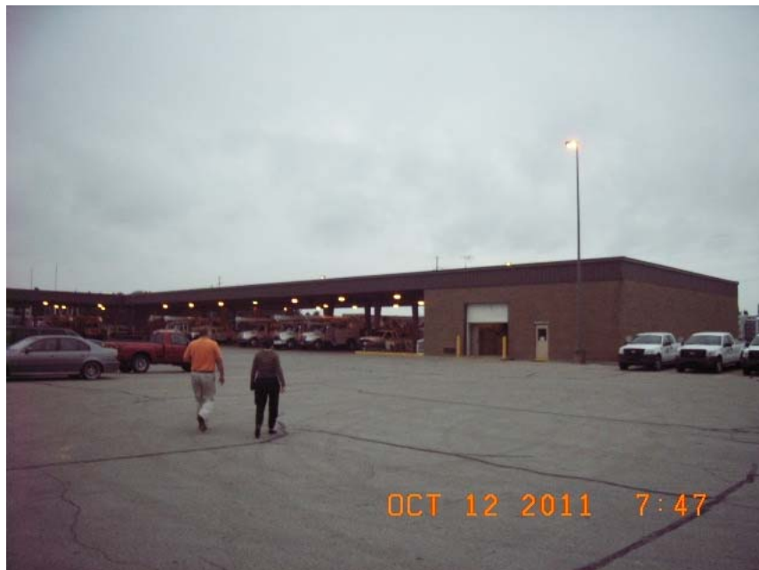
Vehicle Bays at East Service Center
