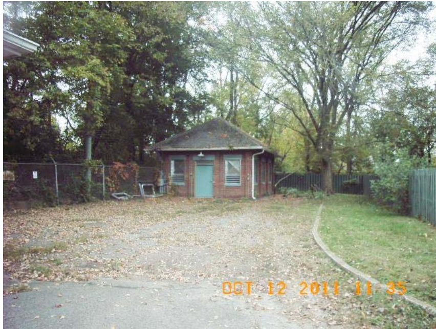
Storeroom/Generator Building at Cannon's Regulating Station
