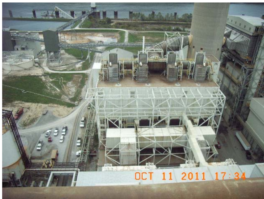
Unit 1 Scrubber at Trimble County Generating Station
