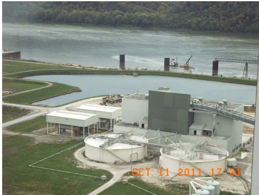
Limestone Facility at Trimble County Generating Station
