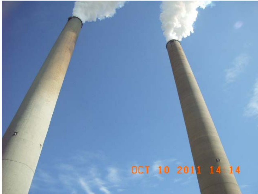
Stacks 3 & 4 at Mill Creek Generating Station
