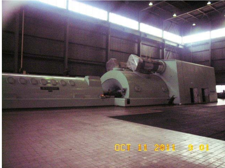
Unit 3 Turbine at Brown Generating Station
