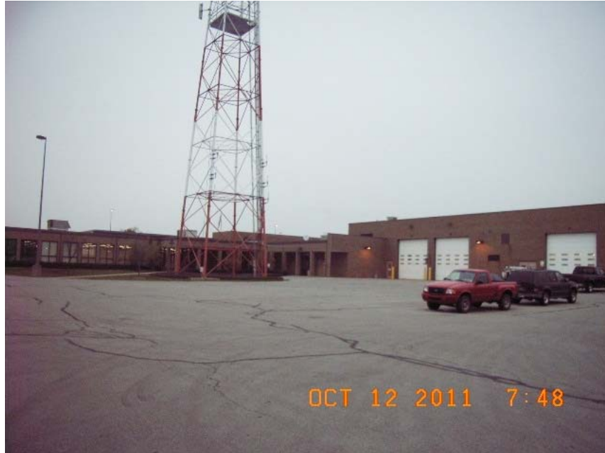
Rear of Building and Tower at East Service Center
