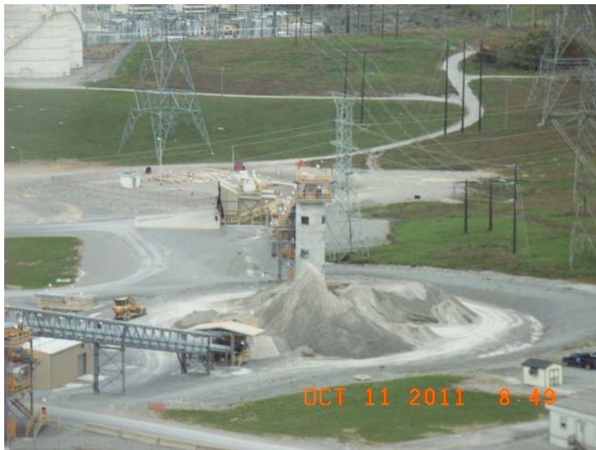
Limestone Loading Facility at Brown Generating Station
