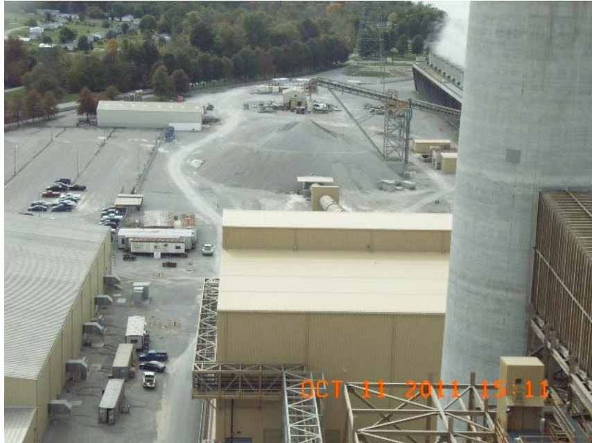
Limestone Building and Loading at Ghent Generating Station
