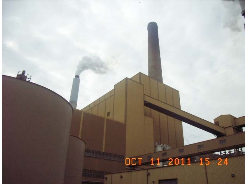
Units 3 & 4 at Ghent Generating Station
