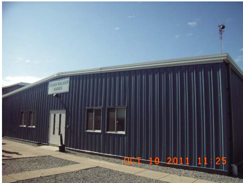
Newly Built Office Building at Muldraugh Compressor Station
