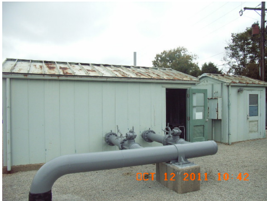
Measurement Buildings at Elder Park City Gate Station
