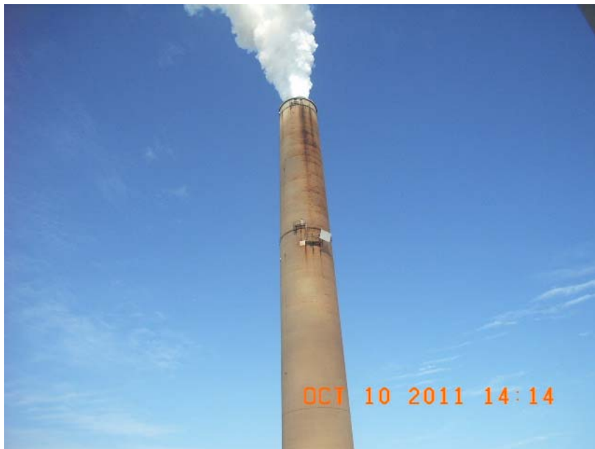
Stack for Units 1 & 2 at Mill Creek Generating Station
