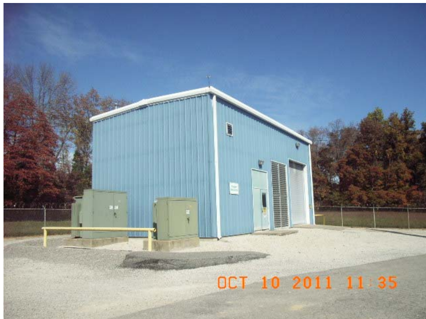
Emergency Generator Building at Muldraugh Compressor Station
