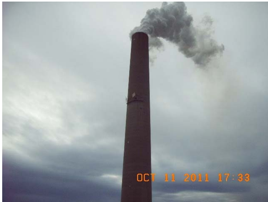
Scrubber Stack at Trimble County Generating Station
