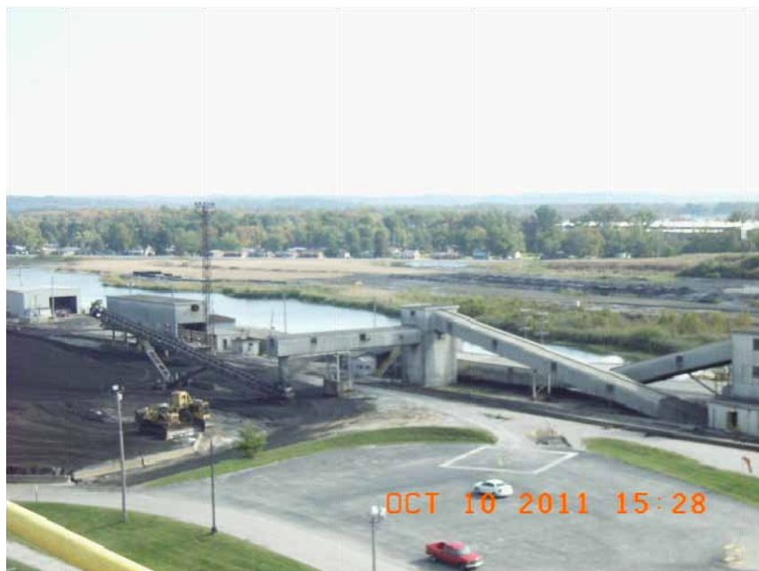
Coal Handling Equipment at Cane Run Generating Station
