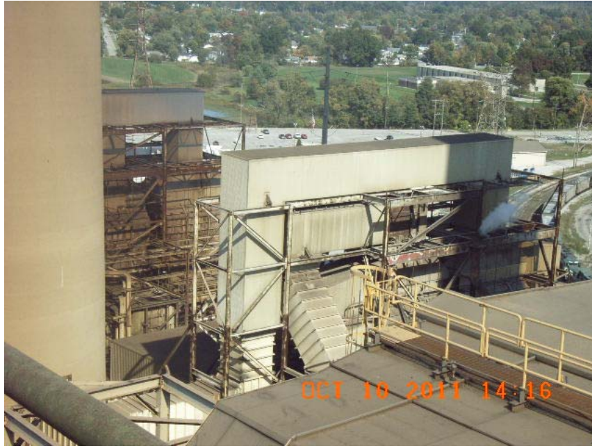
1 & 2 Scrubber at Mill Creek Generating Station
