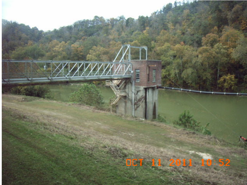
Unit 1 & 2 Intake at Tyrone Generating Station
