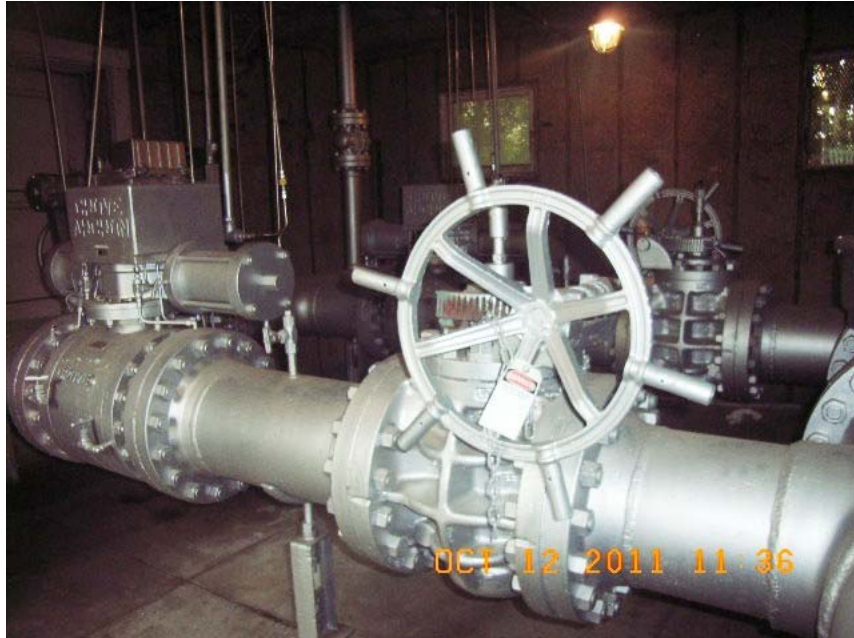
Regulator Runs at Cannon's Regulating Station
