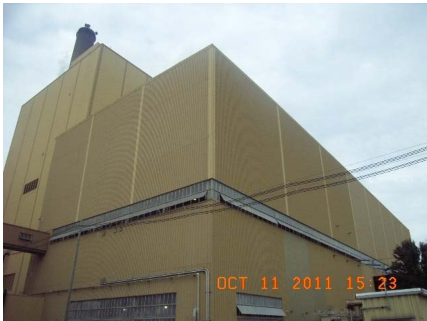
Units 1 & 2 at Ghent Generating Station
