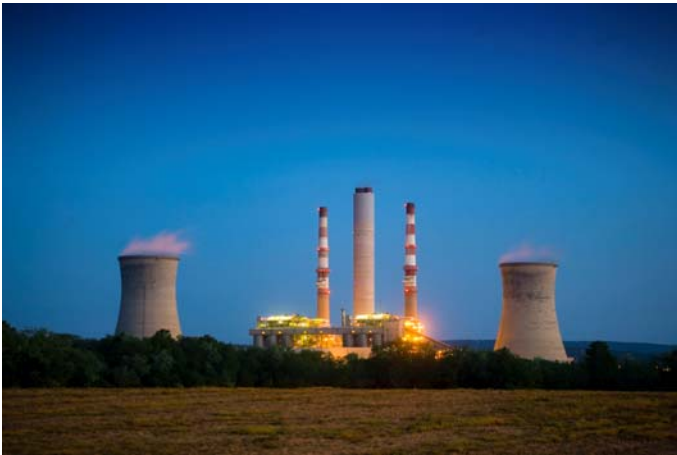
Scrubbers at Montour
