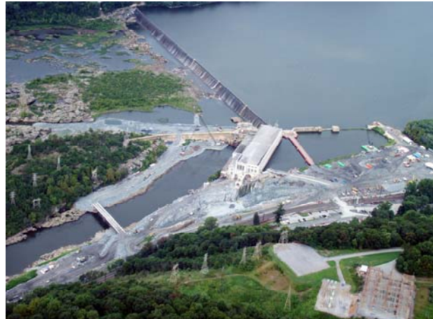
Holtwood Hydro Expansion Project
