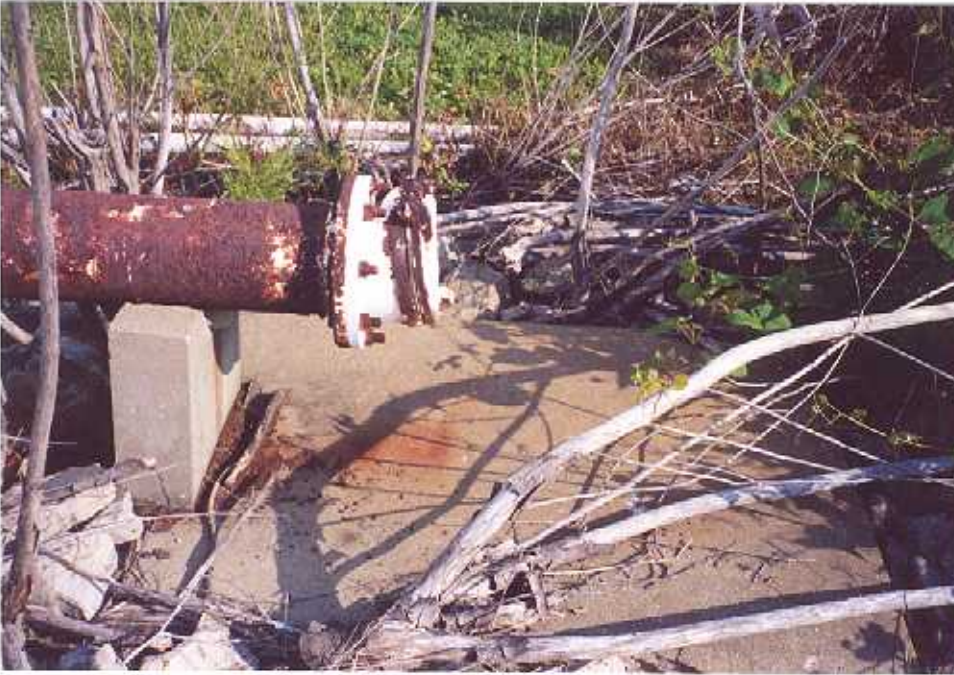
11. Flap gate on overflow discharge above concrete splash pad. Note dead vegetation surrounding concrete splash pad.
