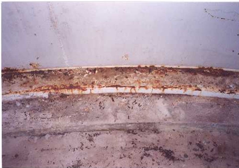
32. Corrosion on the interior base plate projection.
