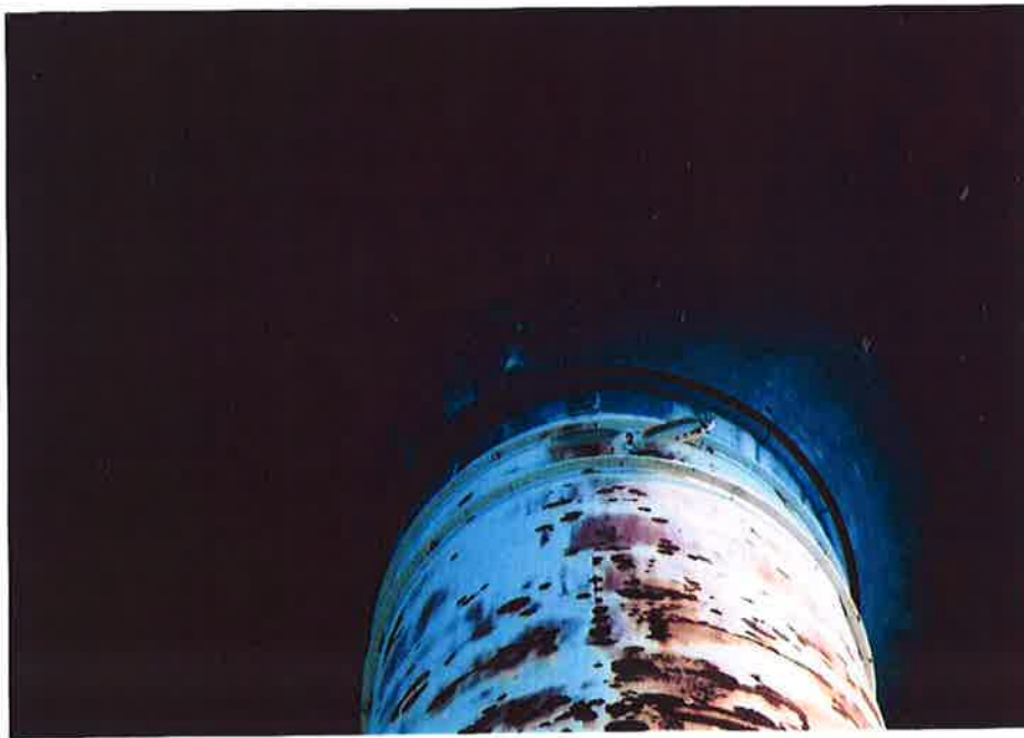
14. Spots of corrosion on support column. Note painter's rings and painter's manhole.
