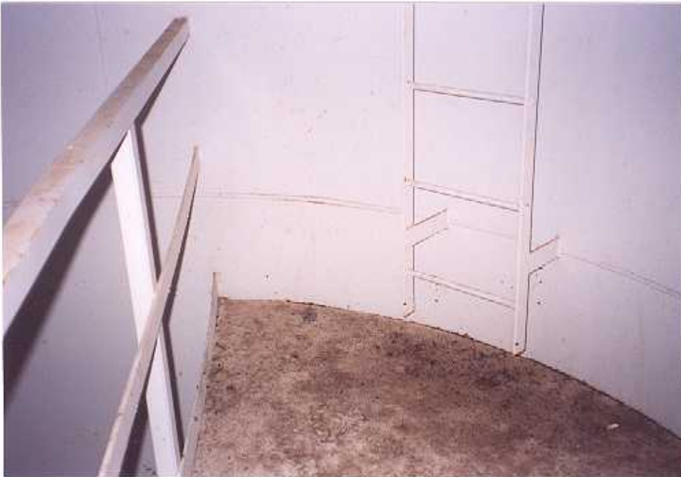
44. Platform and support column ladder section.
