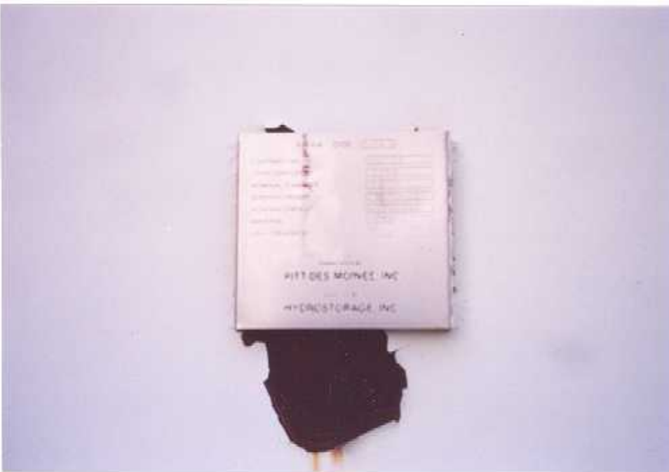
12. Corrosion behind the tank nameplate.
