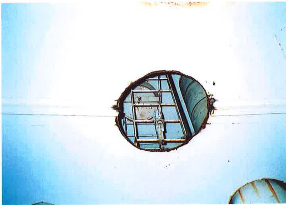
54. Hole cut in stiffening angle.
