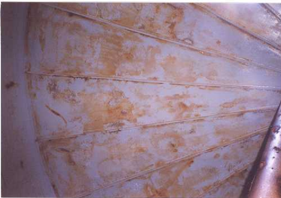
60. Corrosion on the roof.
