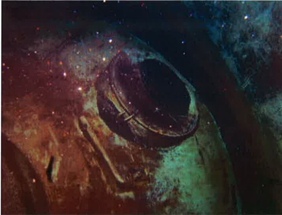
81. Manhole and cover in bowl.
