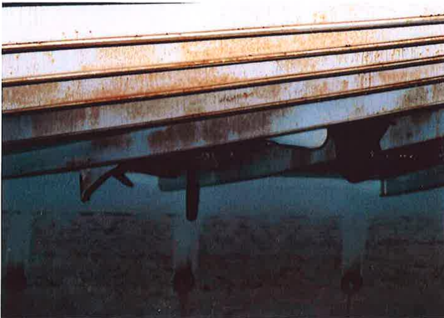
70. Roof support structure and coating failure on shell.
