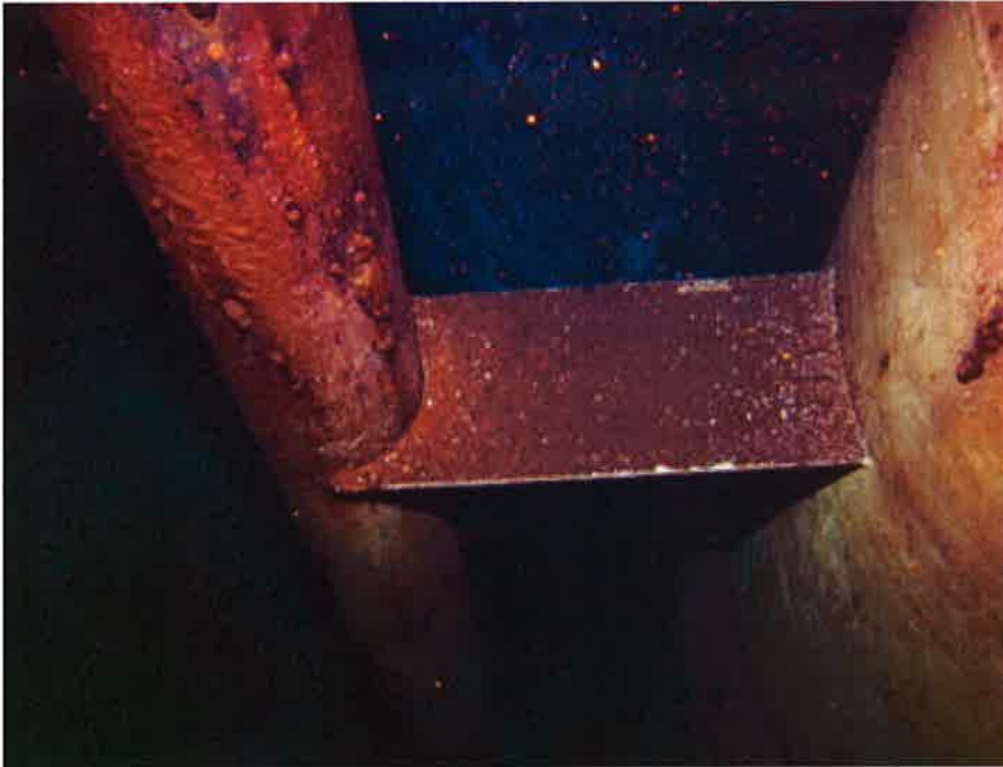
71. Overflow bracket attachment to access tube on tank interior.
