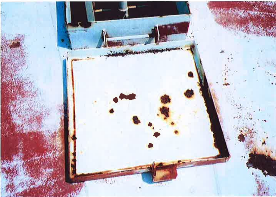
22. Corrosion on roof manhole cover.
