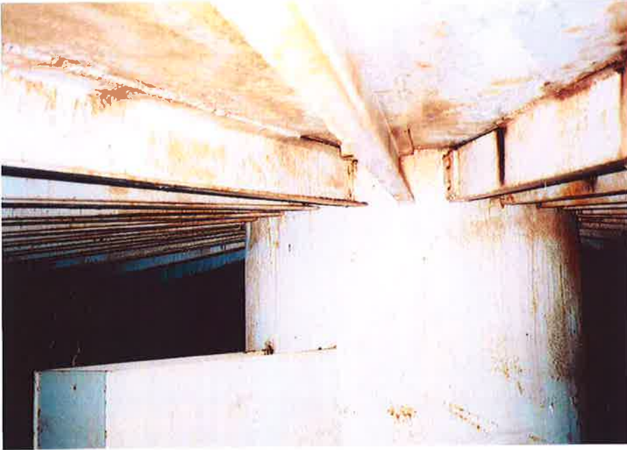
67. Roof support structure connection to access tube.
