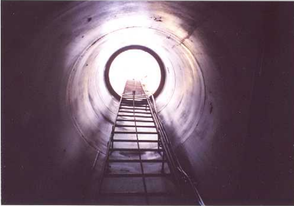
51. Access tube ladder and safe-climbing device. Note conduits.
