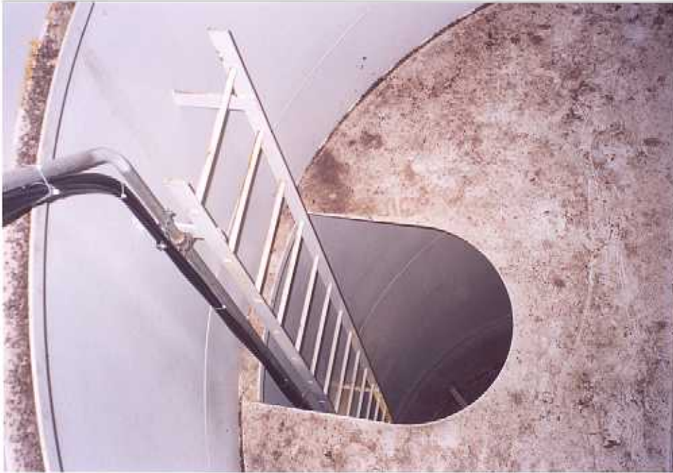
45. Access through a platform and support column ladder section. Note conduit and cables.
