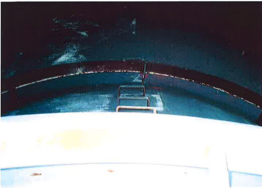
16. Access rungs to painter's rings.
