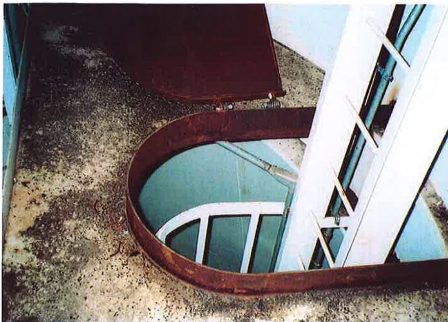
38. Base cone ladder access through bottom platform. Note new, unpainted curb and manhole cover.
