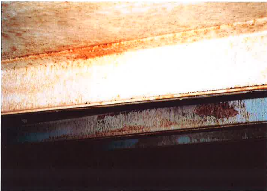
64. Corrosion on the roof support structure.
