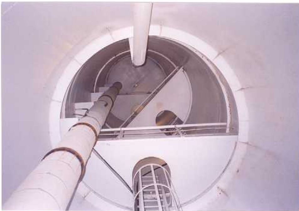
38. Inlet/outlet pipe, dry platforms, and overflow pipe.
