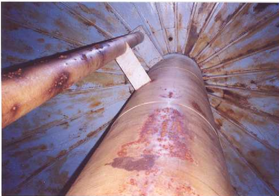
56. Corrosion on the roof, access tube, and overflow pipe.
