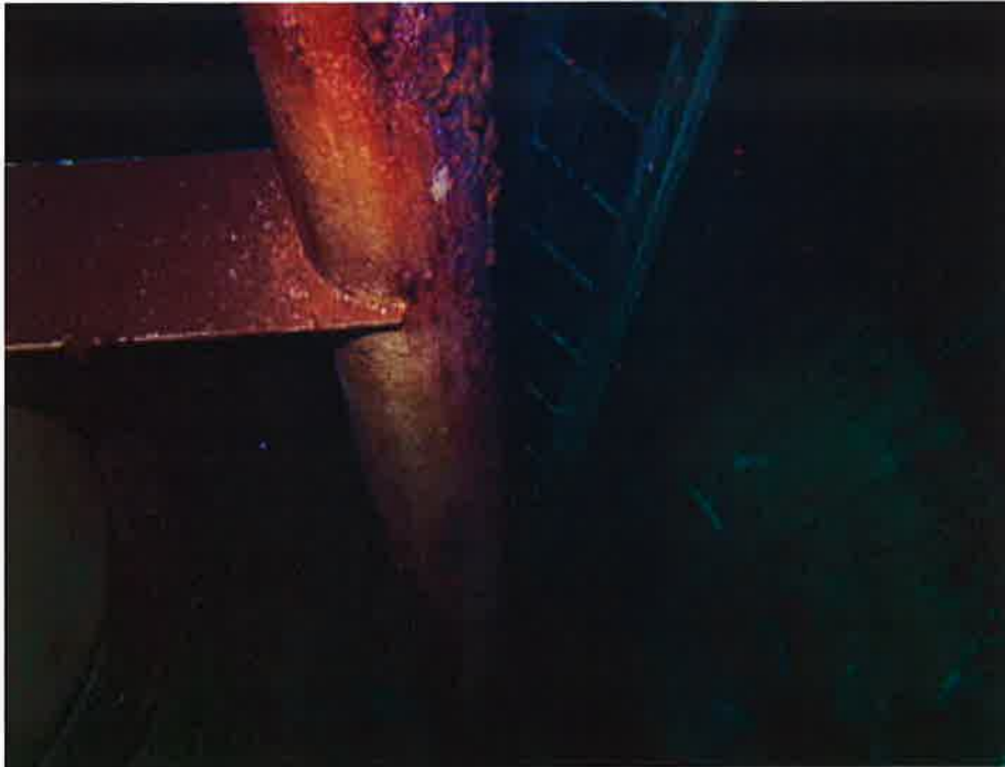
73. Container ladder and overflow pipe and bracket.
