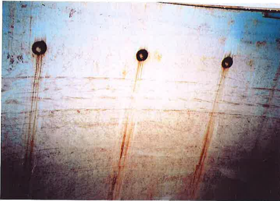
65. Coating failure and rust staining on tank interior.
