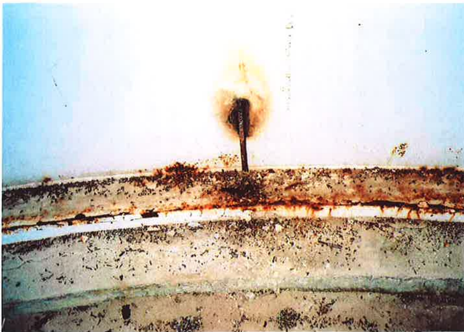
30. Corrosion on the interior base plate projection.
