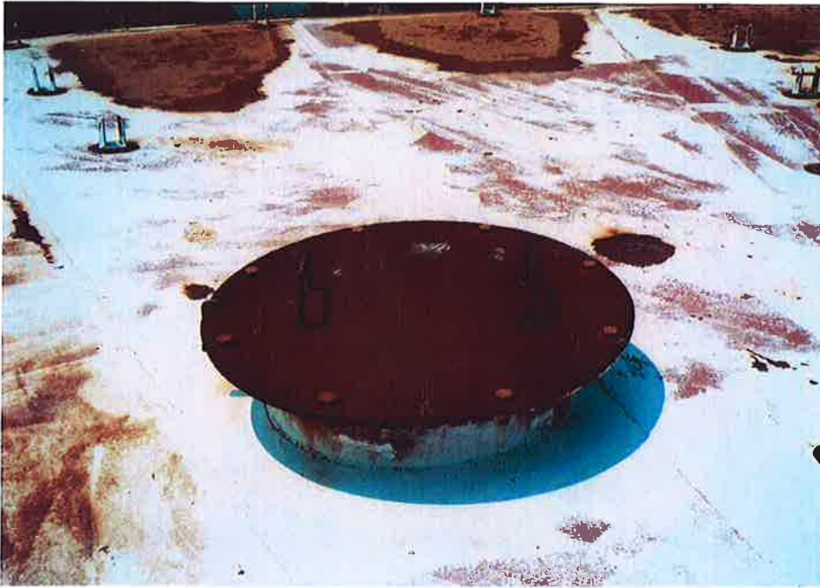
27. Flanged and bolted roof manhole.
