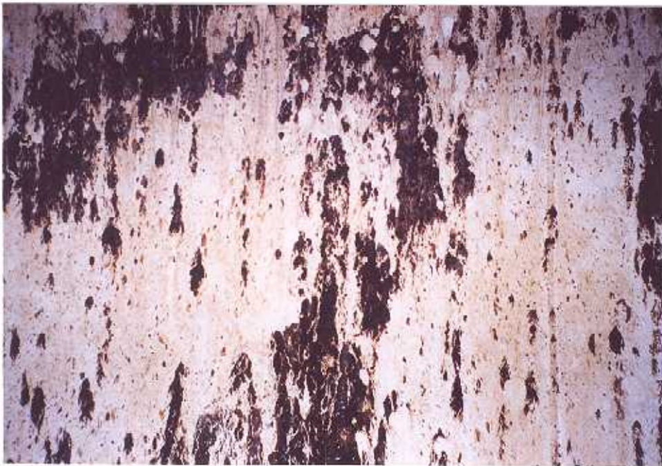
72. Corrosion on the bowl.
