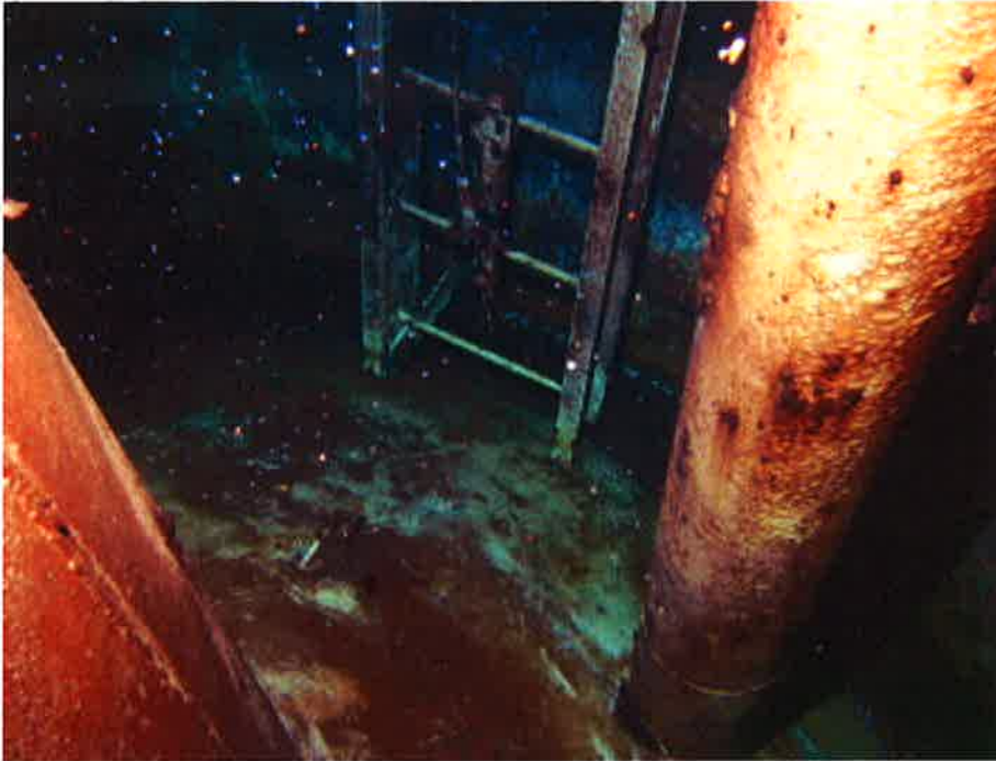
75. Container ladder base and pipe penetration in bowl of tank.
