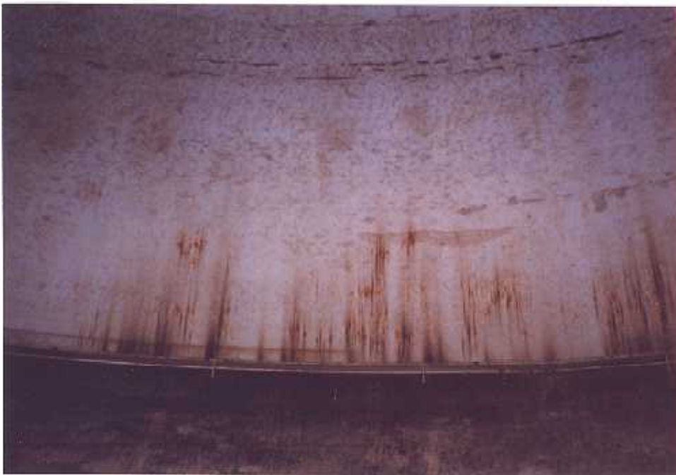
68. Corrosion near the base of the shell.
