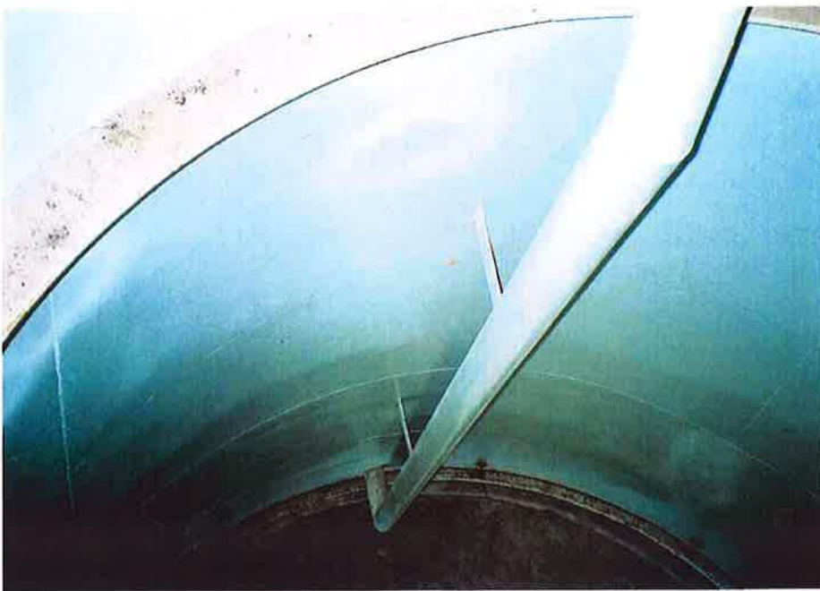
36. Overflow pipe and brackets.
