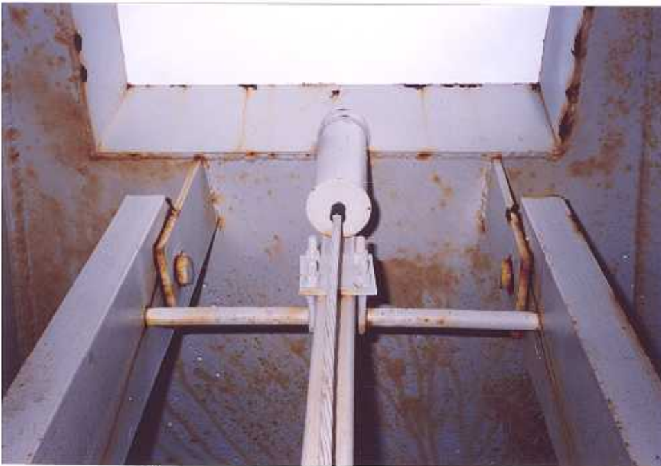
62. Container ladder and safe-climbing device.
