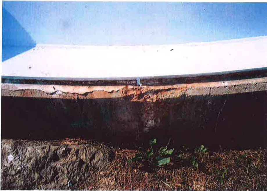
9. Tank foundation, grout, and base plate. Note deteriorated concrete and vegetation near foundation.
