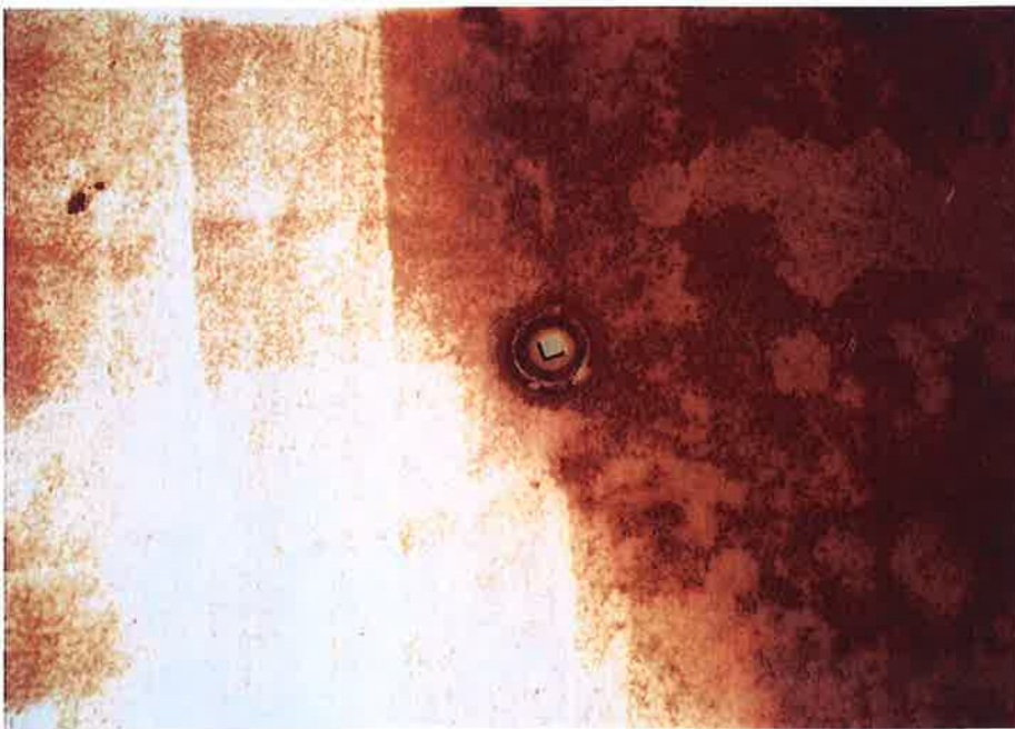
20. Corrosion, topcoat failure, and plugged coupling on the roof.
