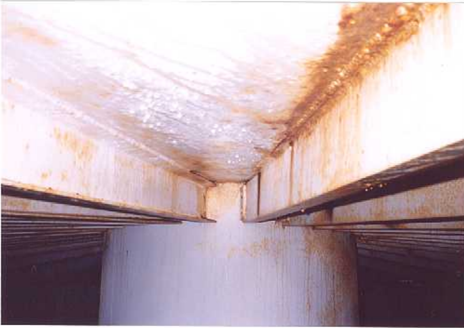
57. Corrosion on the roof.
