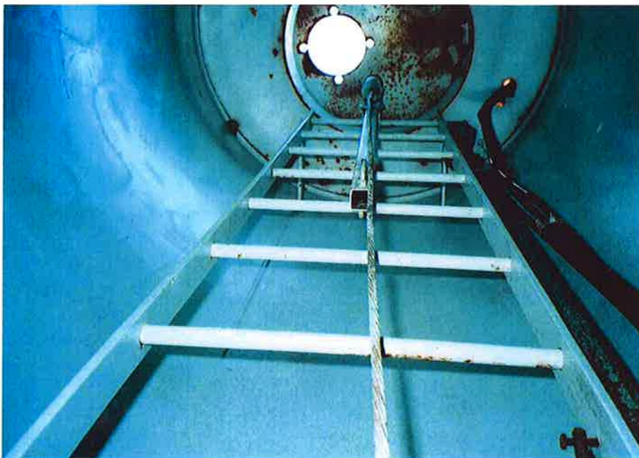
58. Support column ladder, safe-climbing device and platform. Note cables.
