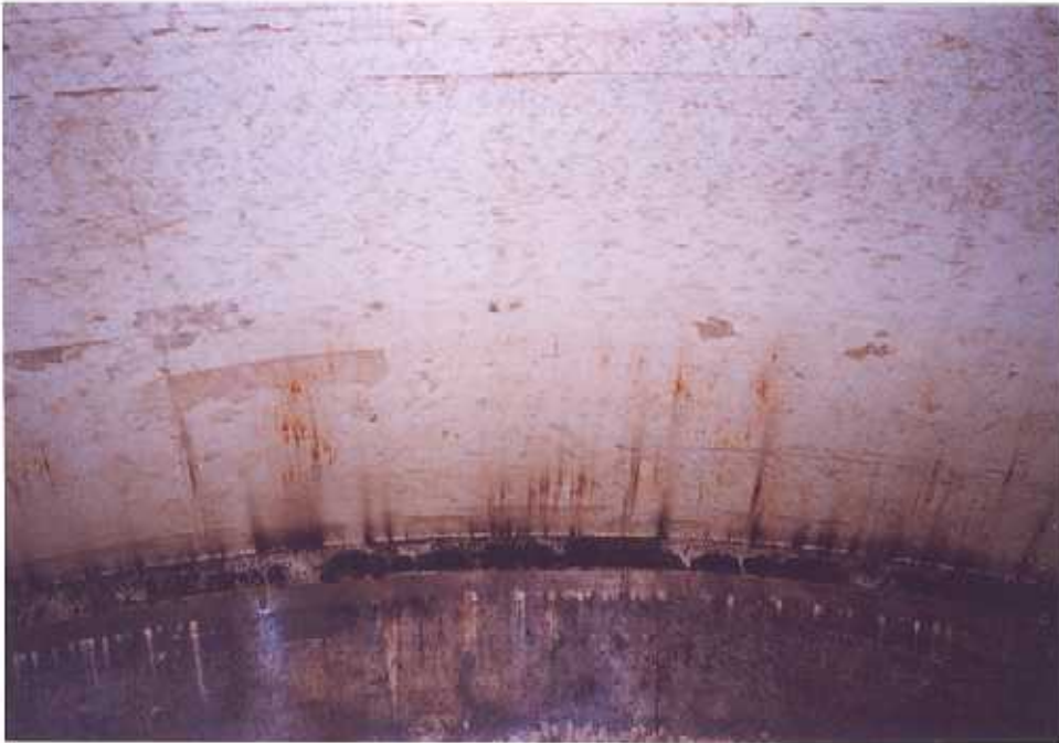
69. Corrosion near the base of the shell.
