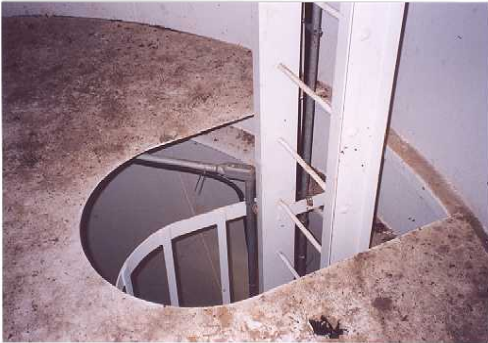
41. Base cone ladder access through bottom platform.
