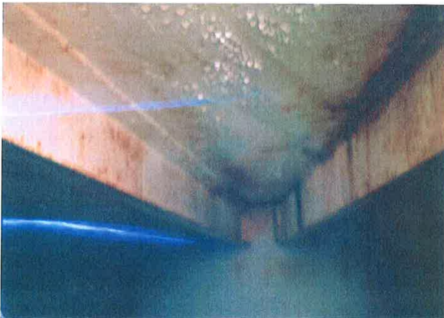
62. Roof support structure.
