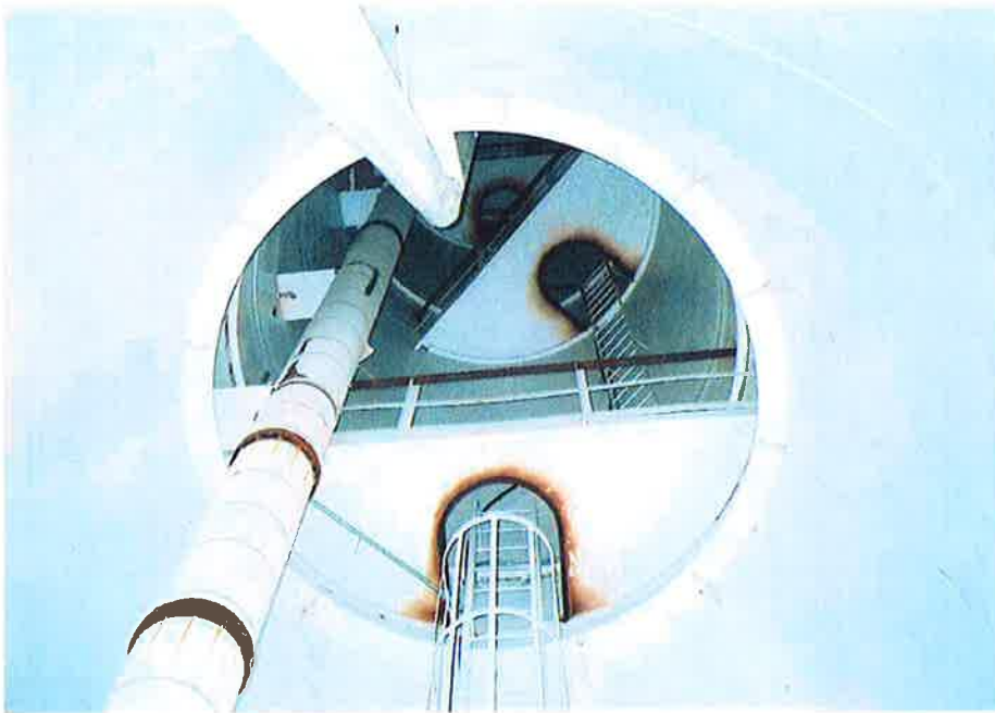
34. Inlet/outlet pipe, dry platforms, and overflow pipe.
