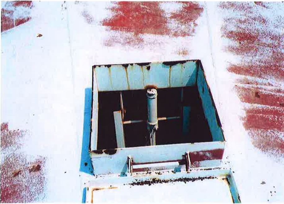
23. Roof manhole and interior container ladder.
