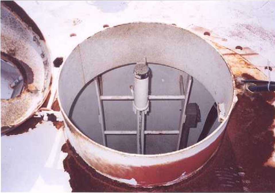
55. Top of the access tube ladder and safe-climbing device.
