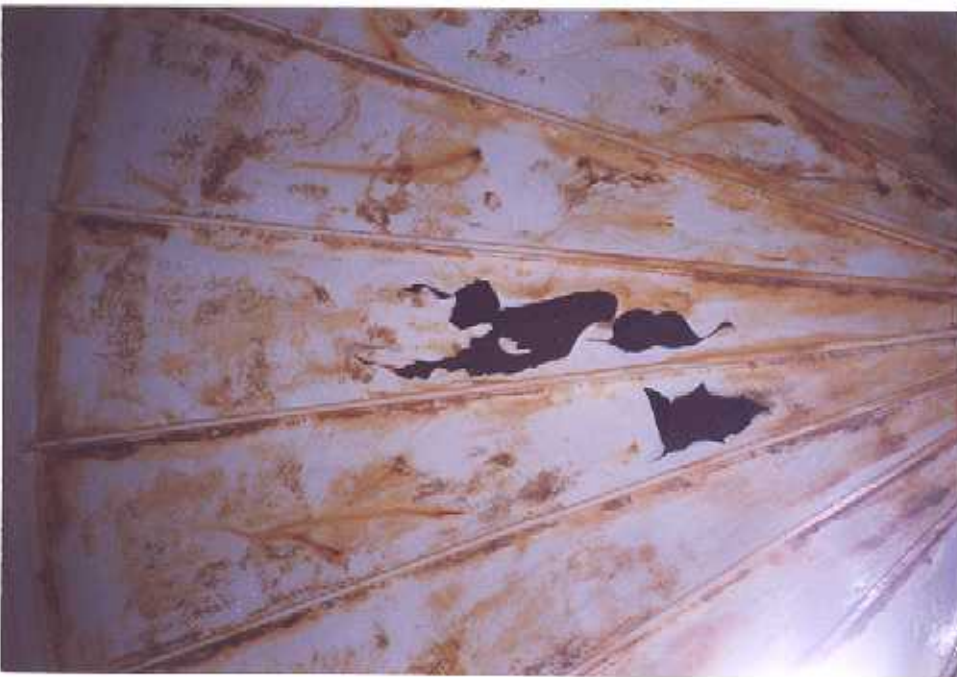
58. Corrosion on the roof.
