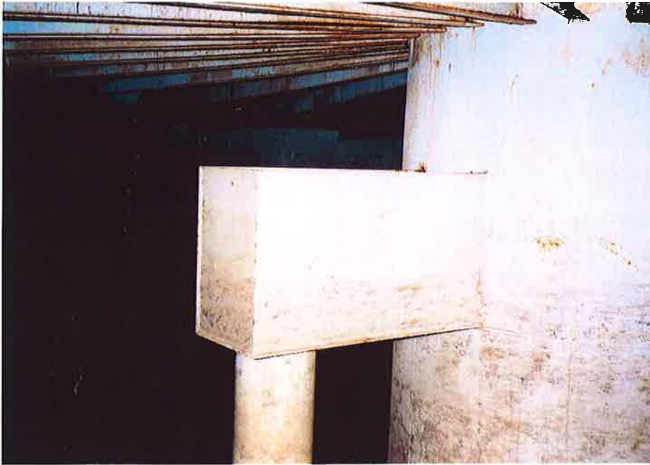
69. Overflow weir box.
