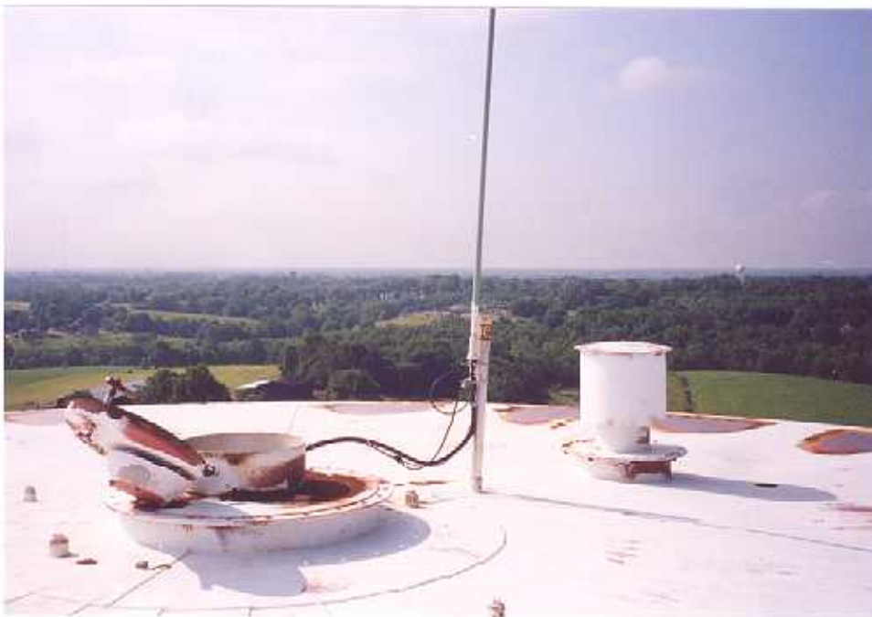
28. Corrosion on the access tube roof manhole, roof vent, and antenna.
