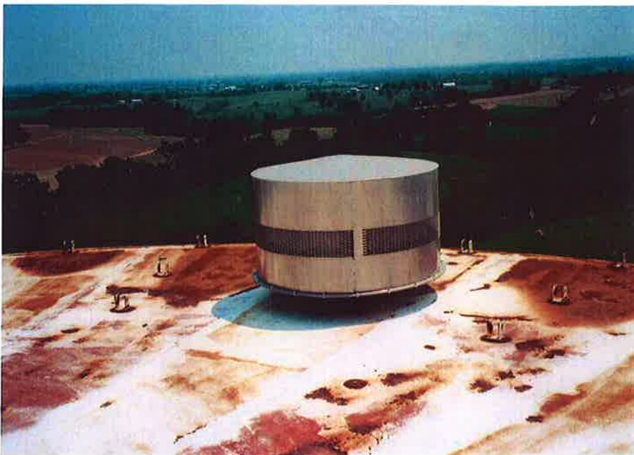
26. Roof vent. Note outrigger lugs on roof.
