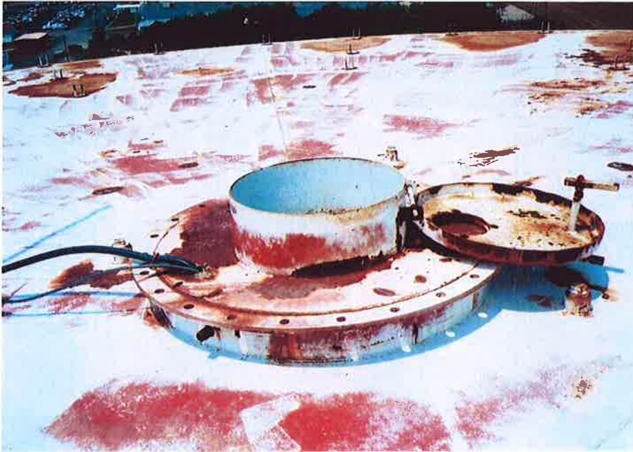
25. Access tube manhole and cover.
