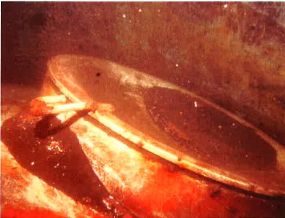
82. Manhole and cover in bowl.
