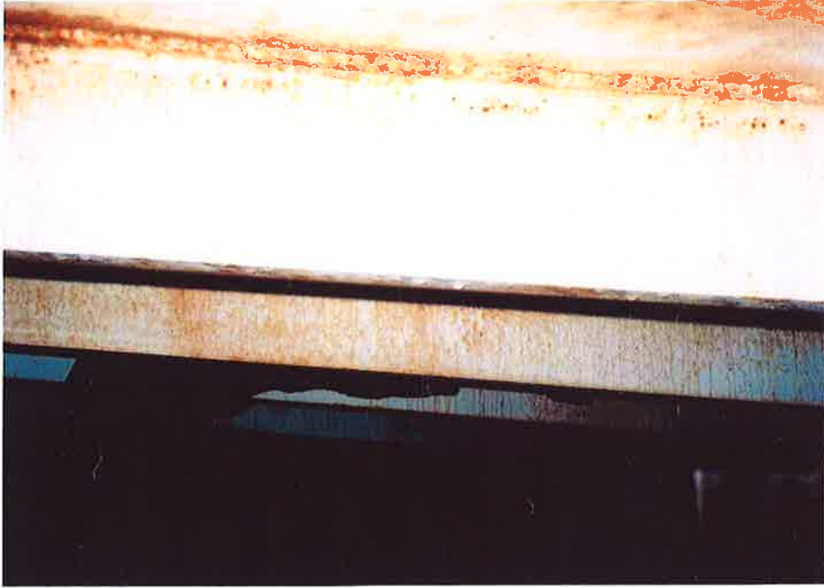
63. Corrosion on the roof support structure.
