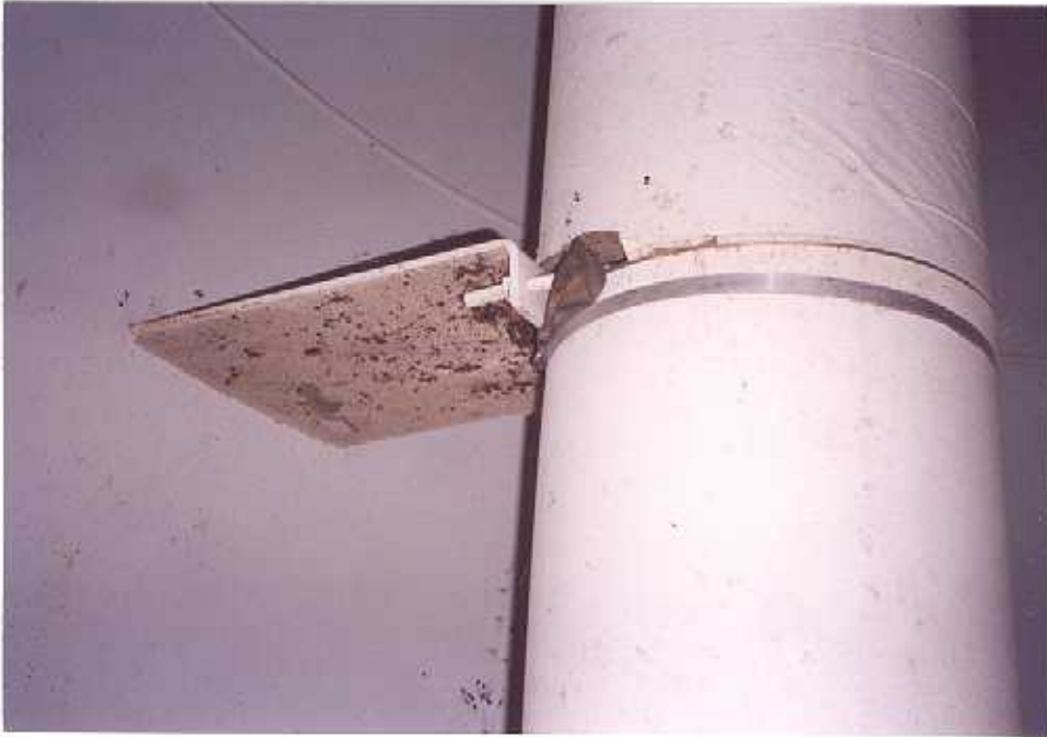
39. Inlet/outlet pipe and bracket.
