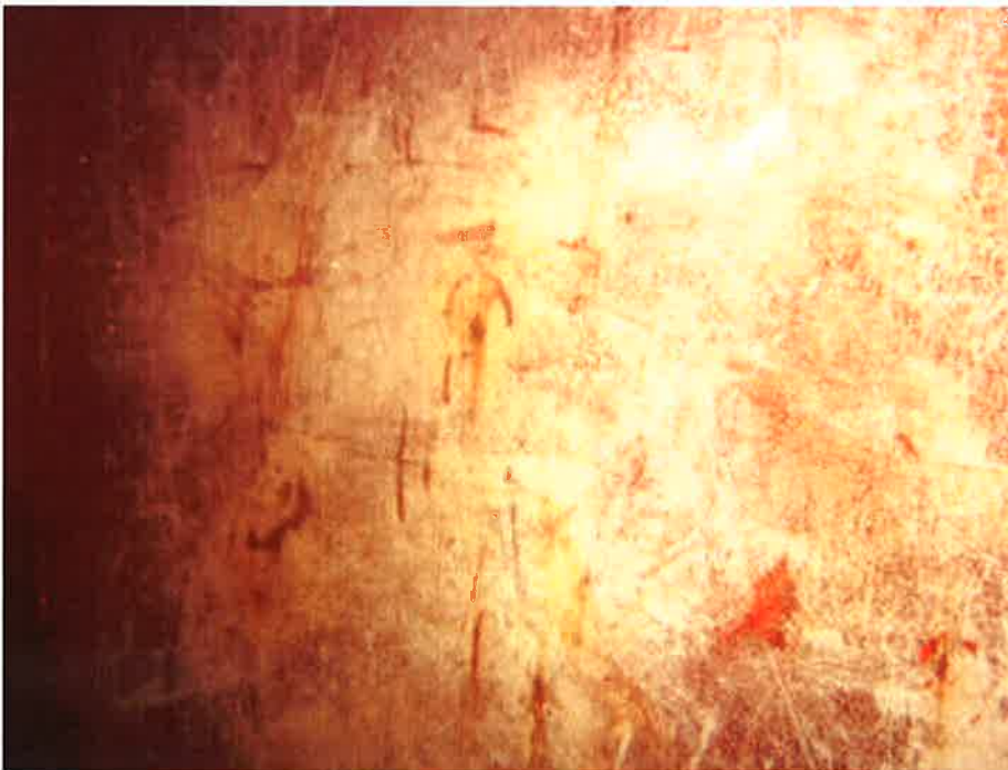
80. Corrosion on the bowl.
