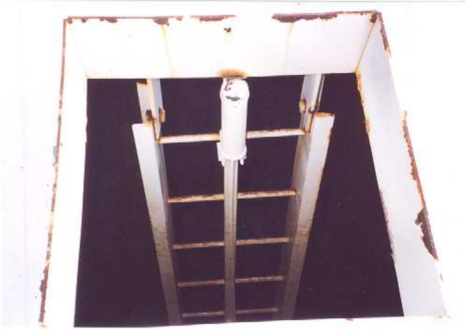
27. Roof manhole and interior container ladder.
