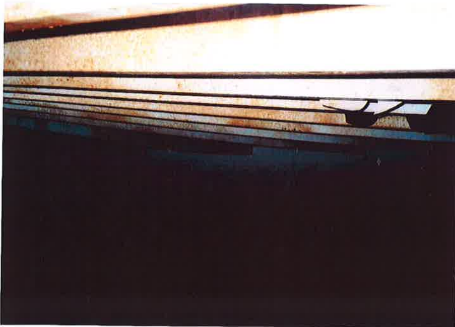
66. Coating failure on roof support structure.
