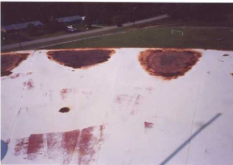
24. Corrosion, topcoat failure, and areas of accumulate water on the roof.
