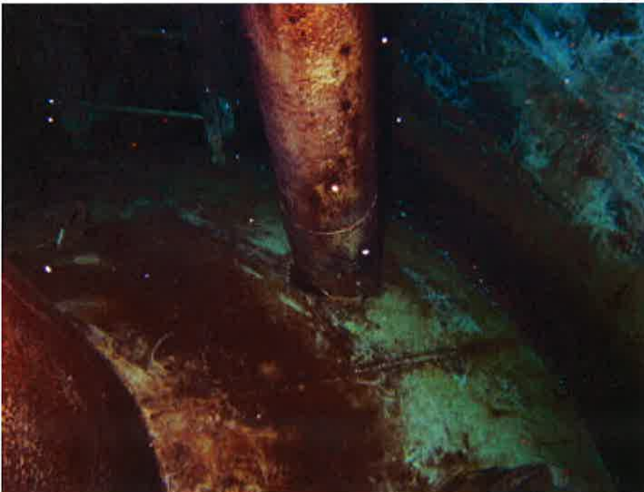
76. Container ladder base and pipe penetration in bowl of tank.
