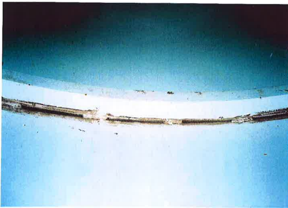
52. Intermittently welded stiffener on interior dry.
