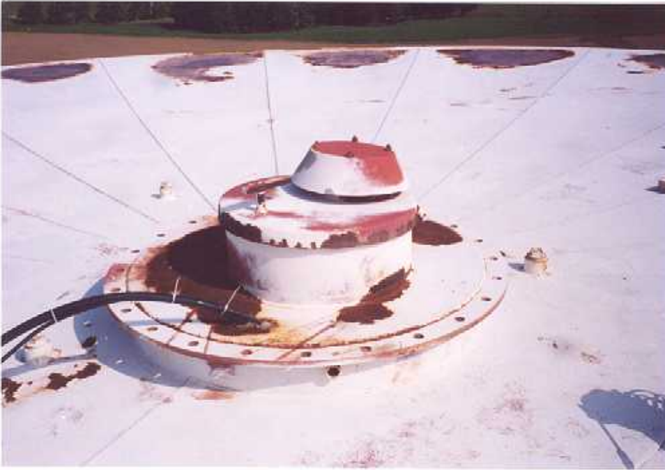
29. Corrosion on the access tube roof manhole.
