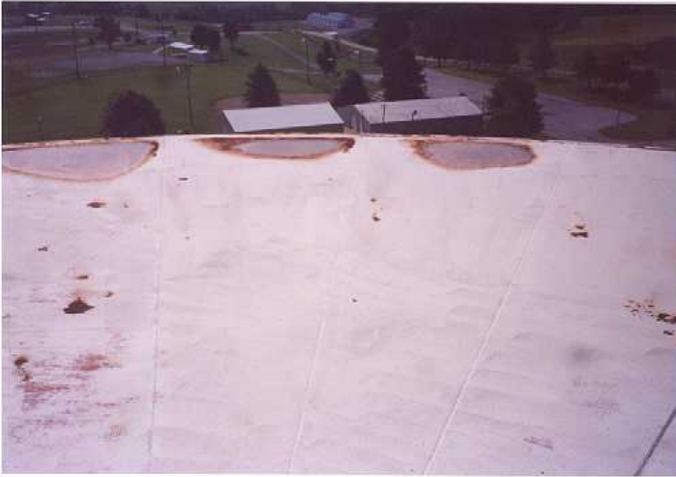
23. Corrosion, topcoat failure, and areas of accumulate water on the roof.
