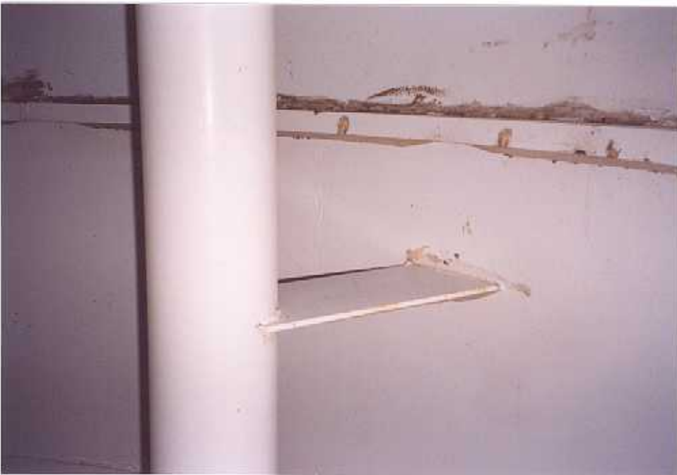
40. Overflow pipe and bracket.
