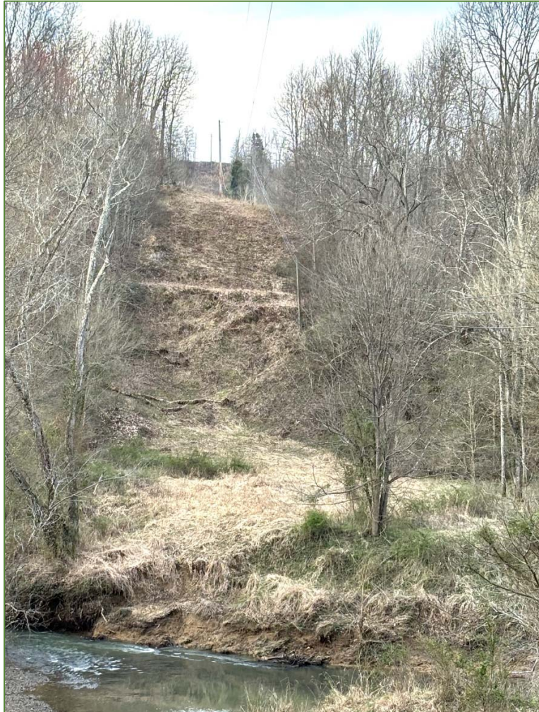
Single phase right-of-way near end segment of Big Sandy Burnaugh North Circuit
