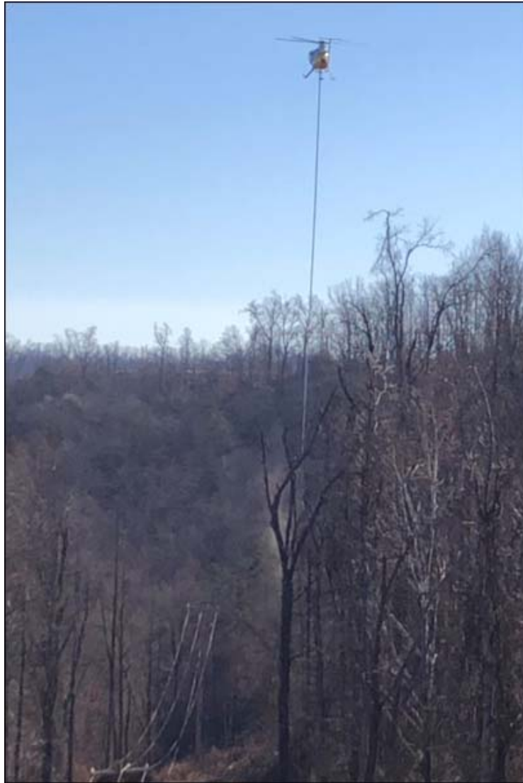
Aerial Saw Work being performed in the Ashland District on the Busseyville Mattie Circuit. This is a remote area adjacent to Yatesville Lake. Picture was taken on December 13, 2021.
