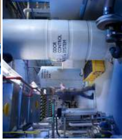
Treated Effluent Storage Tanks in Basement Equipment Room
