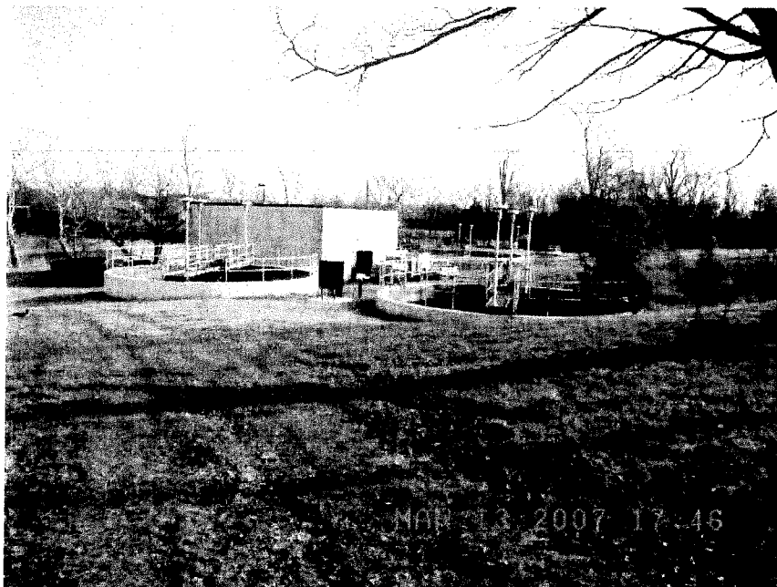
Filter Press Building and Sludge Basins at Richmond Road Treatment Plant
