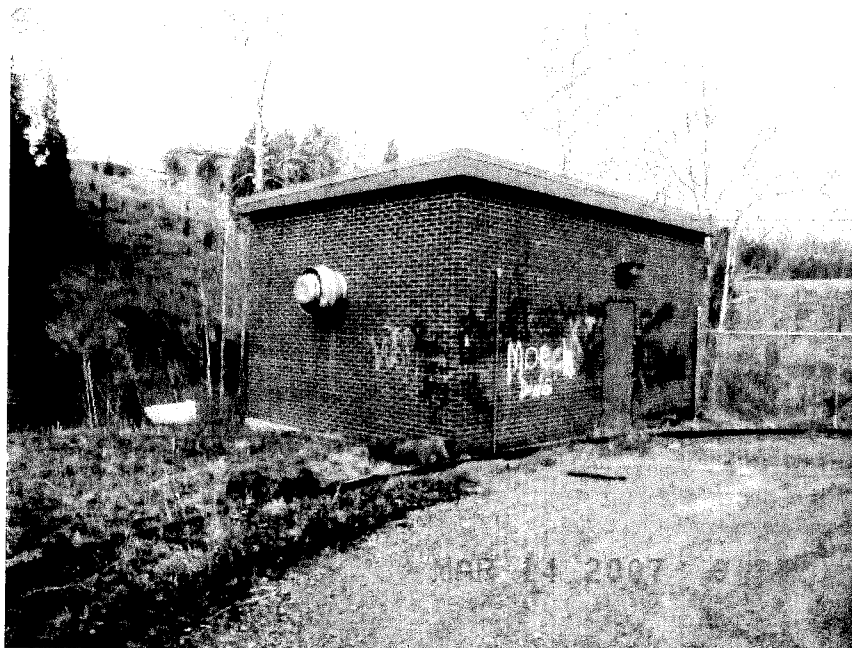
Booster Pump at Owenton Treatment Plant
