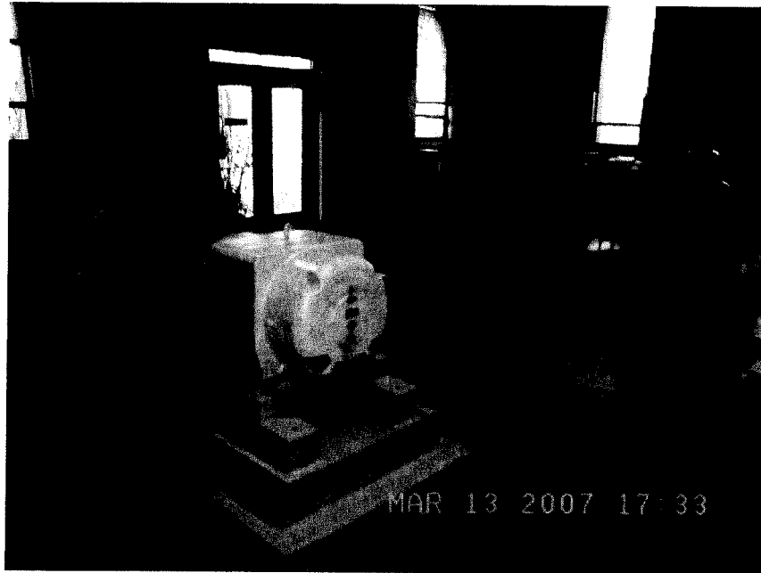
High Service Pumps #17 & #18 t Richmond Road Treatment Plant
