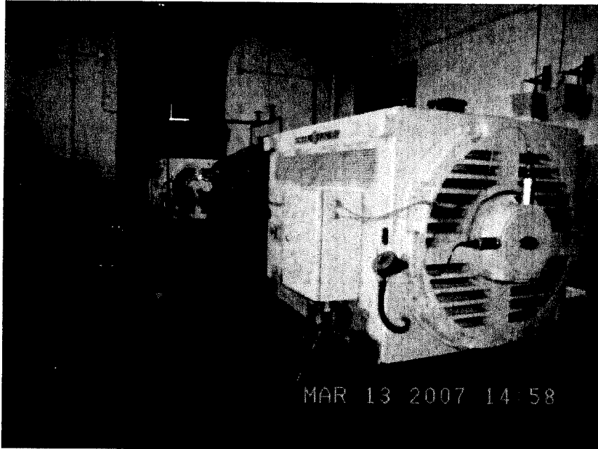
Low Service Pumps at Kentucky River Treatment Plant
