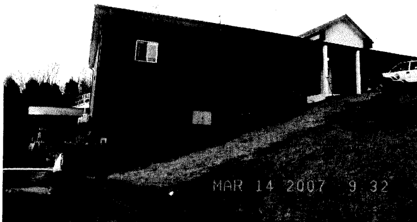
Owenton Treatment Plant
