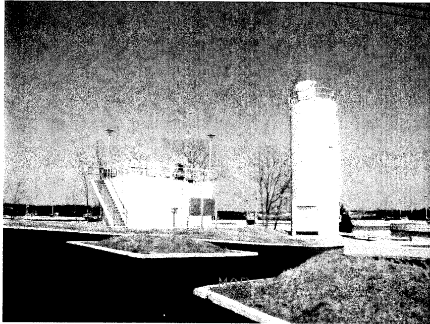
Rapid Mix Chamber and Lime Silo at Kentucky River Treatment Plant
