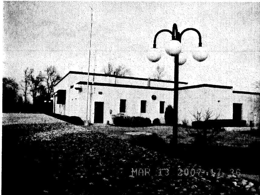
High Service Building at Richmond Road Treatment Plant
