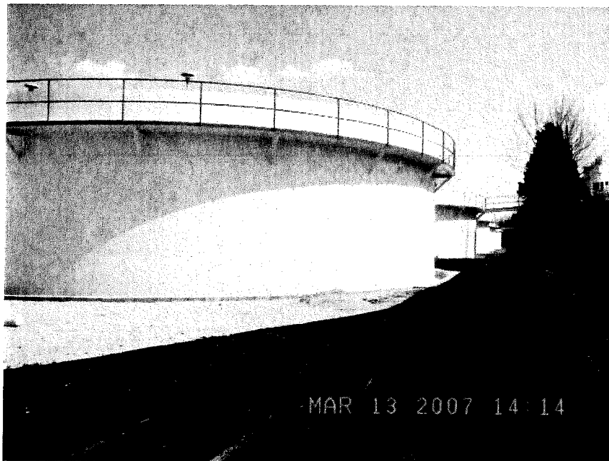
Aldrich Units at Kentucky River Treatment Plant
