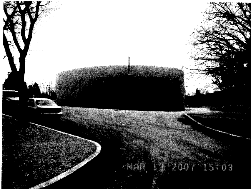
2MG Clearwell at Kentucky River Treatment Plant
