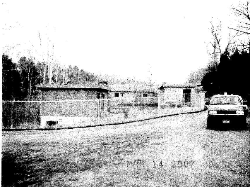
Old Owenton Treatment Plant
