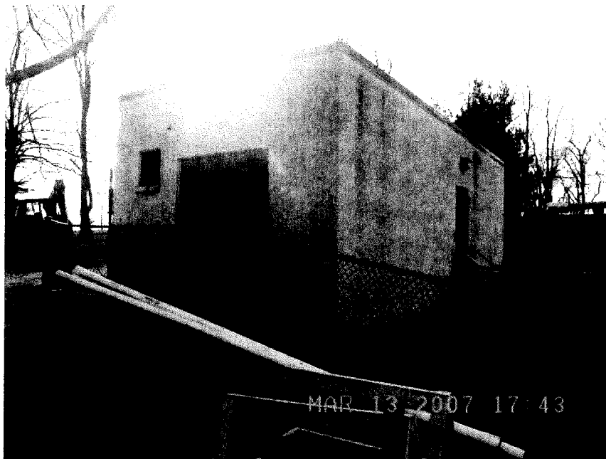
Sludge Press Building at Richmond Road Treatment Plant
