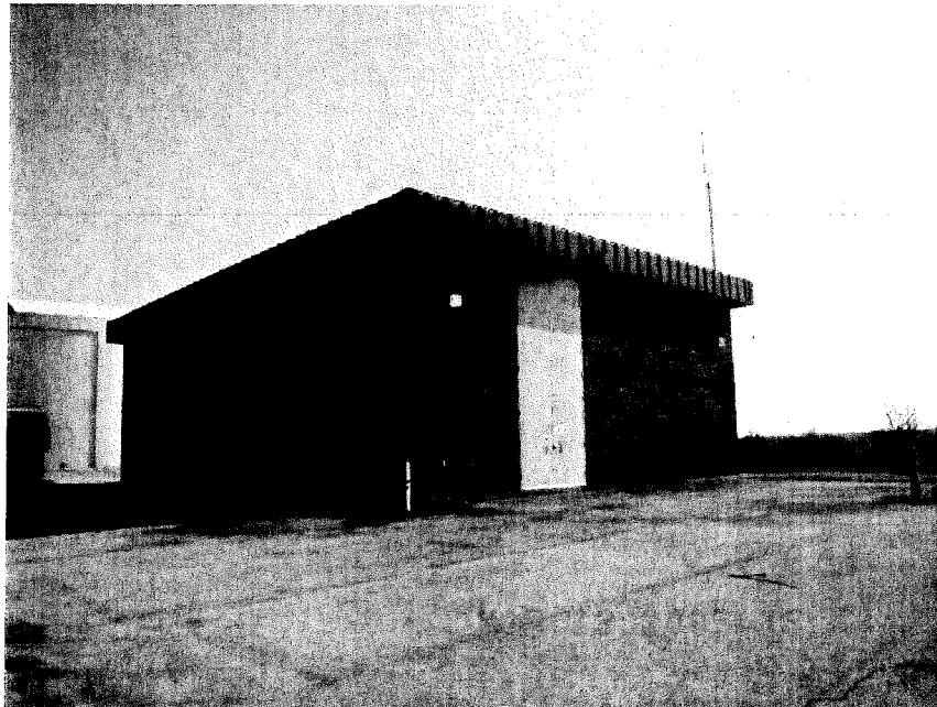
Clays Mill Booster Station
