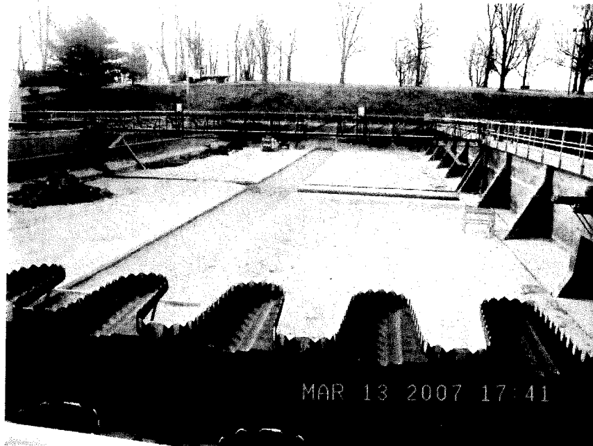
Currently being Upgraded Sedimentation Basin #1 at Richmond Road Treatment Plant
