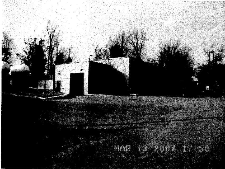
Chemical Building #2 at Richmond Road Treatment Plant
