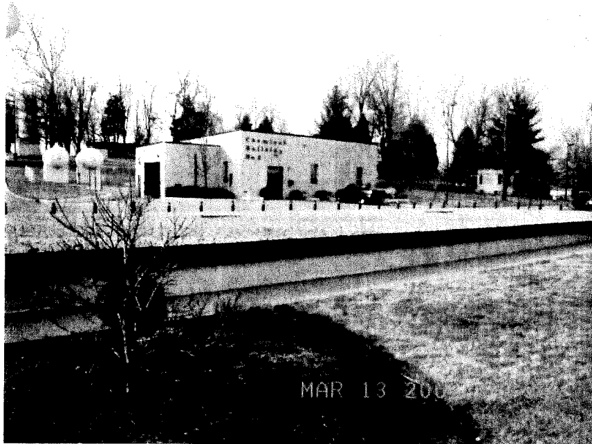
Chemical Building #2 and Clearwell at Richmond Road Treatment Plant
