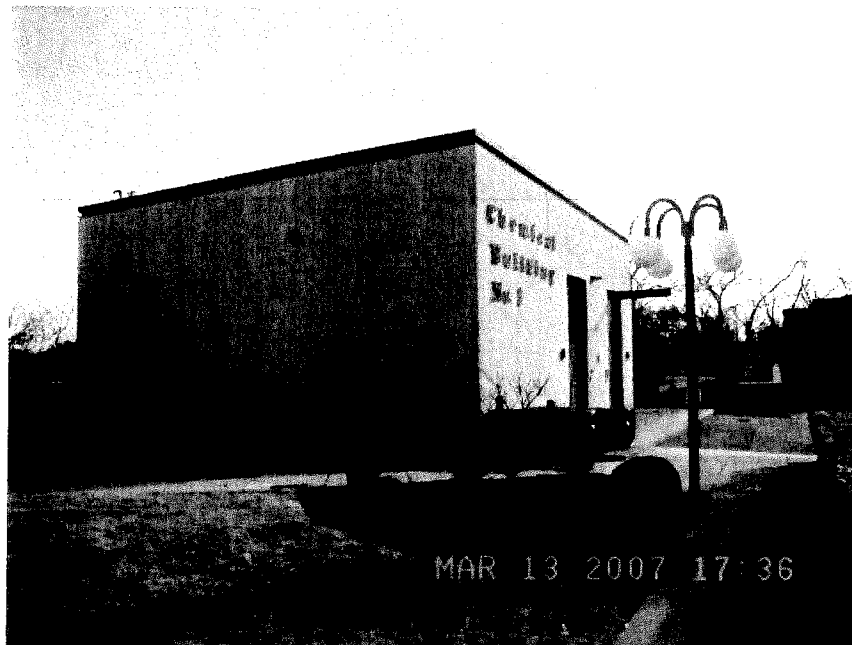
Chemical Building #1 at Richmond Road Treatment Plant
