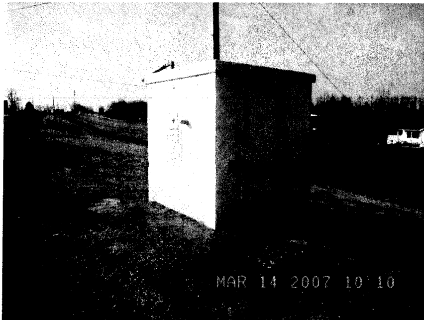
Chlorine Loading Station
