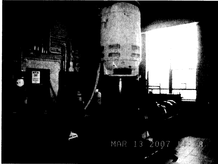
#10 Vertical Pump at Kentucky River Treatment Plant
