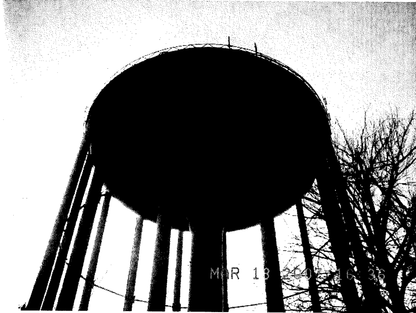
Mercer Road Standpipe
