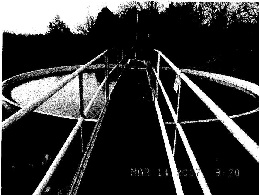
Claircone at Owenton Treatment Plant
