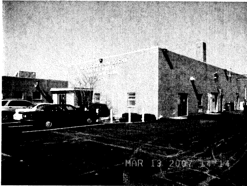
High Service Building at Kentucky River Treatment Plant
