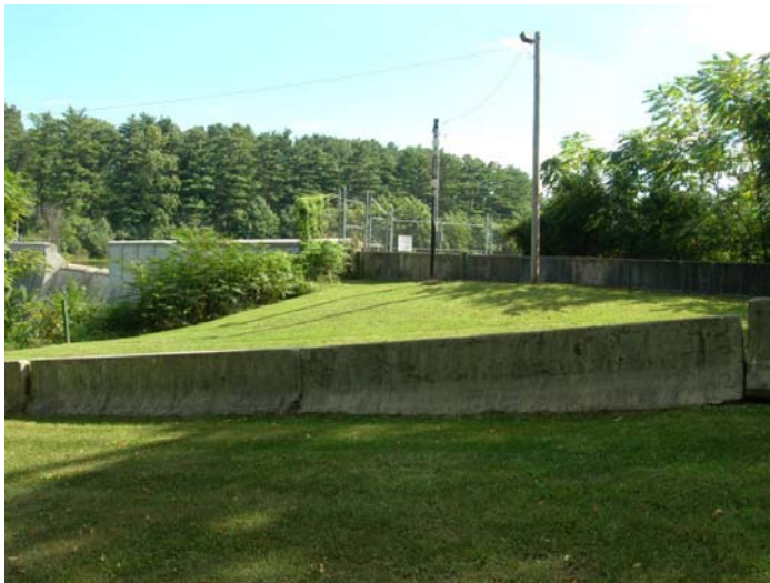
Exhibit V-9 Coatesville Retaining Dam on Reservoir as of December 31, 2007
