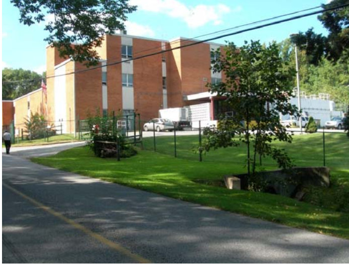
Exhibit V-8 Coatesville Water Treatment Plant as of December 31, 2007
