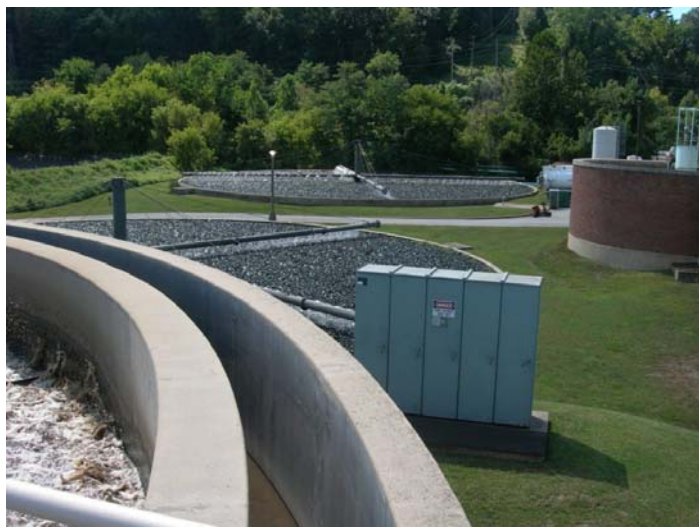
Exhibit V-7 Coatesville Wastewater Treatment Facility as of December 31, 2007
