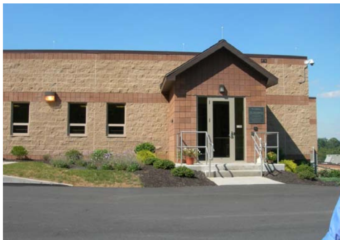
Exhibit V-15 West Shore Plant as of December 31, 2007
