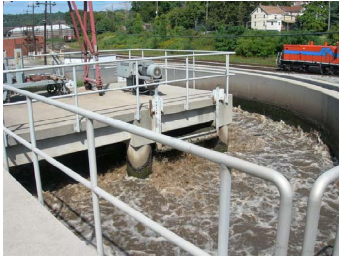
Exhibit V-6 Coatesville Wastewater Treatment Facility as of December 31, 2007
