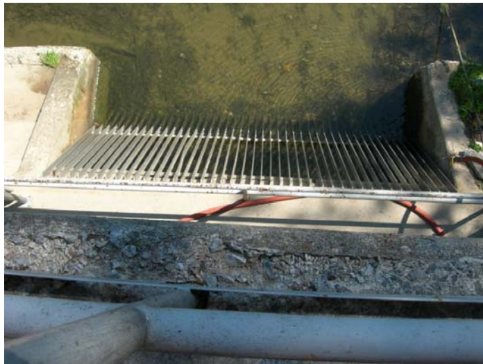
Exhibit V-11 Silver Springs Water Intake Showing Exterior Screen as of December 31, 2007
