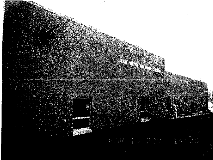
Raw Water and Chemical Building at Kentucky River Treatment Plant
