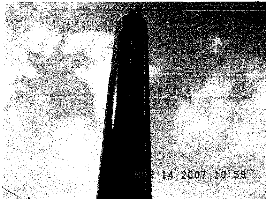
177,000 Gallon Bromley Standpipe
