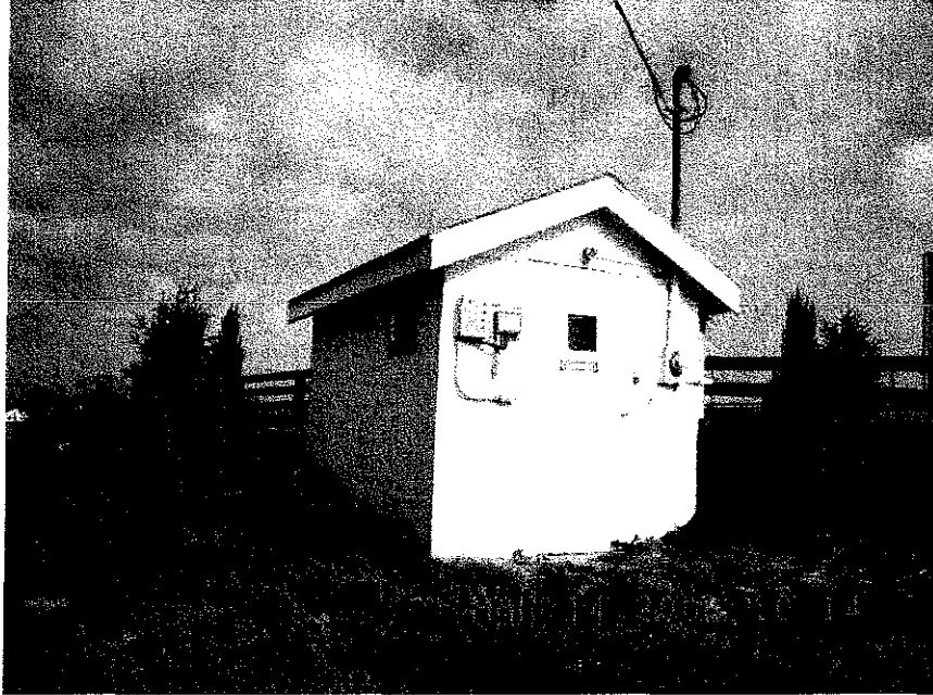
Chlorine Booster Station
