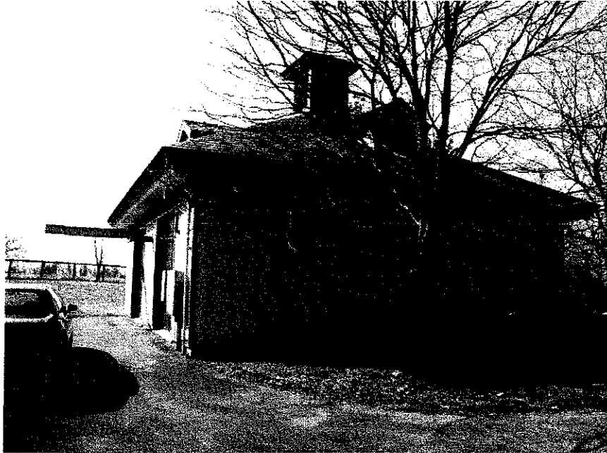
Newtown Pike Booster Station
