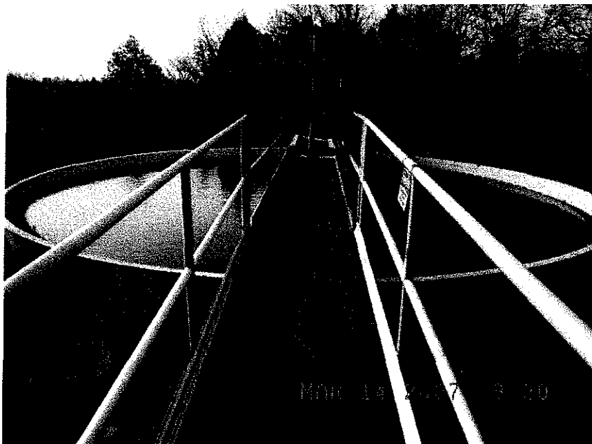
Claircone at Owenton Treatment Plant
