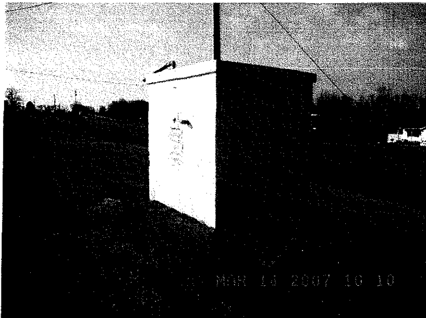
Chlorine Loading Station
