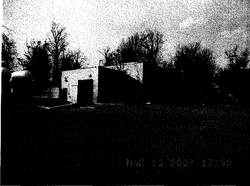
Chemical Building #2 at Richmond Road Treatment Plant
