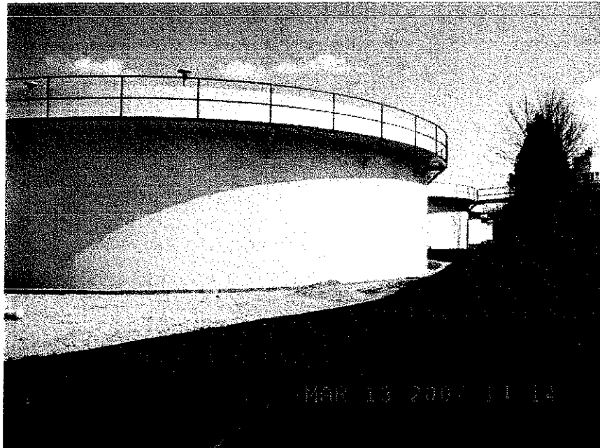
Aldrich Units at Kentucky River Treatment Plant
