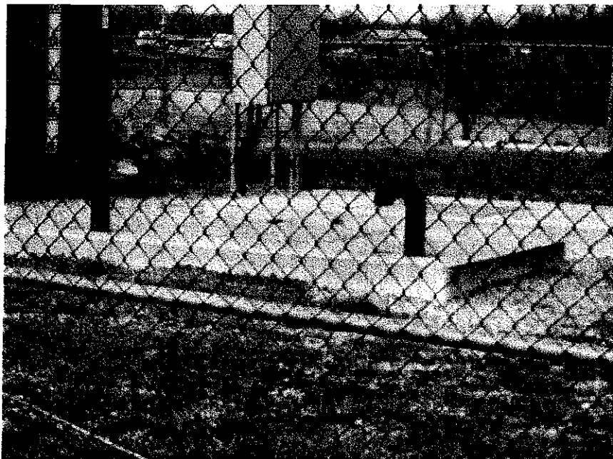
Altitude Valve Pit and Booster at Bromley Standpipe
