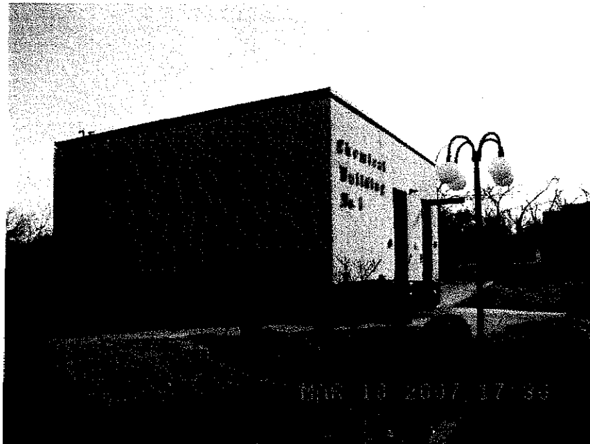
Chemical Building #1 at Richmond Road Treatment Plant
