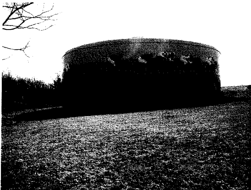
3MG Hume Road Standpipe
