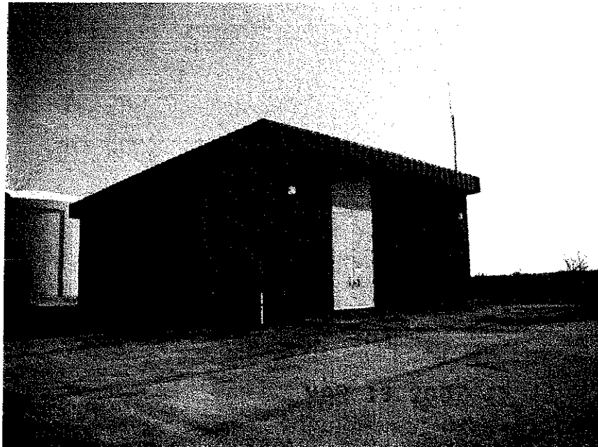
Clays Mill Booster Station
