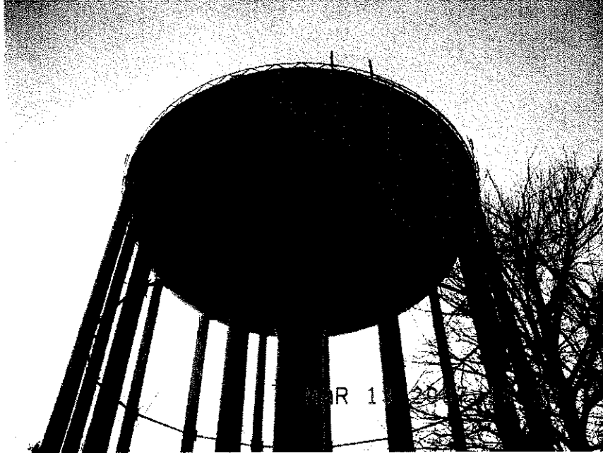
Mercer Road Standpipe
