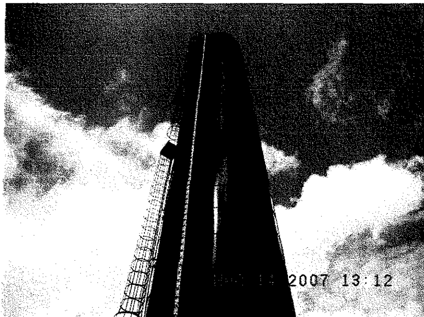
230,000 Gallon New Columbus Standpipe
