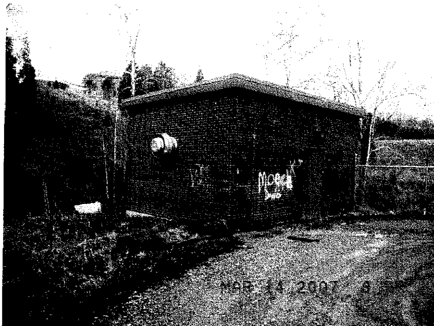
Booster Pump at Owenton Treatment Plant
