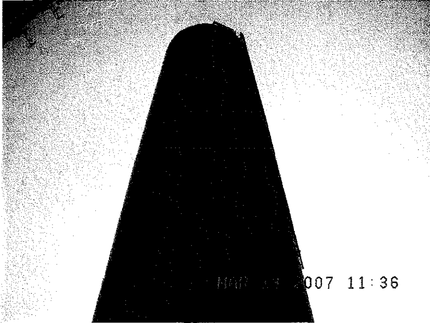
200,000 Gallon Hall Standpipe
