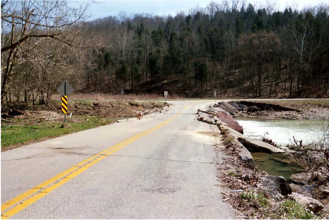
Exhibit C-8. Corn Creek Bridge from State Highway 625
