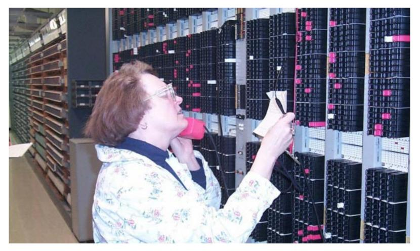
Step 6: Technician walks along Main Distributing Frame to locate both ends of jumper to be cut.
