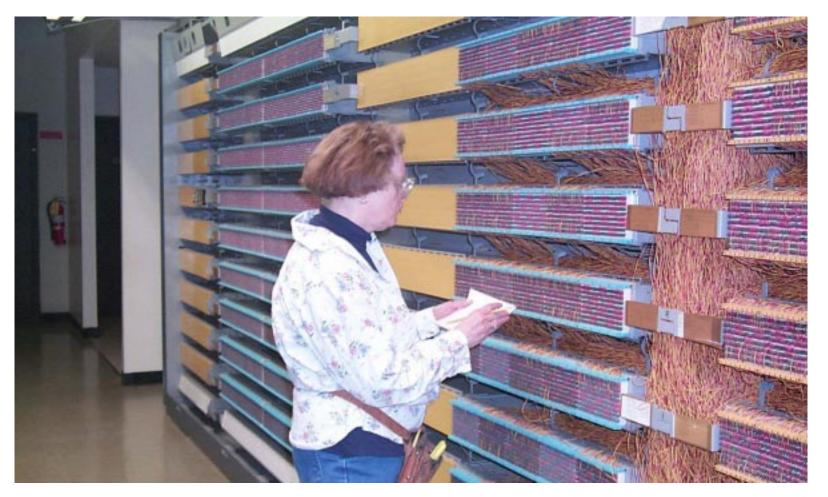
Step 8: Technician locates and removes end of jumper connected to the BellSouth cable pair.
