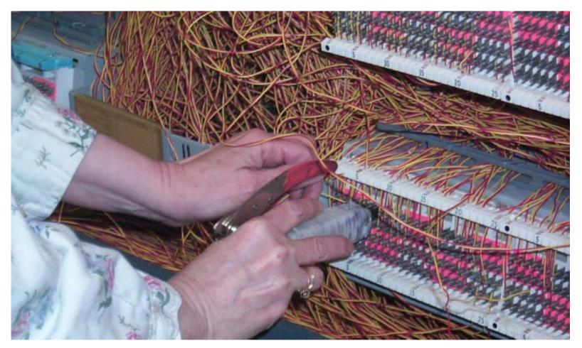
Step 13: Technician conducts ANAC test to verify that loop has been cut to correct CLEC switch port.
