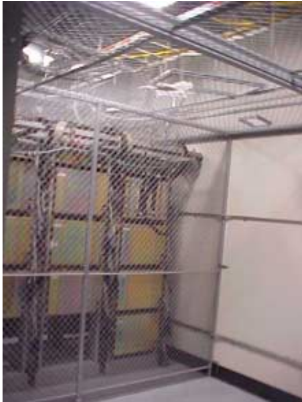
Collocation Cage (Empty—Looking Out)
