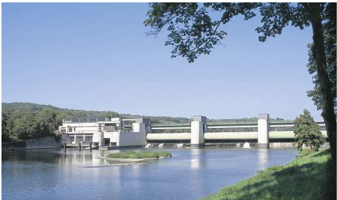
Baldeneysee, Essen, Germany: RWE run-of-river power plant
