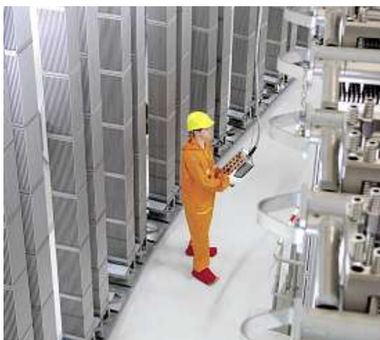
Biblis nuclear power plant: storage of fresh fuel elements
