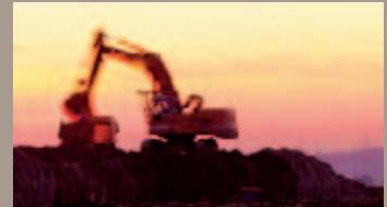
Excavation works in Neurath (GER)
