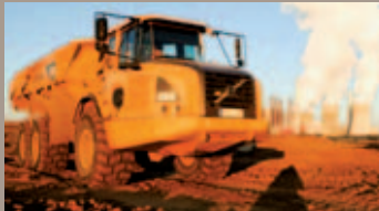
Removal of excavated earth
