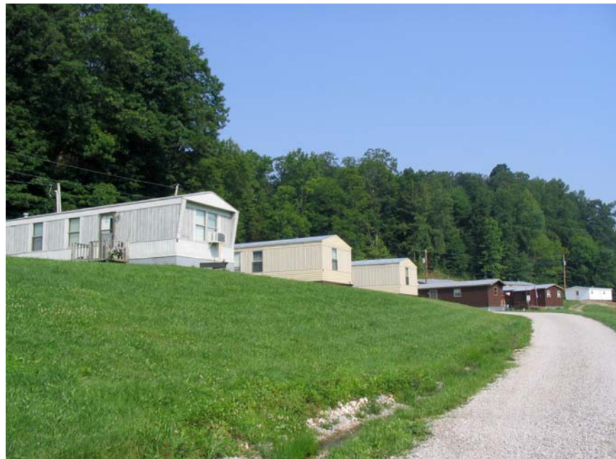
Photograph 3 Homes off Coal Wash Road Photograph taken by Brighton A & E, Inc., from Coal Wash Road. June 29, 2004
