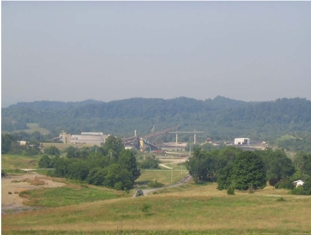
Photograph 6 - Existing Site Looking at Location of Proposed Power Plant Photograph taken by Brighton A & E, Inc., Dated June 29, 2004
