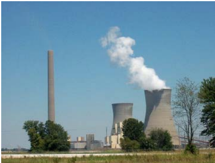
View of Plant from Fulkerson east line
