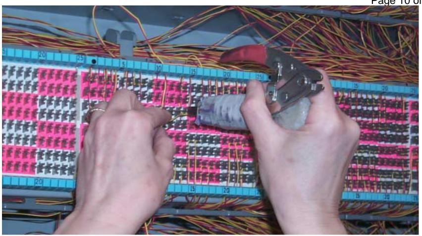
Step 11: Technician weaves wire through cable rack to reach tie cable to CLEC's collocation equipment.
