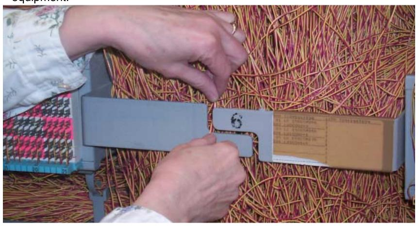
Step 12: Technician connects new jumper on frame to tie cables to CLEC equipment.
