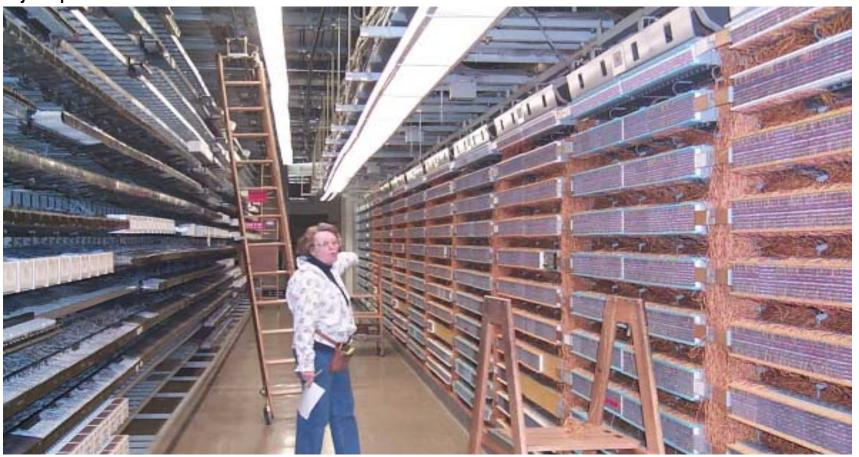
Step 7: Technician locates precise location of jumper.
