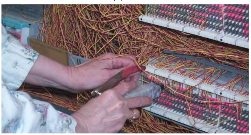
Step 13: Technician conducts ANAC test to verify that loop has been cut to correct CLEC switch port.
