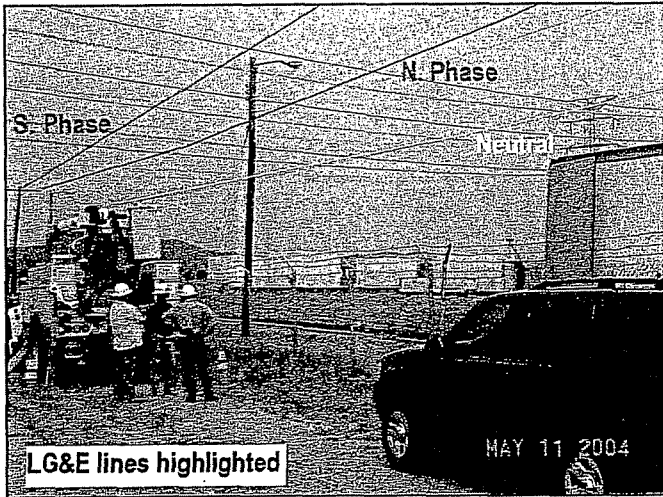
VIEW 1: NEAR CONTACT POINT - FACING NW
