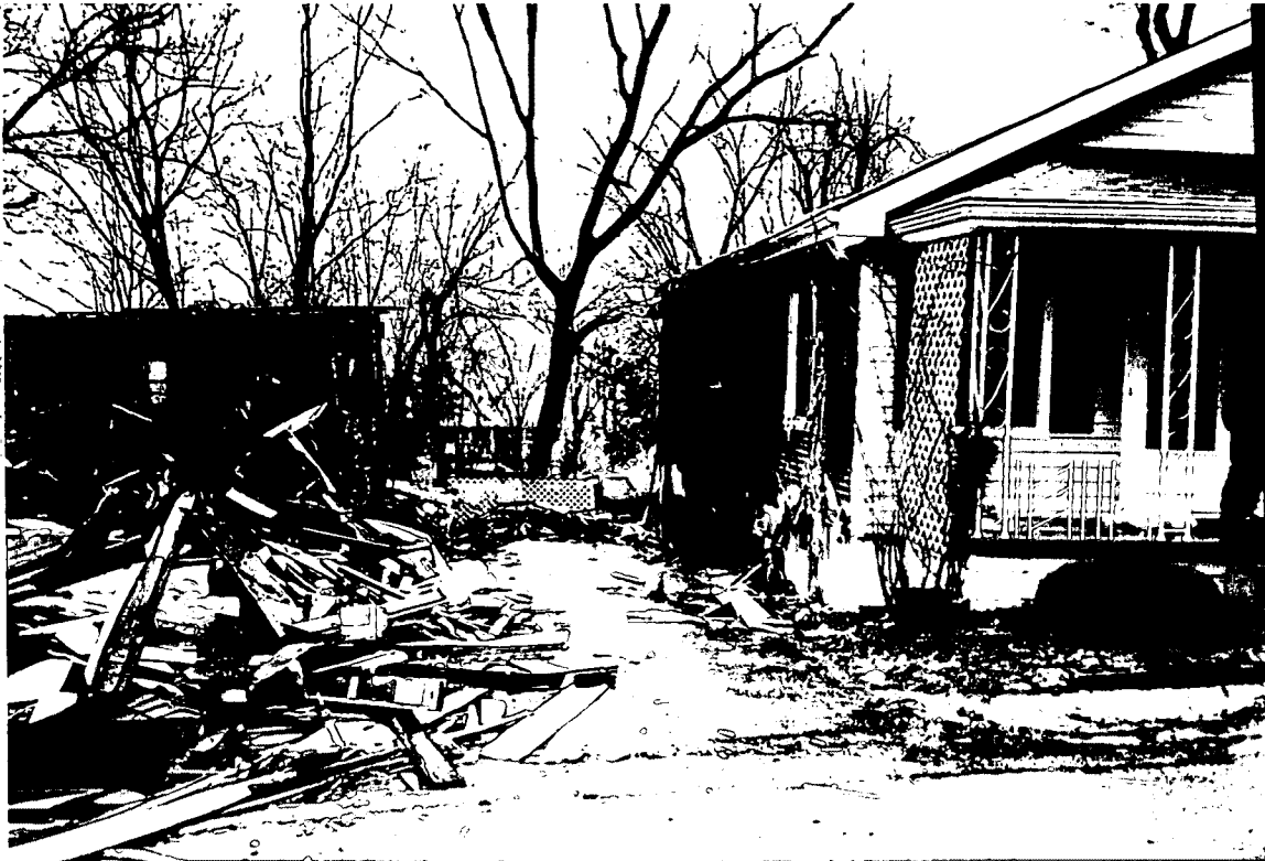
PHOTOGRAPH 1 - Front and east side of house. Debris covering area of curb valve location. West side of 509 Smith Street also shown. (3/5/97)
