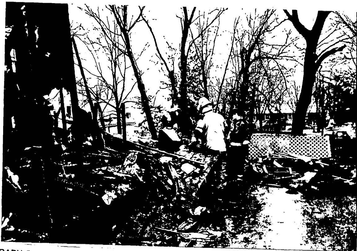
PHOTOGRAPH 5 - Fire department representative sawing opening in floor. Taken looking north from northeast corner of drive between 511 & 509 Smith Street (3/5/97).
