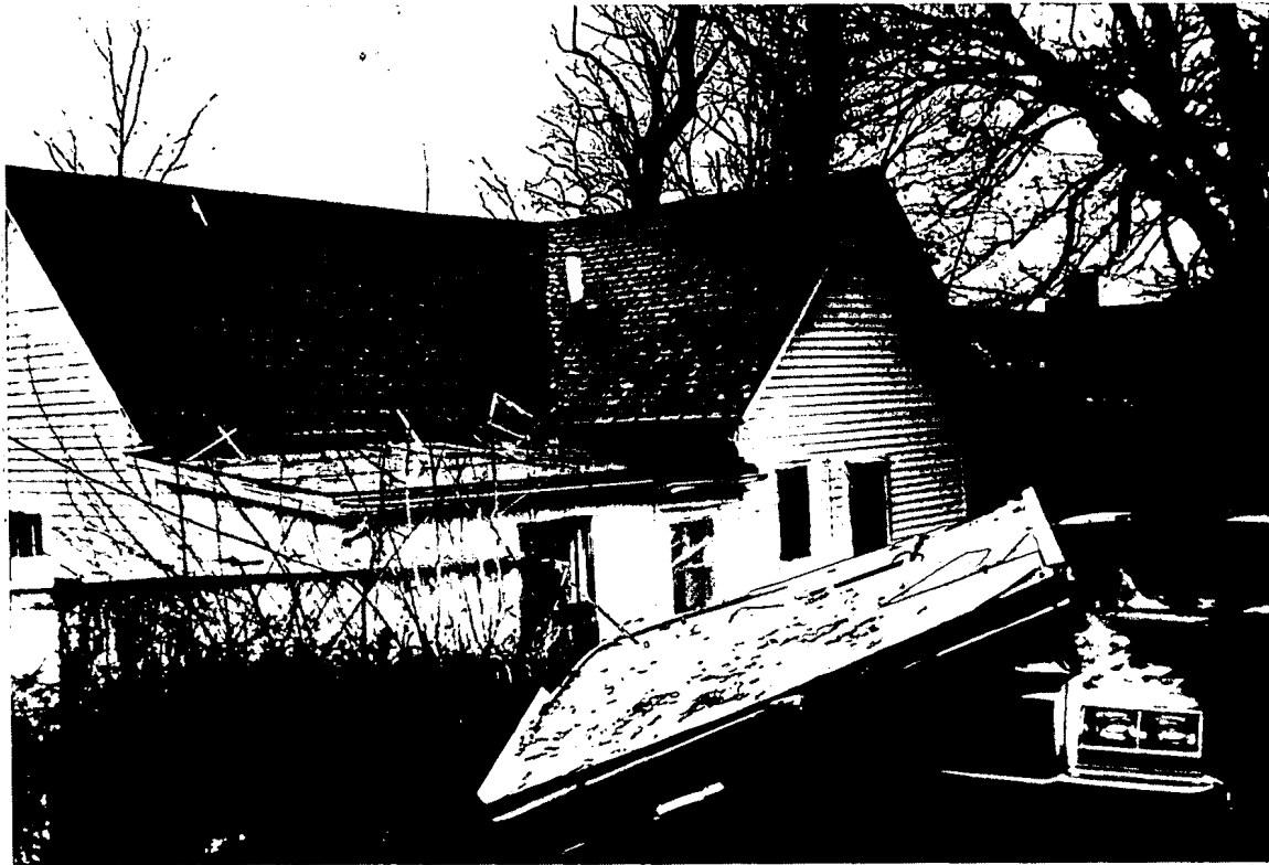
PHOTOGRAPH 4 - Portion of wall of house looking northwest from front. Also shown is east side of 402 6th Street with debris and explosion damage. (3/5/97).
