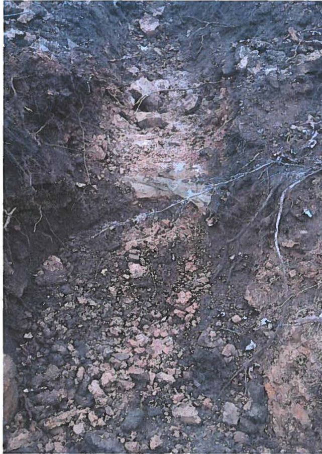
Sandstone Bottom of Trench
