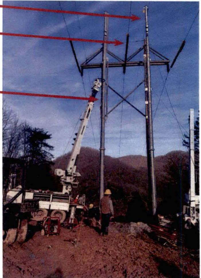
Steel bar and strap used to cant the pole
