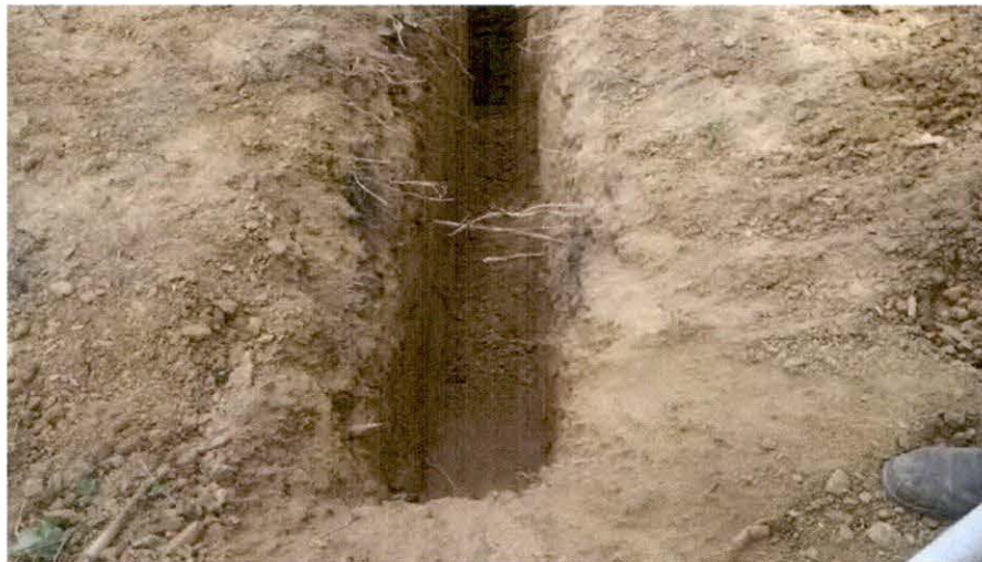
Sandstone Bottom of Trench
