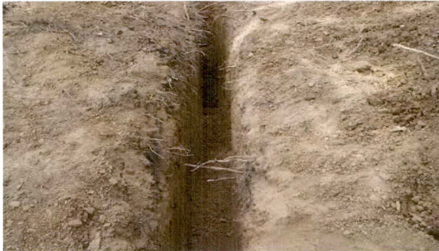
Sandstone Bottom of Trench
