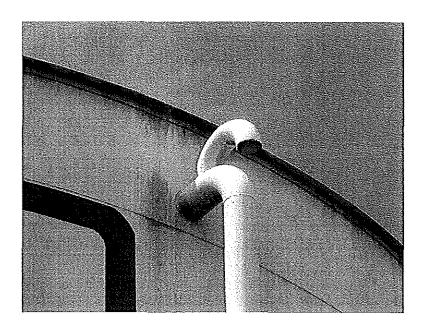
Photo shows a vent pipe attached to the overflow pipe where it exits the tank's upper two foot shell panel.
