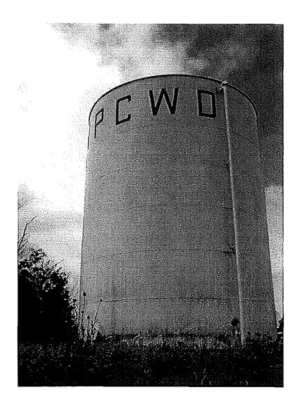
Photo shows an overall view of the northeast side of the tank. Mildew covers most surfaces. No rust was noted. The overflow pipe is located on this side of the tank.
