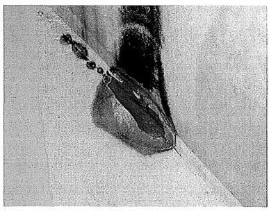
Photo shows severe metal loss along a shell to floor weld on the northeast side. The pitted areas will need to be repaired by welding.
