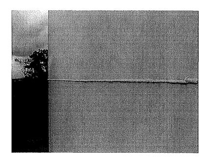
Photo shows the lower middle west shell. All weld seams appear structurally sound.
