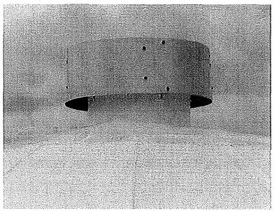
Photo shows the 24" diameter roof vent pipe with an aluminum cover. The insect screen could not be inspected since the roof was too steep to gain safe access.
