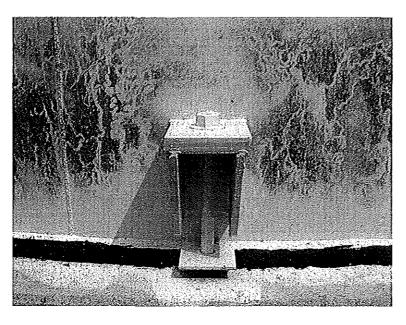
Photo shows one of the 1½" diameter anchor bolts. The chairs are wide enough to provide access to the backsides of the bolts. The bottom plate is unnecessary and should be removed.
