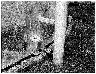
Photo shows the base of the north shell covered with mildew. The 8" diameter overflow pipe discharges below grade. The drainpipe ties into the overflow pipe and has a valve.
