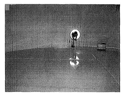
Photo shows the northwest section of the floor and the shell manway. Numerous corrosion cells are visible along the floor to shell panel weld seam.
