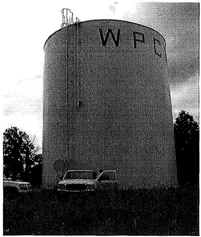
Photo shows the southwest side of the tank. Coating coverage is good. The white finish coat is chalky.
