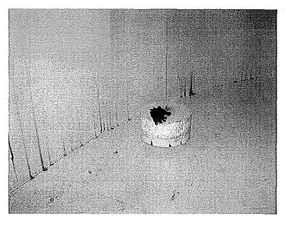
Photo shows the float in the empty position. Numerous active corrosion cells are visible along the shell to floor weld seam. The DFT on the lower shell ranged from 9.0-14.8 mils and averaged 11.96 mils.
