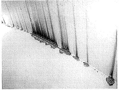
Photo shows the shell to floor interface with the rust nodules removed with the 4,000-psi pressure washer. Severe metal loss was noted.
