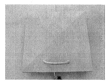
Photo shows the 24" square roof access hatch. The hatch was not secured with a lock.
