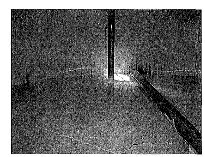
Photo shows the north section of the floor. The tank has two fill pipes to help with water turn over.
