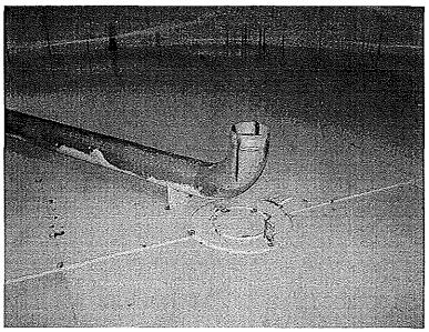
Photo shows the lower fill pipe in the center of the tank floor. Scattered active corrosion cells are visible.
