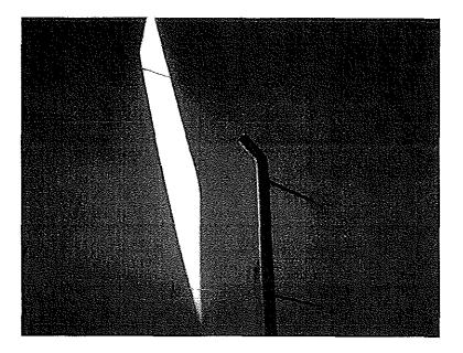
Photo shows the north shell and the stainless steel fill pipe. Scattered active corrosion cells are visible.
