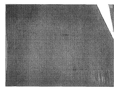
Photo shows the southwest middle shell panels. If the weld seams had been stripe coated only minor coating failure would be present.
