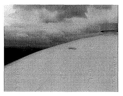
Photo shows the northwest section of the roof. One spot where the epoxy intermediate coat is exposed and has faded was noted.
