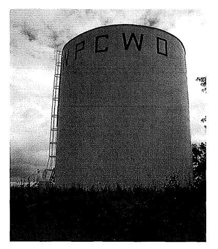
Photo shows an overall view of the south side of the ground storage tank. The tank has six 8' tall ring sheets and one 2' tall ring at the top for a total of a 50' shell.
