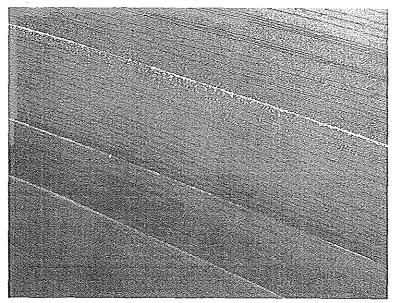
Photo shows the southwest middle section of the roof. Overall the white epoxy coating continues to provide very good protection. Minor rust is visible along the seams.
