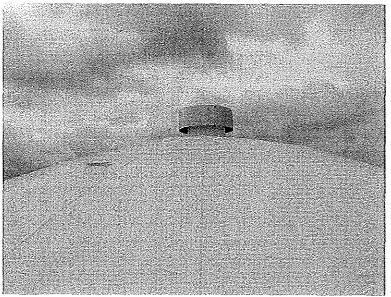
Photo shows the center section of the roof with the vent located at the apex. A handrail should be extended to the vent to allow safe access on the steep roof.
