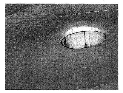
Photo shows the center section of the roof with the vent pipe in the middle. Crevice corrosion is visible along the roof seams and along the pipe to roof panel connection.
