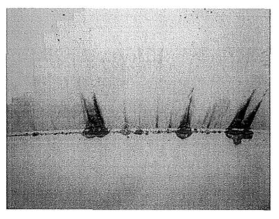
Photo shows a series of pits along the shell to floor interface on the southeast side. Metal loss is active.
