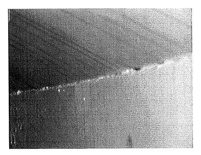
Photo shows active crevice corrosion along the roof to upper shell panel interface.
