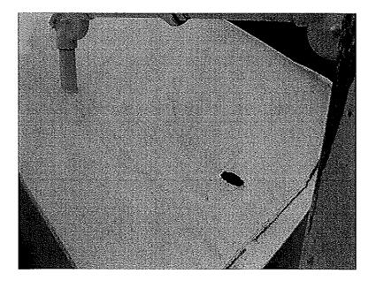
Photo shows a rusty spot on the west outer section of the roof. The coating has delaminated to the steel substrate.
