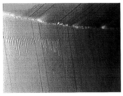
Photo shows active crevice corrosion along the roof to upper shell panel interface on the north side. Runs are visible where the last paint crew rolled a heavy coat into the joint.
