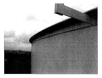
Photo shows mildew along the stiffener angle at the top of the northwest shell.
