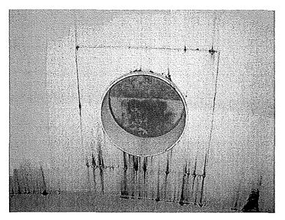
Photo shows the northeast shell manway. Active corrosion is visible along the weld seams of the reinforcing plate.
