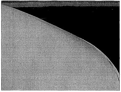
Photo shows the outer southwest section of the roof. The average DFT was 9.84 mils.
