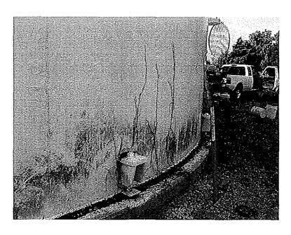
Photo shows vines attached to the northwest lower shell and mildew. The concrete foundation projects above grade.
