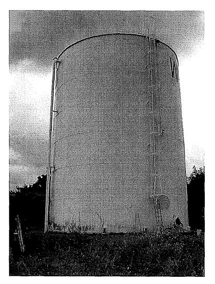
Photo shows an overall view of the northwest side of the tank. The caged shell ladder is located on the west side. Handrails should be extended 10' to each side of the shell ladder along the edge of the roof. The 8" diameter overflow pipe is located on the north side.
