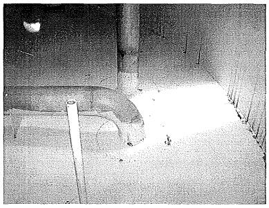
Photo shows the point where the two fill pipes enter the tank floor. The stainless steel pipes are partially coated.
