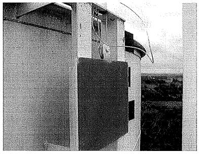
Photo shows the red target in the empty position. The float and level indicator were in good condition.
