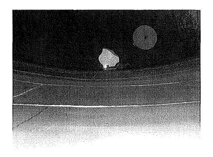
Photo shows a view looking down the west shell from the roof access hatch. The tank does not have an interior ladder. Minor coating failure is visible along the weld seams.
