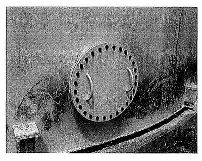
Photo shows the northeast shell manway. The bolts are rusty. At the next maintenance event a new gasket and new stainless steel bolts and washers should be installed. New brass nuts should be installed to prevent galling.
