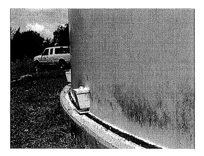
Photo shows the south lower shell and one of 14 anchor bolts. Mildew covers the lower tank surfaces. The steel to concrete interface was sealed with a tar like substance.
