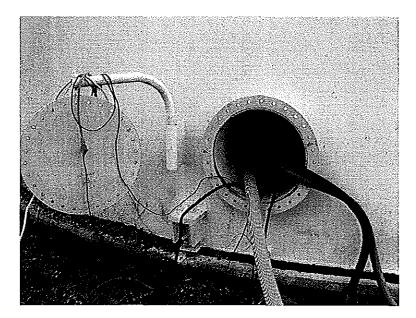
Photo shows the southwest shell manway. The 24" diameter bolted flange manway has a davit arm that functioned properly. The davit arm is not necessary and should be removed as many times they become frozen in place making access difficult.
