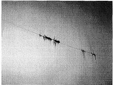
Photo shows large rust nodules along a horizontal weld seam.
