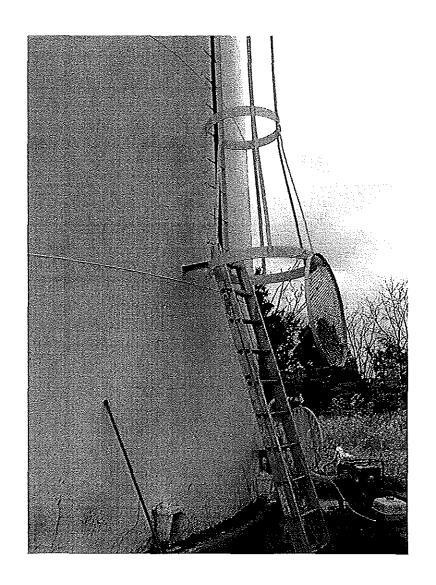
Photo shows the lower west shell and the bottom of the caged ladder. The ladder has a hinged climb prevention shield to prevent unauthorized access.
