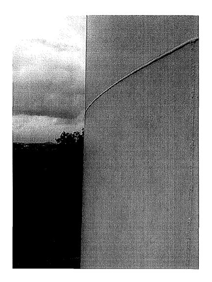
Photo shows the middle shell panels on the west side. Coating coverage is excellent. Minor mildew is visible along the bottom of the weld seams.
