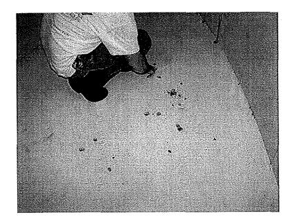
Photo shows a cluster of rust nodules in the middle of the floor panels. Metal loss is active. If left unrepaired leaks will soon develop.
