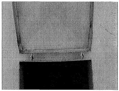
Photo shows the hatch hinges. Minor rust is visible but the hinges appear to be structurally sound.
