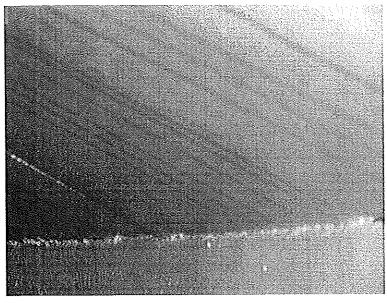
Photo shows another view of the south outer roof and upper shell panel. This joint will need to be sealed with a flexible caulk such as Sika Flex-1A after the new coating system is installed.
