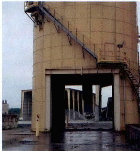
Figure 3-5: U4 Fly Ash Loading Operation
