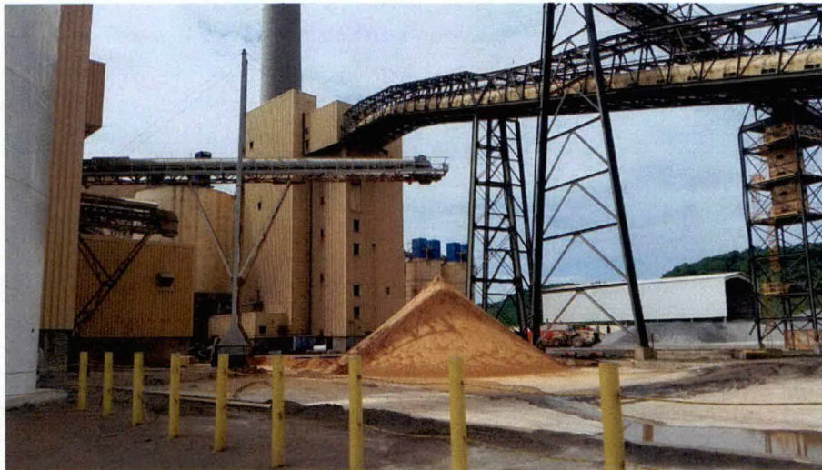
Figure 3-6: Gypsum Pile and Loadout Operations
