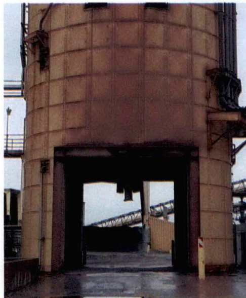
Figure 3-4: U4 Bed Ash Loading Operation
