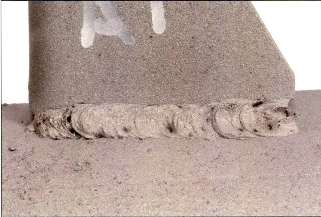
Figure 4. Image of the Lug A1 exterior top weld which exhibited substantial fusion except for some overlap and undercut.
