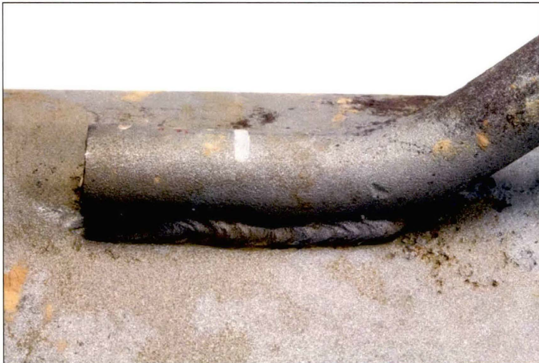
Figure 3. Image of the Rod Side A top joint region showing the attachment weld.
