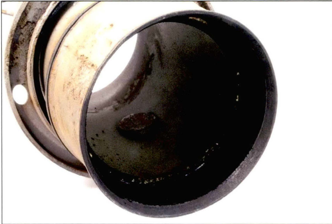
Figure 11. Image looking into the interior of the coupling which remained affixed to pipe End A.
