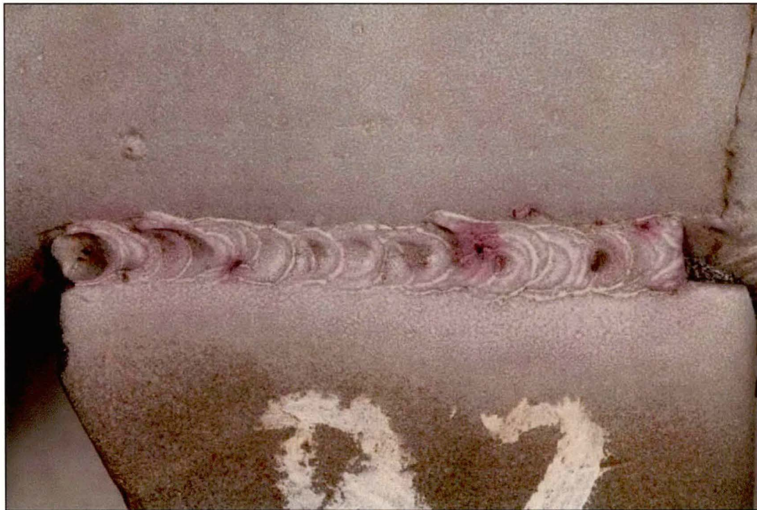
Figure 13. Image of the Lug B2 exterior top weld after dye penetrant media had been used during inspection.
