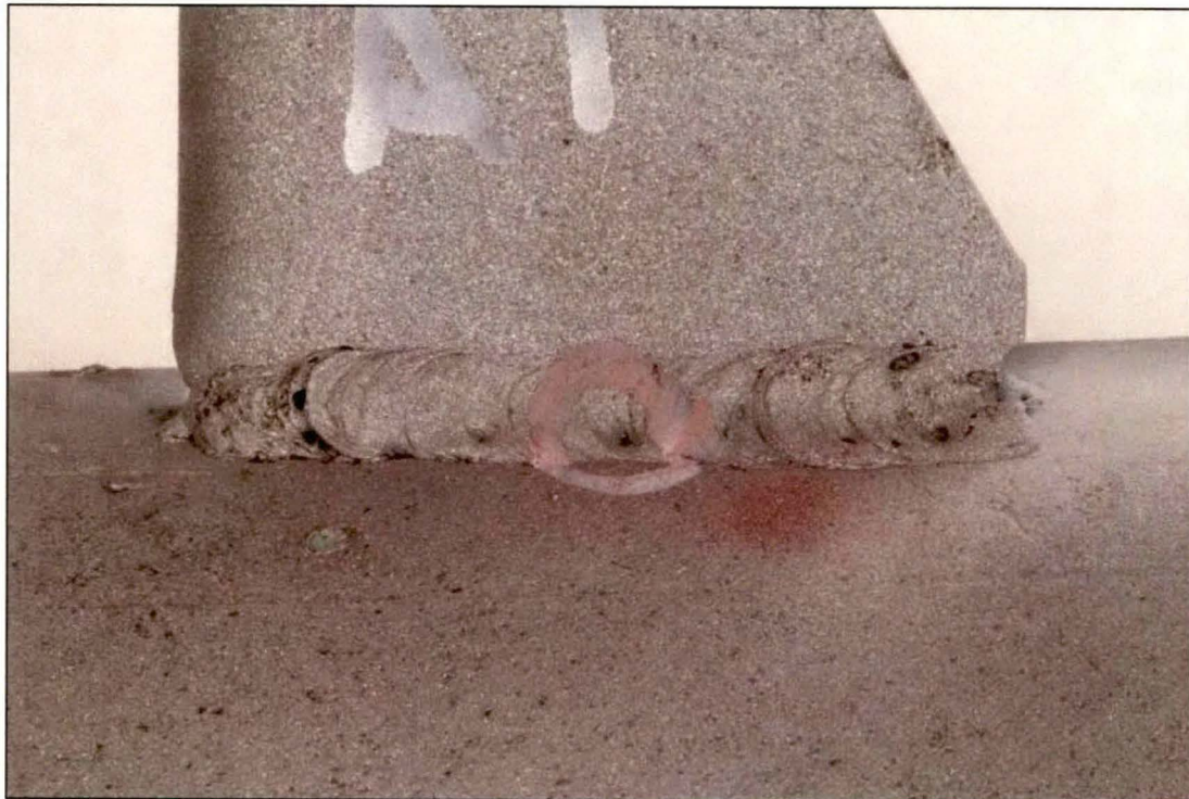
Figure 14. Image of the Lug A1 exterior top weld with a pore identified by NDE.
