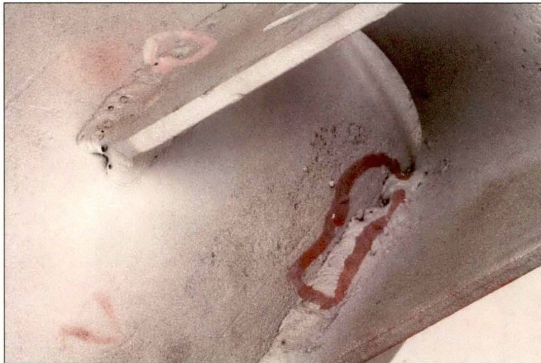
Figure 16. Image of the Lug A1 exterior top and interior top welds after dye penetrant media had been used during inspection.
