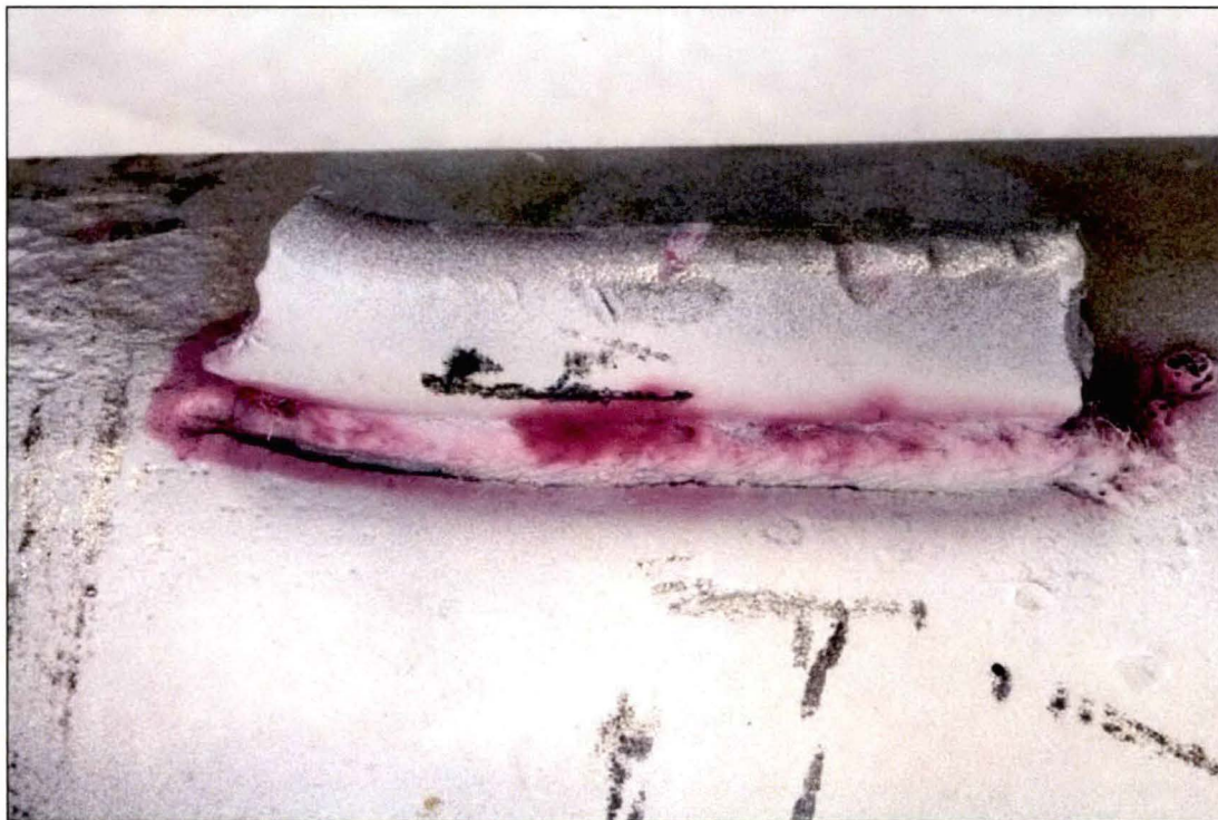
Figure 14. Image of the Rod End B top weld after dye penetrant media had been used during inspection.
