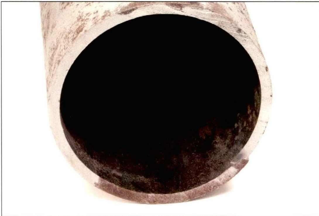
Figure 8. Image of the Pipe A section which had been in the coupling.
