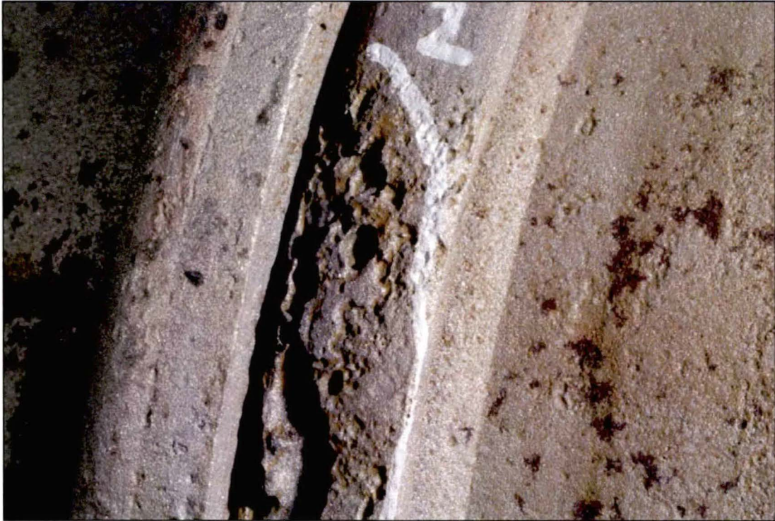
Figure 5. Image of a circled corrosion pit on the coupling identified as Location 2.
