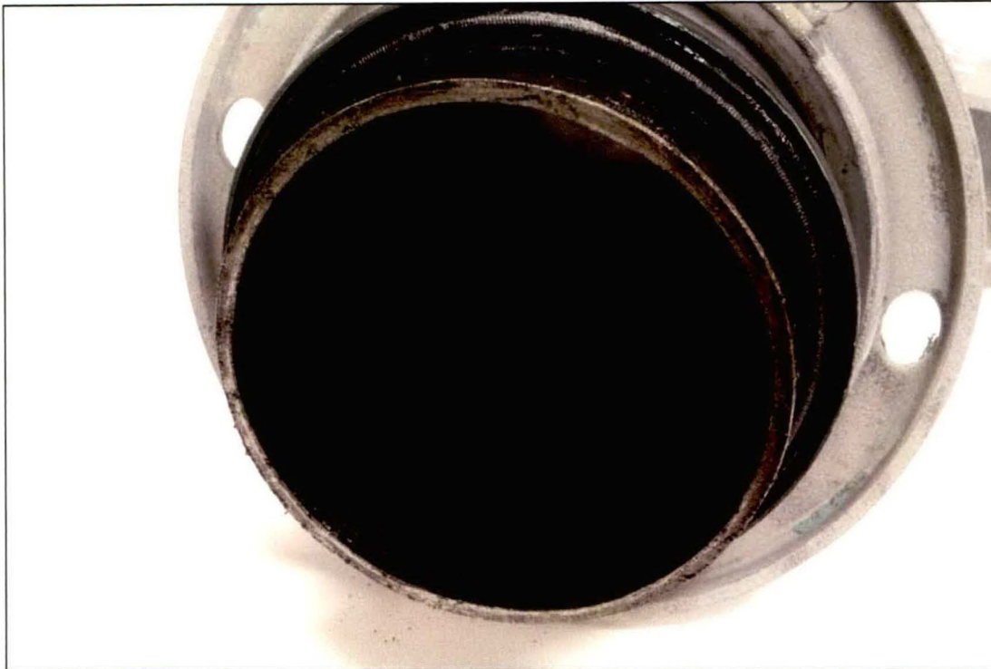
Figure 12. Image of the Pipe B region that had been inside the coupling.
