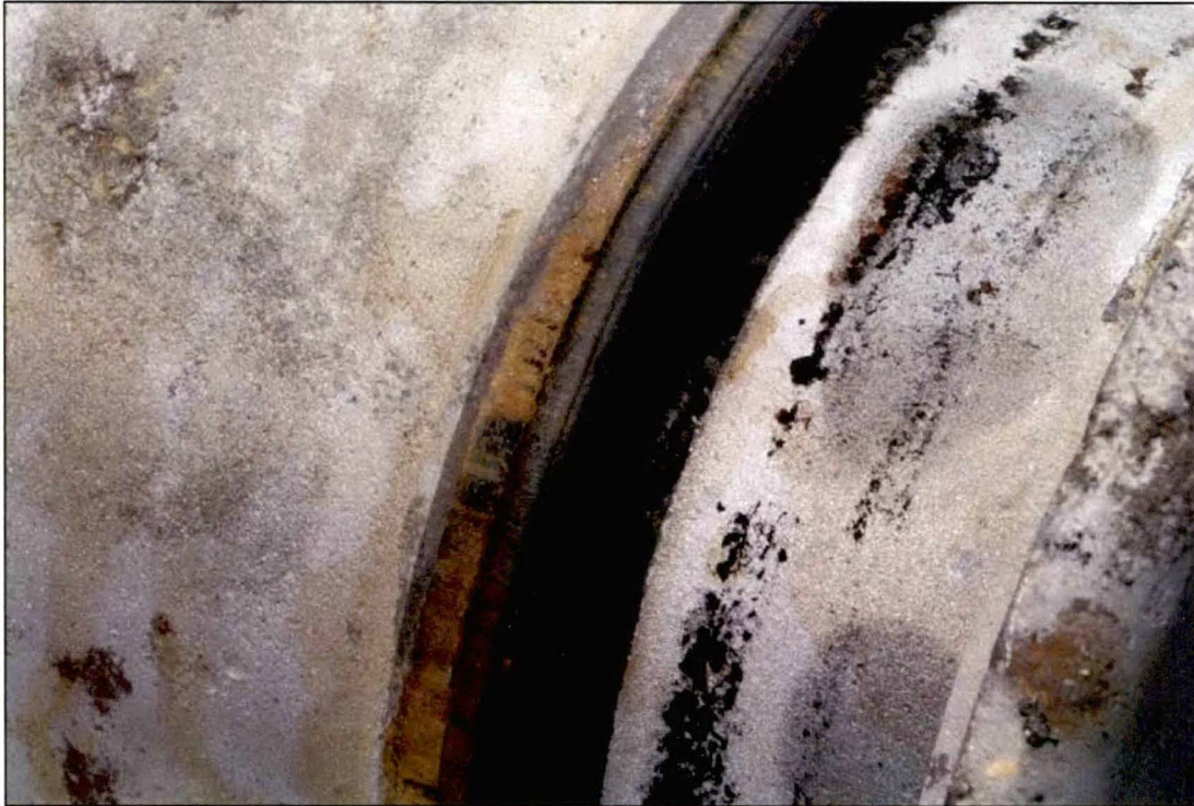
Figure 12. Photograph of the gasket at End B.
