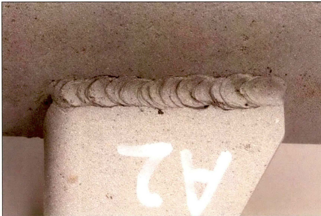
Figure 5. Image of the Lug A2 exterior top weld which exhibited substantial fusion except for some overlap and undercut.
