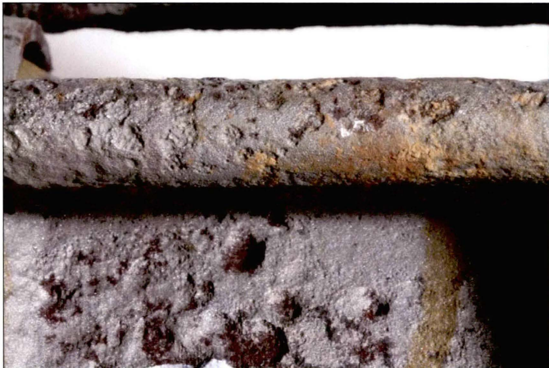
Figure 9. Image showing corrosion to a bolt and the coupling surface.
