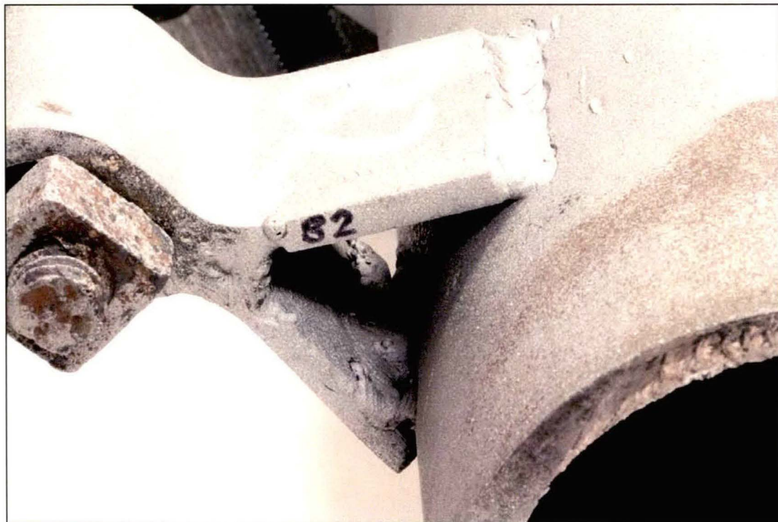
Figure 10. Oblique view of Lug B2 showing the partial weld at the bottom interior location.
