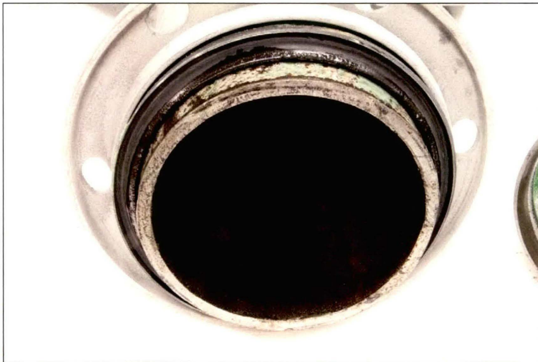
Figure 11. Image of the Pipe A region that had been inside the coupling.
