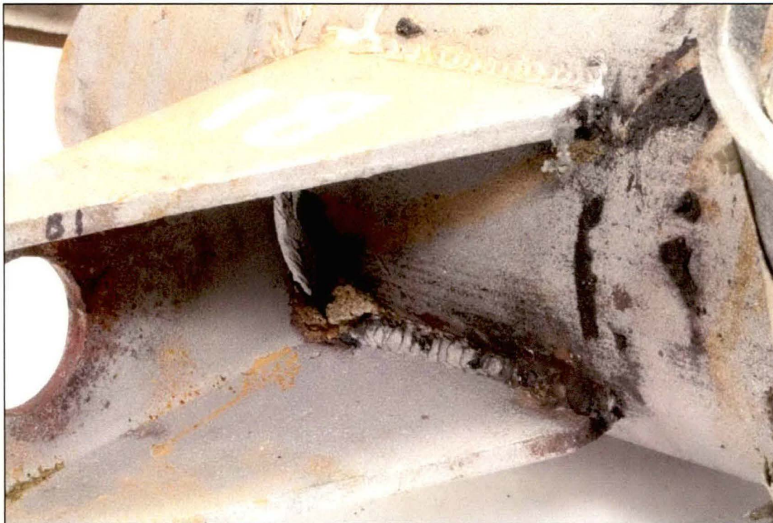
Figure 6. Image of the Lug B1 interior bottom weld which exhibited substantial fusion but was incompletely sand blasted.
