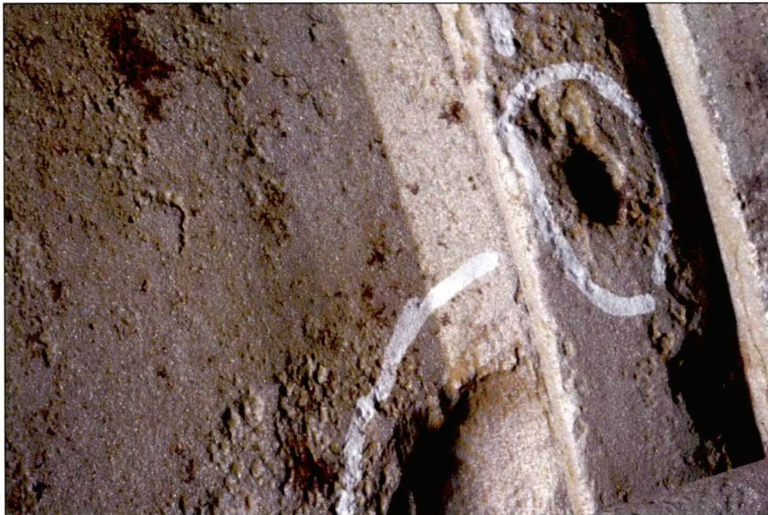
Figure 4. Image of a circled corrosion pit on the coupling identified as Location 1.
