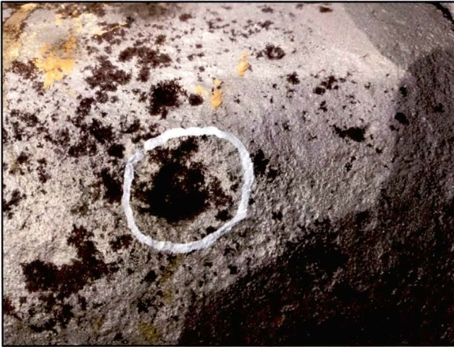
Figure 7- Severe Corrosion on Pipe A
