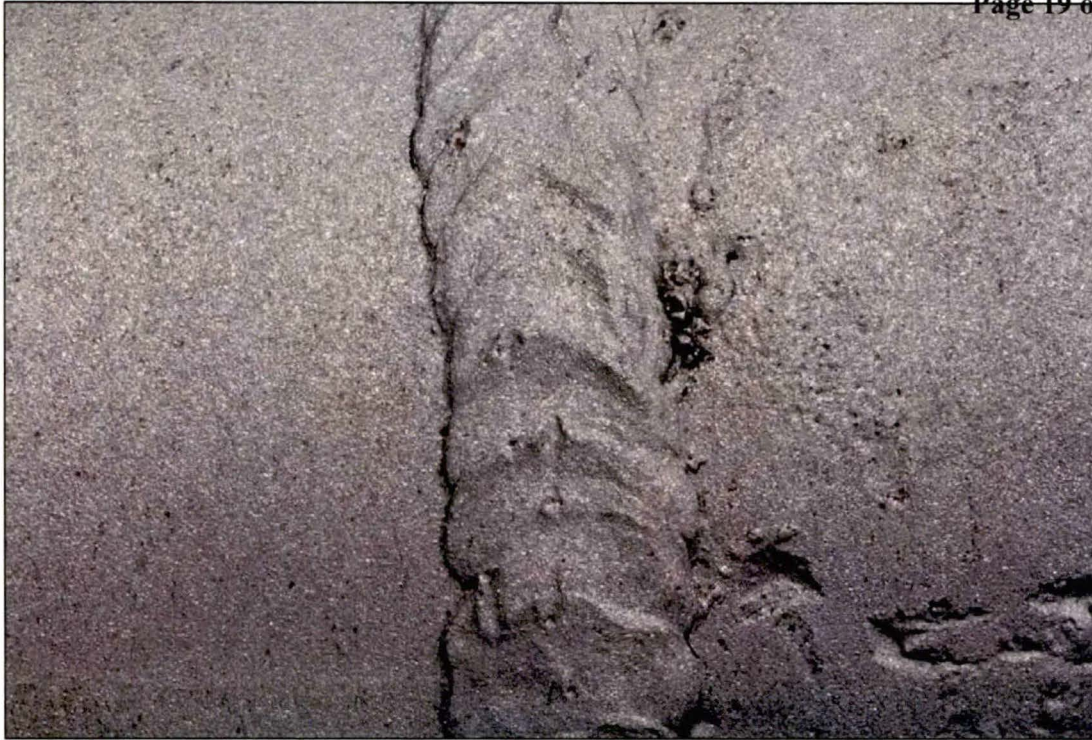
Figure 13. Photograph of a representative region of the circumferential weld on Section A.
