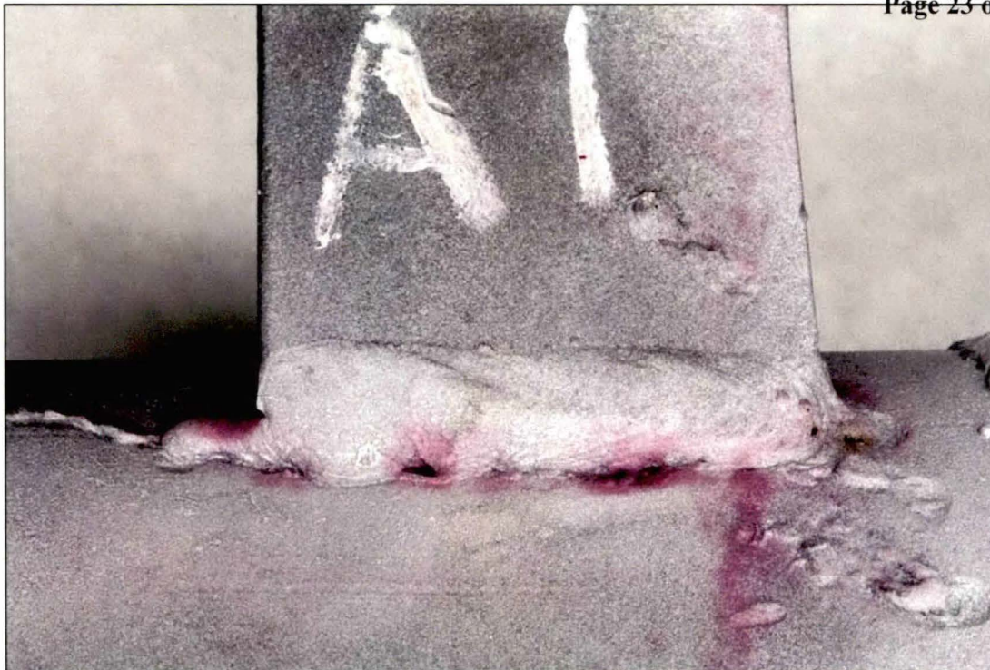
Figure 17. Image of the Lug A1 exterior top weld after dye penetrant media had been used during inspection.
