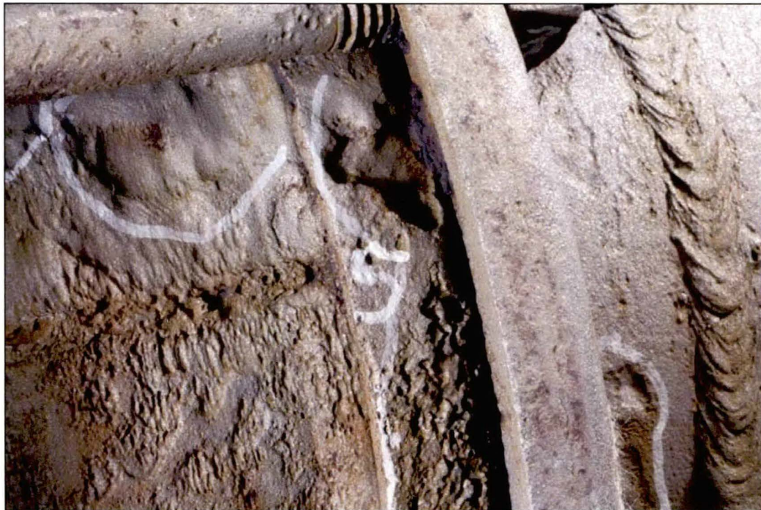
Figure 8. Image of a circled corrosion pit on the coupling identified as Location 5.
