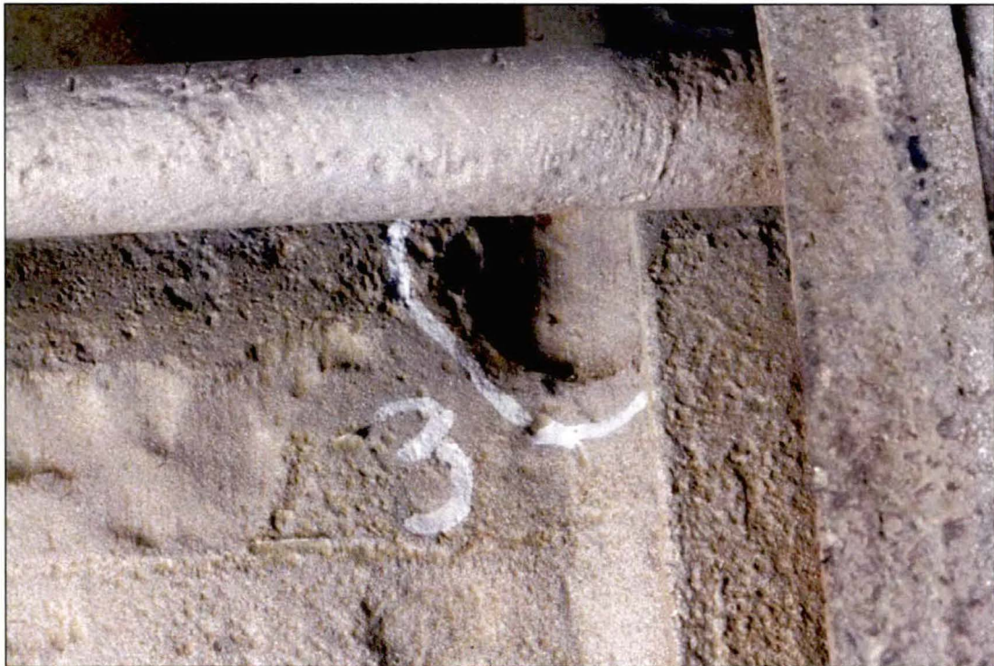
Figure 6. Image of a circled corrosion pit on the coupling identified as Location 3.
