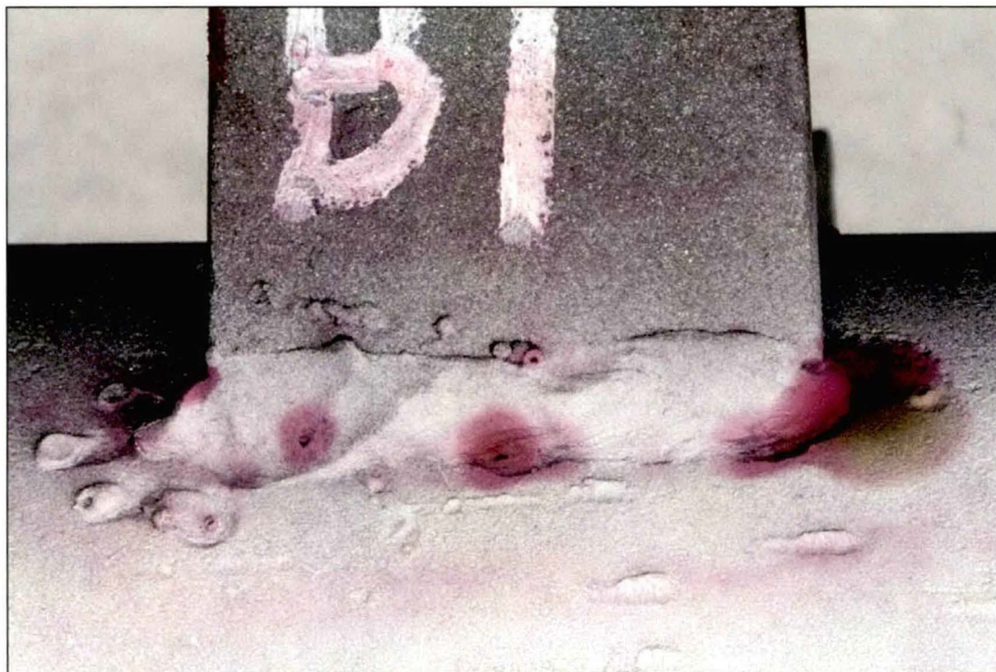
Figure 18. Image of the Lug B1 exterior top weld after dye penetrant media had been used during inspection.
