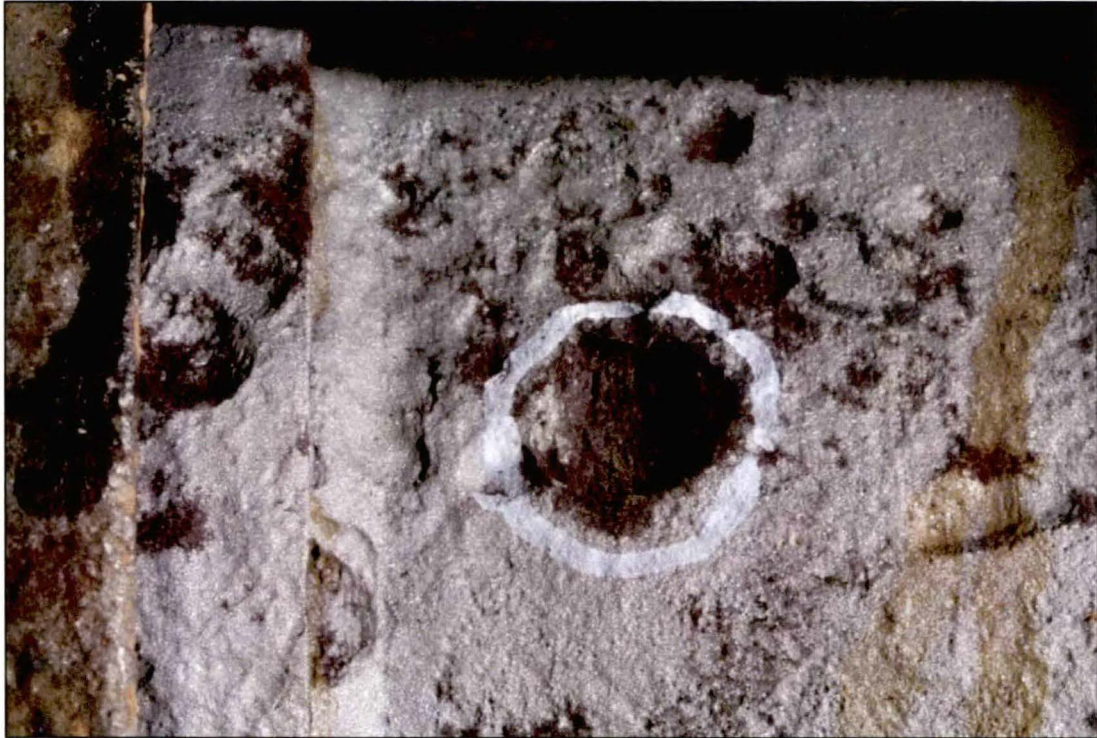
Figure 8. Photograph of an additional deep corrosion pit on the bottom of the coupling.
