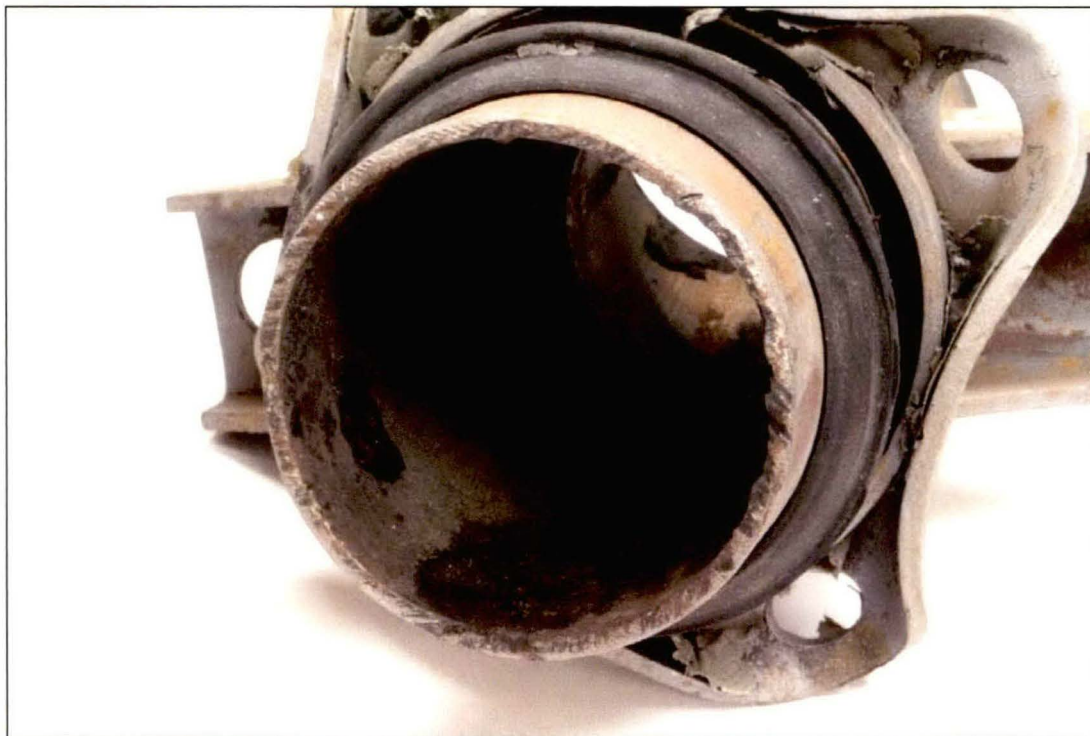
Figure 9. Image of the Pipe B section which had been in the coupling.
