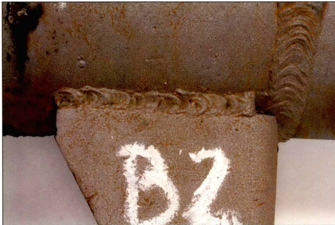
Figure 5. Image of the Lug B2 exterior top weld which exhibited substantial fusion except for some overlap.
