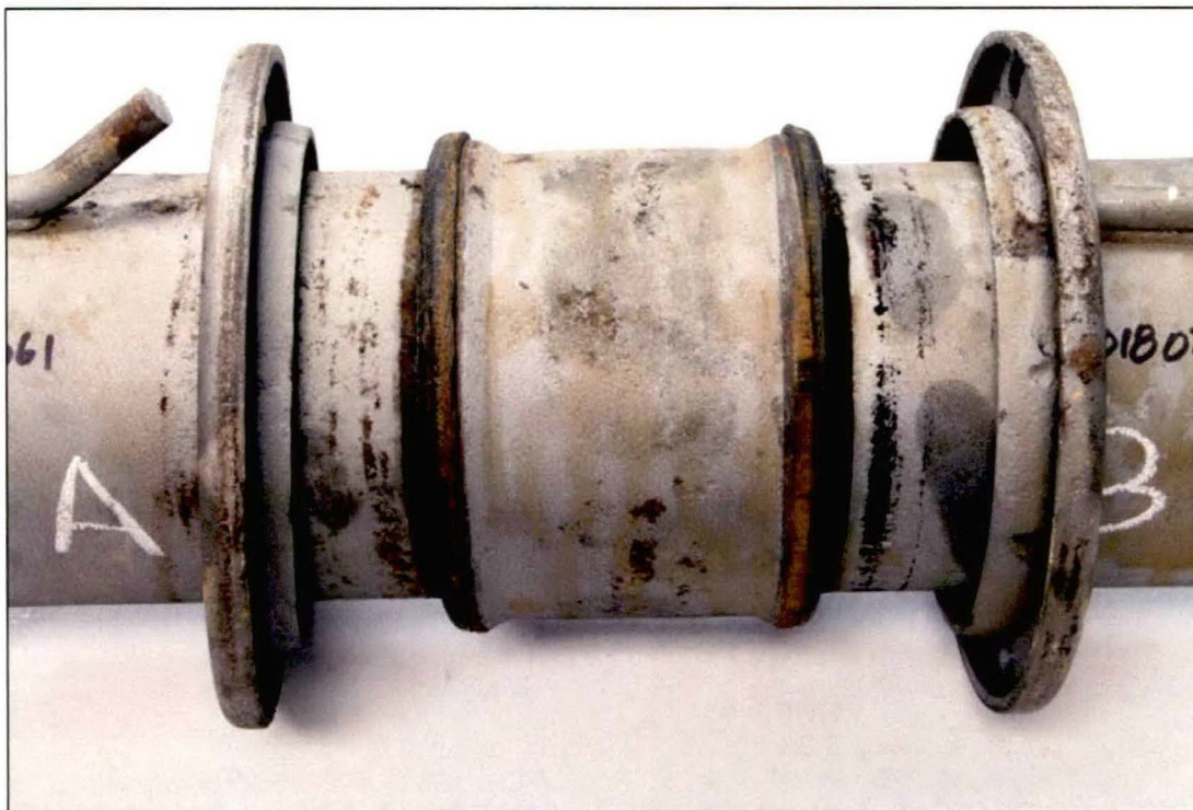
Figure 10. Photograph of the pipe sample after disassembly of the coupling. The ends of the pipe segments could not be removed from the coupling.
