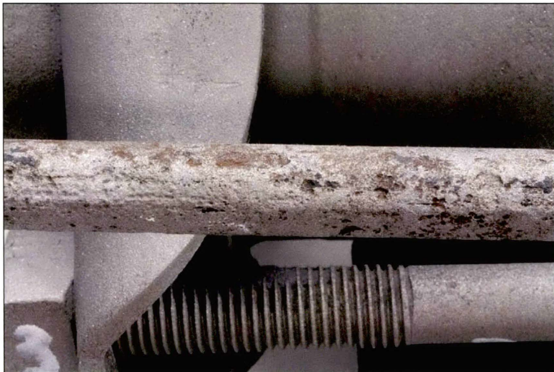
Figure 12. Slight corrosion was apparent on an attachment rod in this location.
