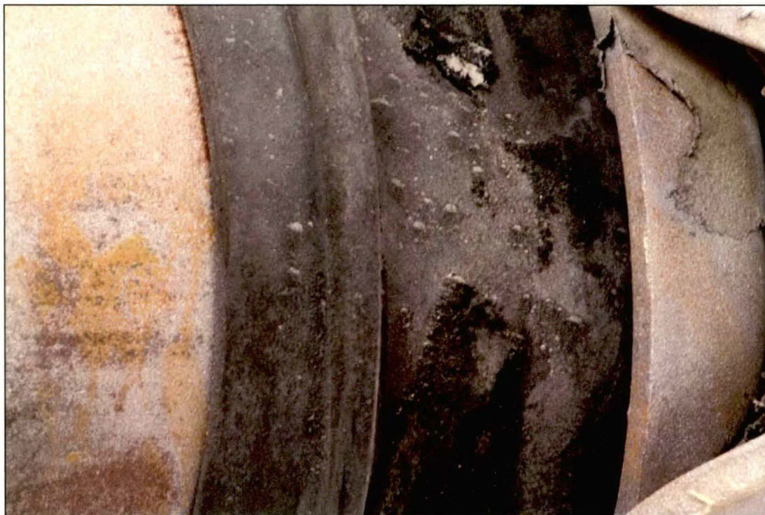
Figure 11. Close-up image of the condition of the elastomeric seal within the coupling.
