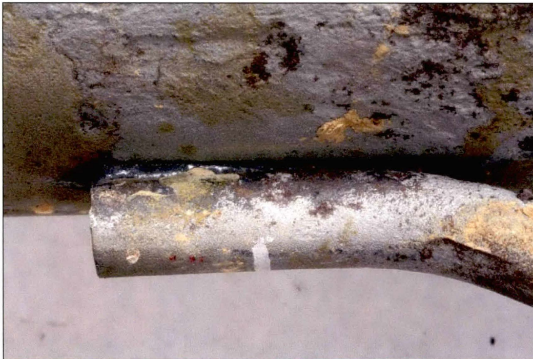
Figure 5. Image of the Rod Side A bottom joint region showing the absence of a weld.
