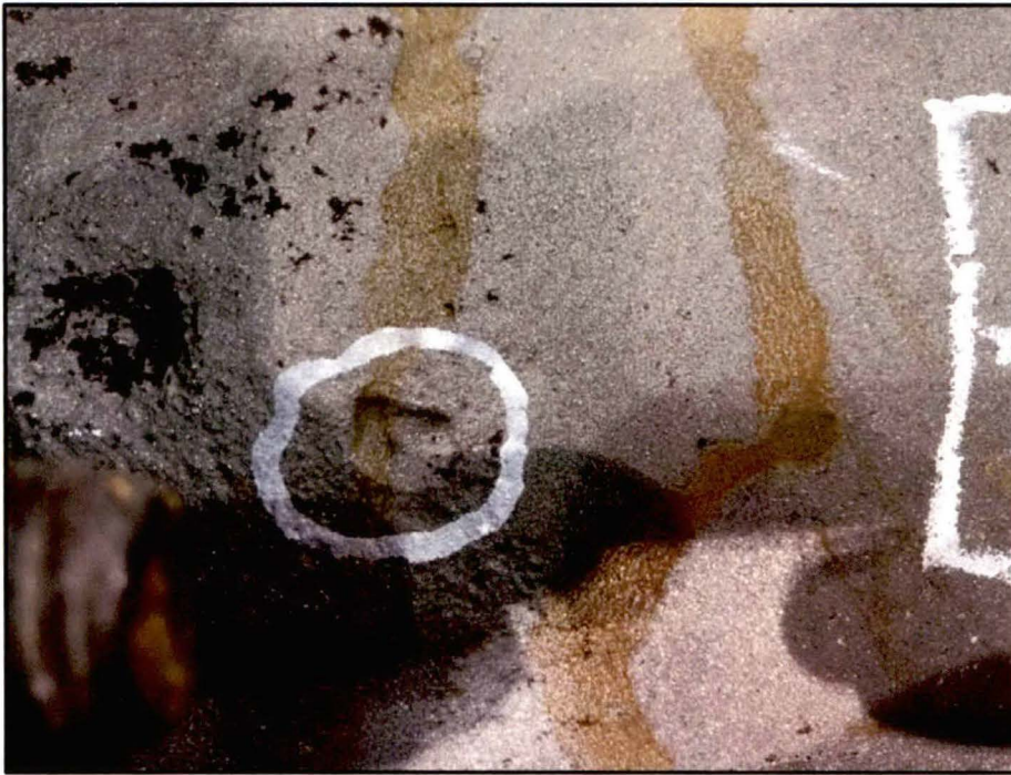
Figure 8- Moderate Corrosion on Pipe B
