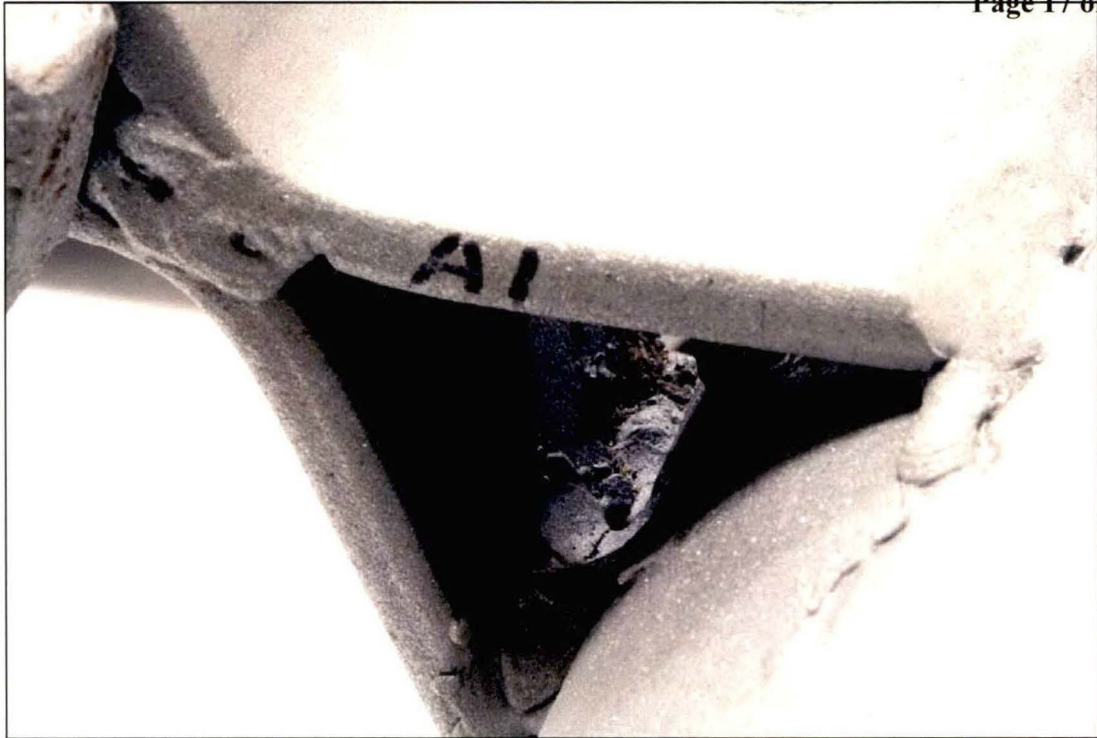
Figure 9. Oblique view of Lug A1 showing the partial weld at the bottom interior location.
