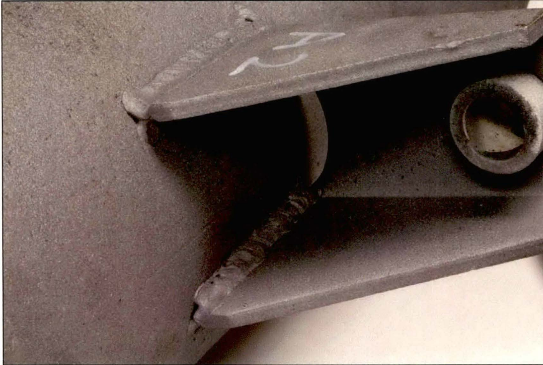
Figure 8. Image of the Lug A2 interior bottom weld which exhibited substantial fusion except for some overlap, and undercut.
