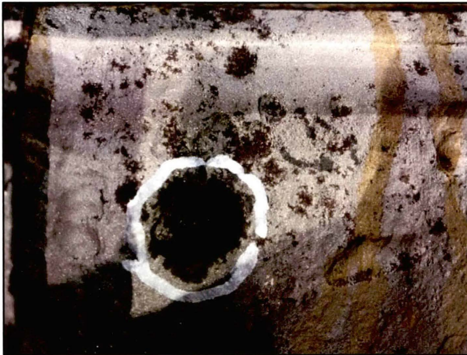
Figure 9- Severe Corrosion on Coupler
