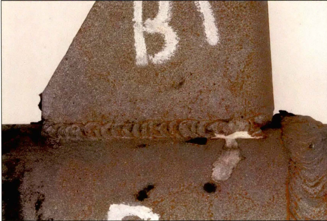
Figure 4. Image of the Lug B1 exterior top weld which exhibited substantial fusion except for some overlap.
