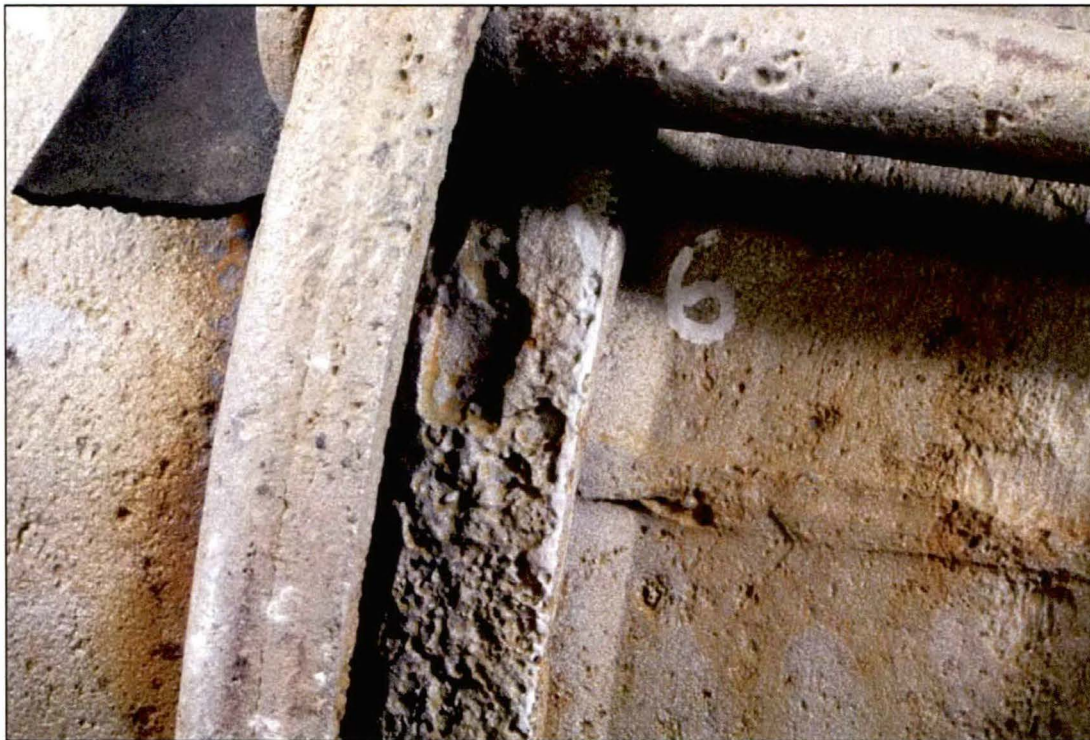
Figure 9. Image of a circled corrosion pit on the coupling identified as Location 6.
