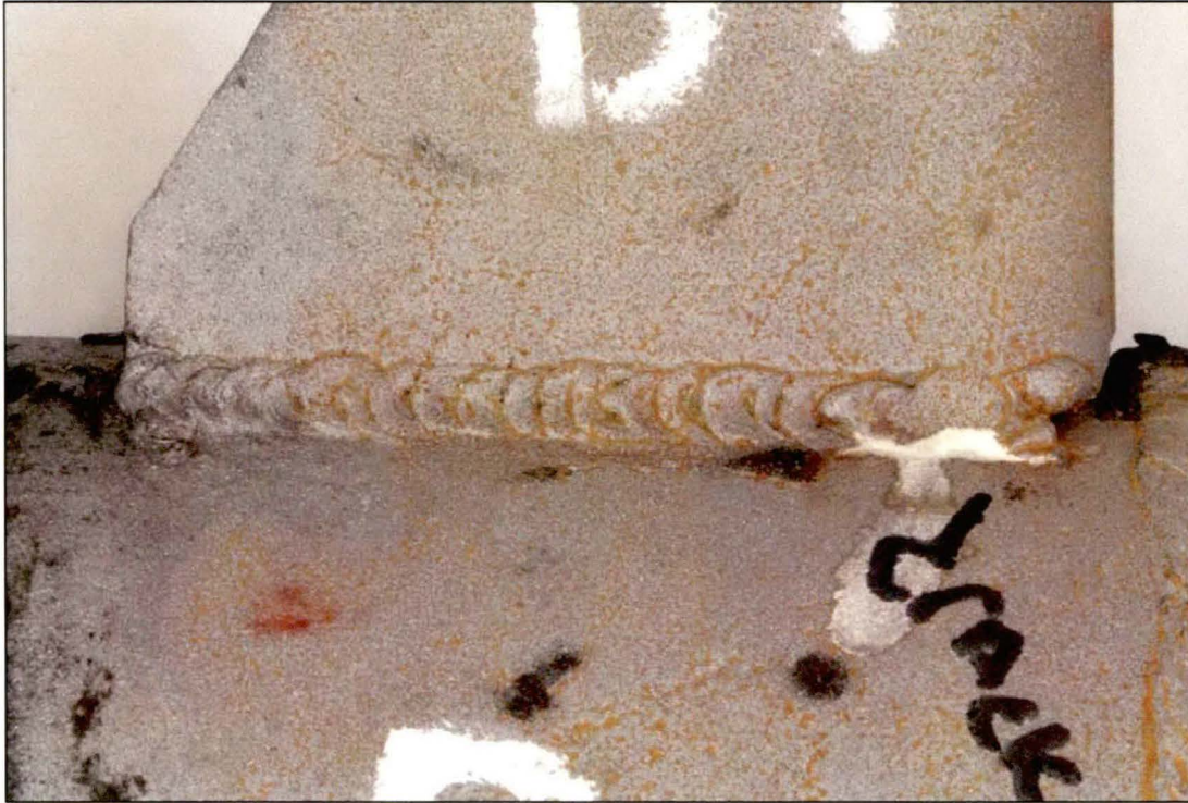
Figure 12. Image of the Lug B1 exterior top weld after magnetic particle media had been used during inspection.
