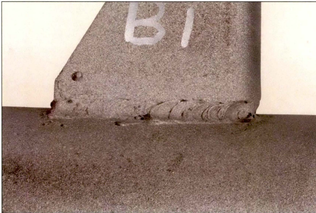
Figure 7. Image of the Lug B1 exterior bottom weld which exhibited substantial fusion except for some overlap, undercut, and spatter.
