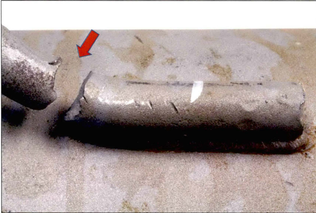
Figure 4. Image of the Rod Side B top joint region showing the attachment weld. The rod fracture site is indicated by an arrow.
