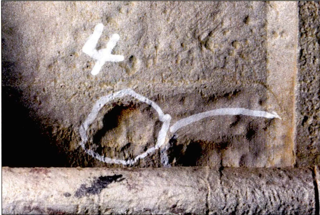
Figure 7. Image of a circled corrosion pit on the coupling identified as Location 4.
