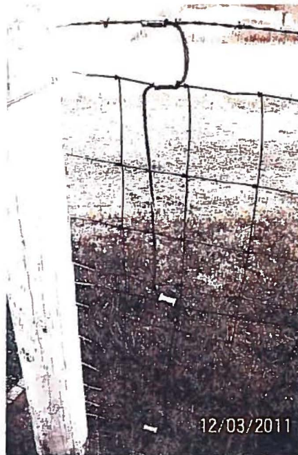
Figure 50 - Fence Grounding at House
