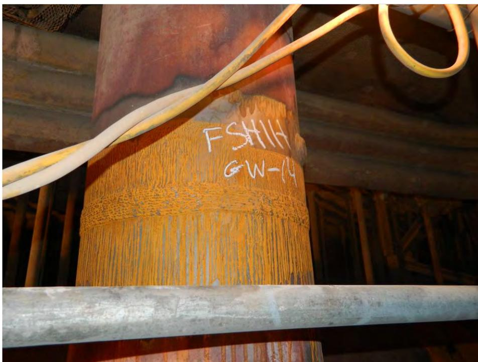
Fig. 39. Photographs of girth weld Nos. GW-13 and GW-14 on the Finishing Superheater Inlet header
