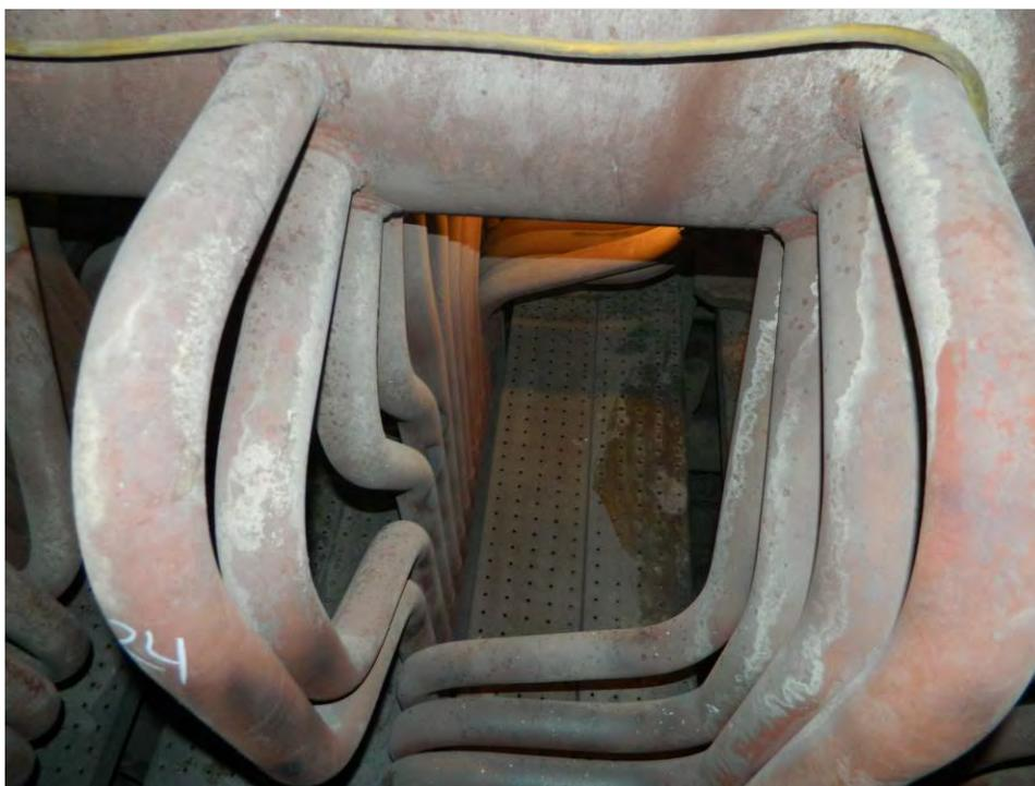
Fig. 16. Photographs of the Platen Superheater Outlet header tubing.
