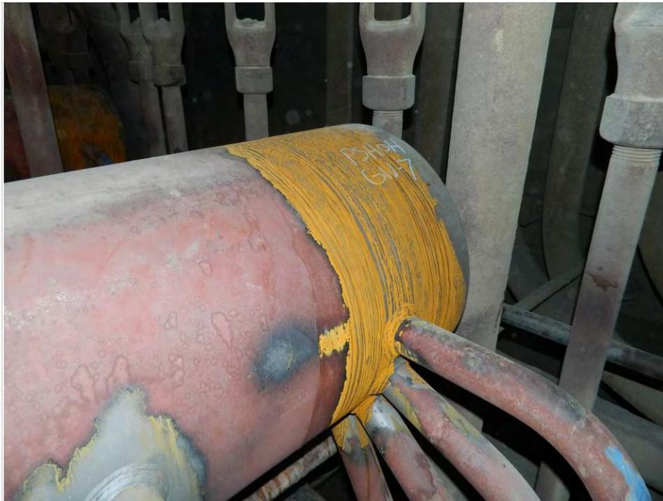
Fig. 19. Photographs of girth weld Nos. GW-6 and GW-7 on the Platen Superheater Outlet header.
