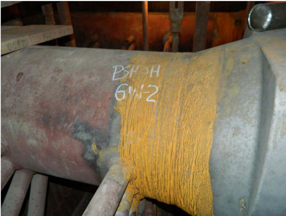
Fig. 17. Photographs of girth weld Nos. GW-1 and GW-2 on the Platen Superheater Outlet header.
