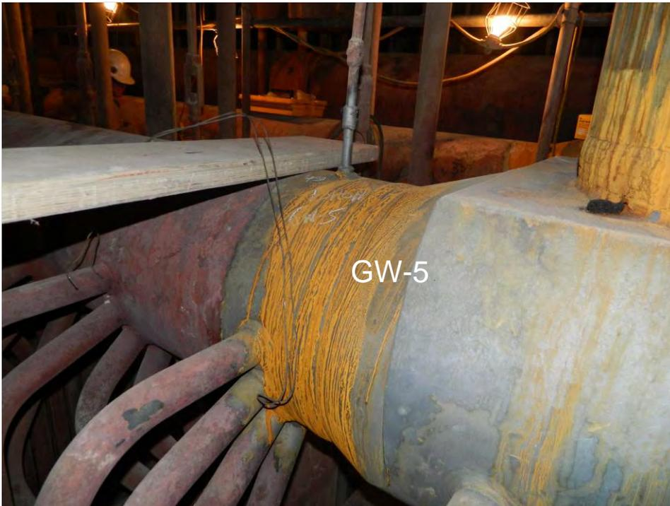
Fig. 18. Photographs of girth weld Nos. GW-4 and GW-5 on the Platen Superheater Outlet header.
