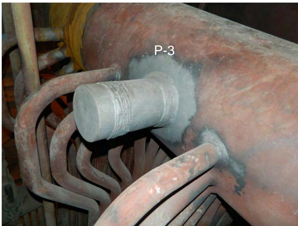
Fig. 33. Photographs of girth weld No. GW-1 and penetration Nos. P-1 and P-3 on the Finishing Superheater Inlet header.
