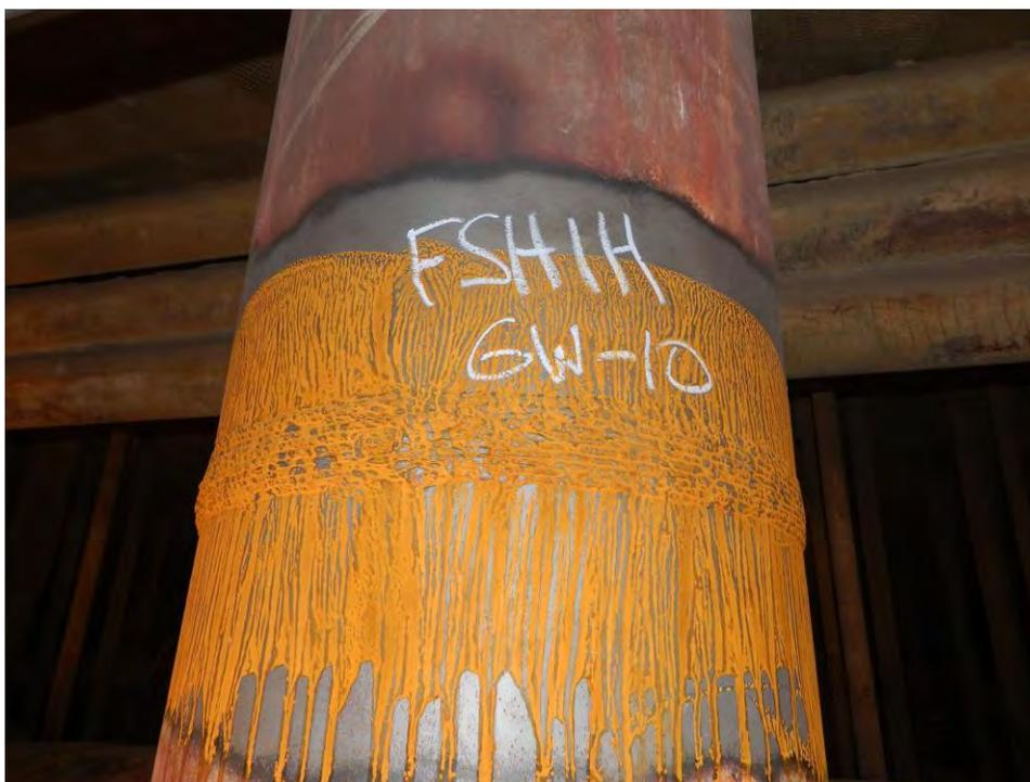
Fig. 37. Photographs of girth weld Nos.GW-9 and GW-10 on the Finishing Superheater Inlet header.
