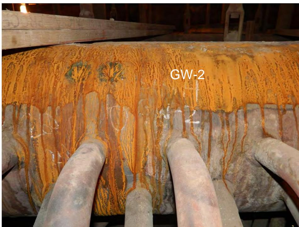
Fig. 5. Photographs of girth weld Nos. GW-1 and GW-2 on the Platen Superheater Inlet header.
