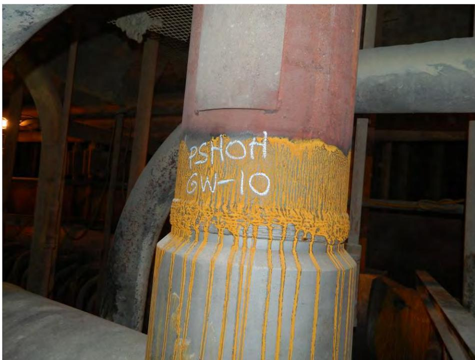
Fig. 20. Photographs of girth weld Nos. GW-8 and GW-10 on the Platen Superheater Outlet header.
