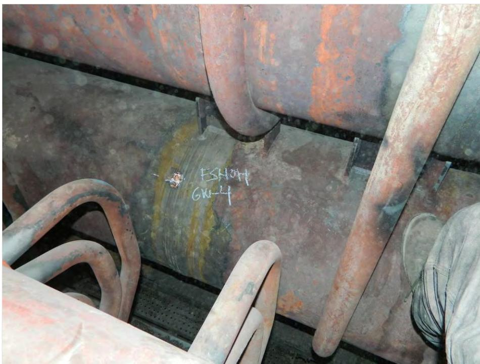
Fig. 54. Photographs of girth weld Nos. GW-3 and GW-4 on the Lower Finishing Superheater Outlet header.
