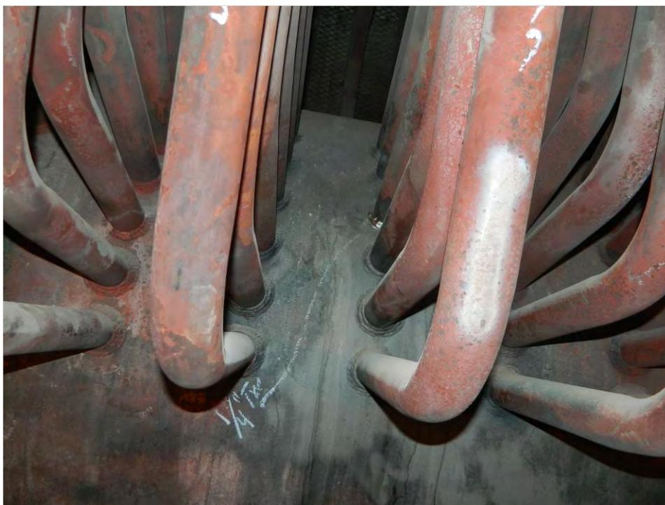
Fig. 91. Photographs of the indications on the tube stubs of the LP Reheat Outlet header.
