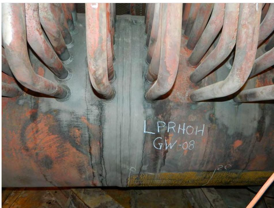
Fig. 87. Photographs of girth weld Nos. GW-7 and GW-8 on the LP Reheat Outlet header.
