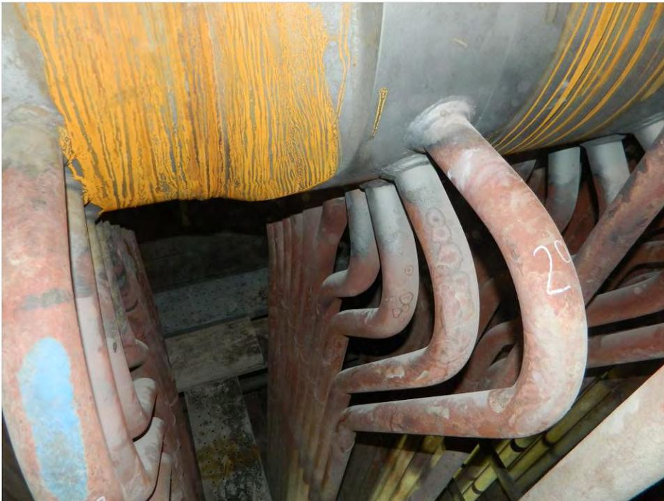
Fig. 32. Photographs of the Finishing Superheater Inlet header and tubing.
