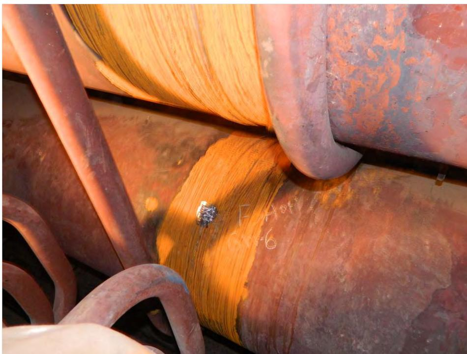
Fig. 55. Photographs of girth weld Nos. GW-5 and GW-6 on the Lower Finishing Superheater Outlet header.
