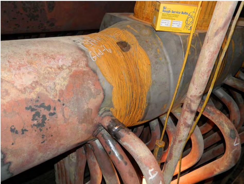
Fig. 35. Photographs of girth weld Nos. GW-5 and GW-6 on the Finishing Superheater Inlet header.
