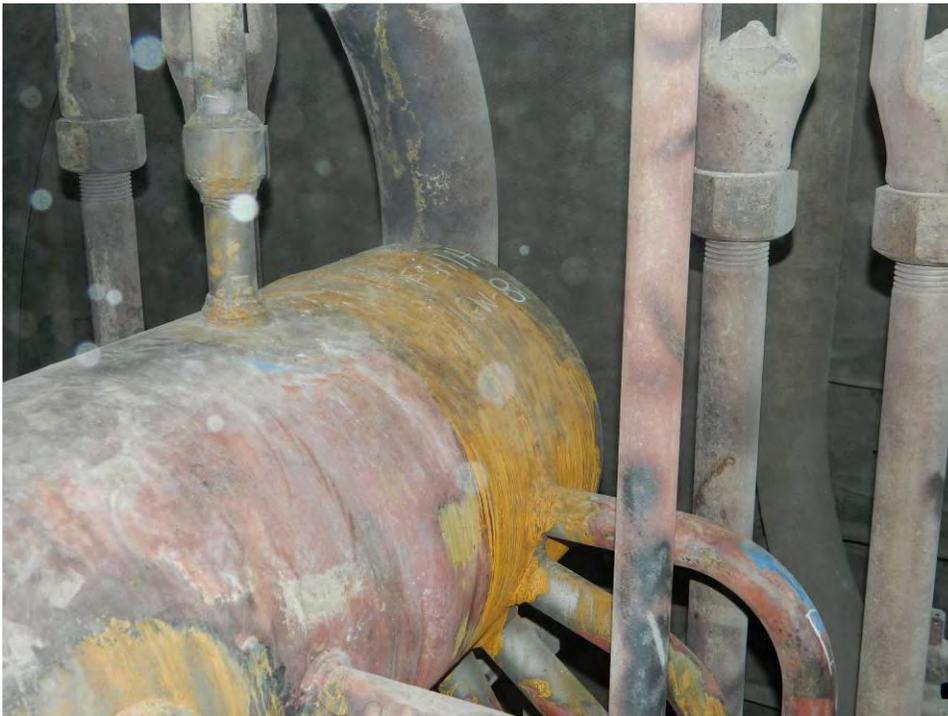
Fig. 36. Photographs of girth weld Nos. GW-7 and GW-8 on the Finishing Superheater Inlet header.
