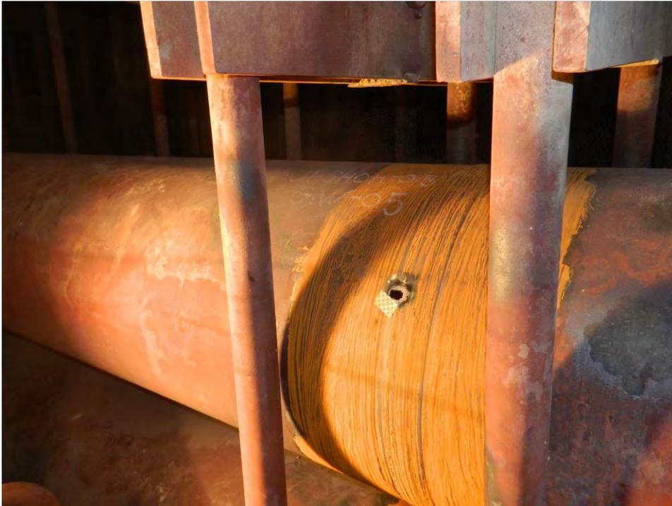
Fig. 51. Photographs of girth weld Nos. GW-4 and GW-5 on the Upper Finishing Superheater Outlet header.
