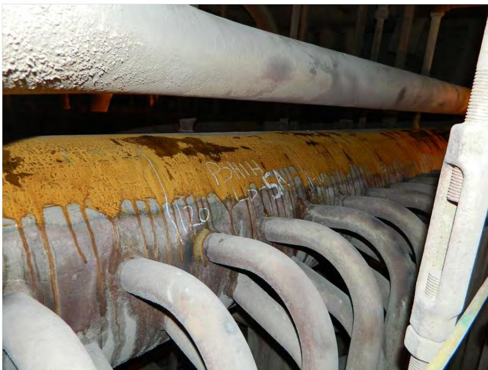
Fig. 4. Photographs of seam weld Nos. LS-4A and LS-5A on the Platen Superheater Inlet header.
