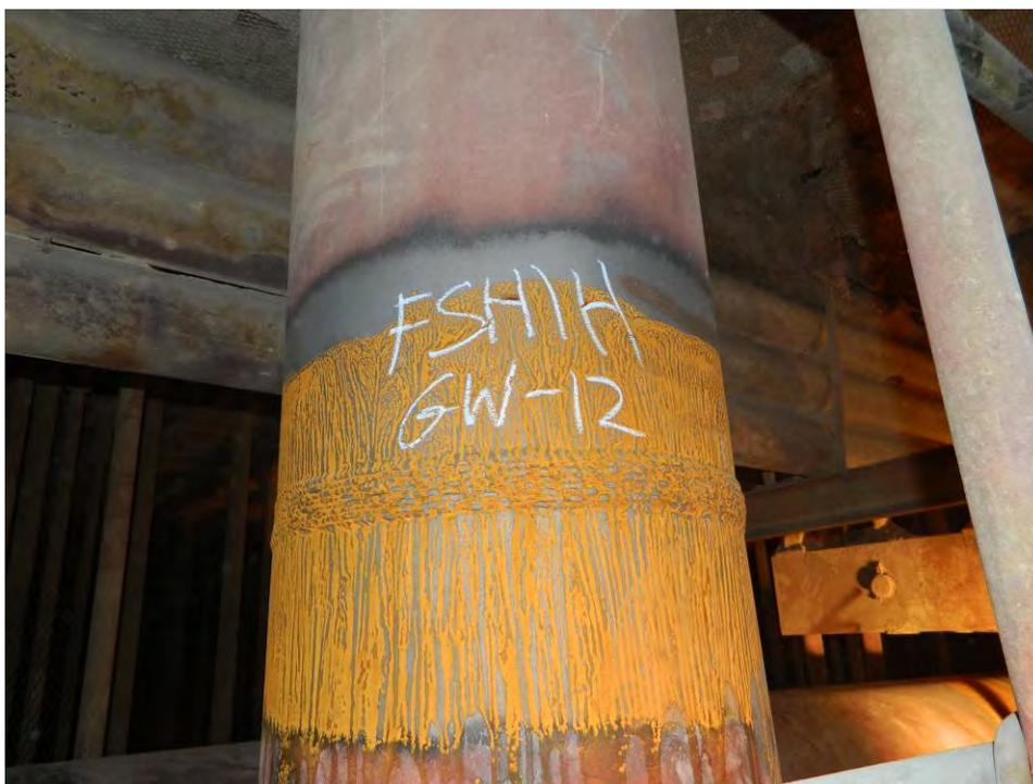
Fig. 38. Photographs of girth weld Nos.GW-11 and GW-12 on the Finishing Superheater Inlet header.
