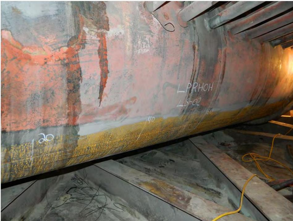
Fig. 88. Photographs of seam weld Nos.LS-01 and LS-02 on the LP Reheat Outlet header.
