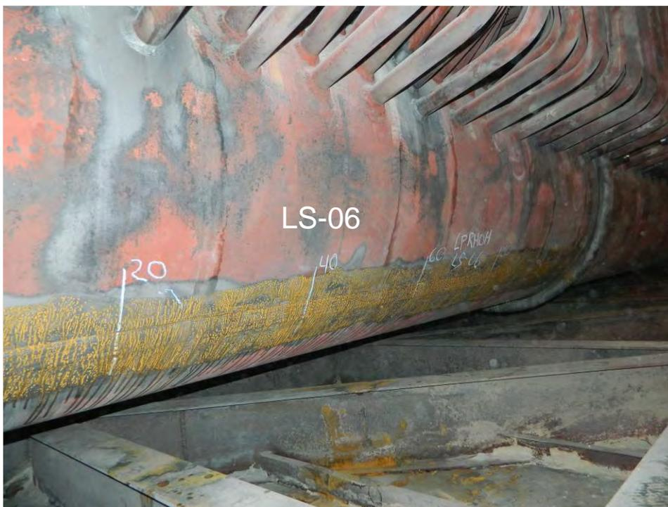
Fig. 89. Photographs of seam weld Nos.LS-04 and LS-06 on the LP Reheat Outlet header.
