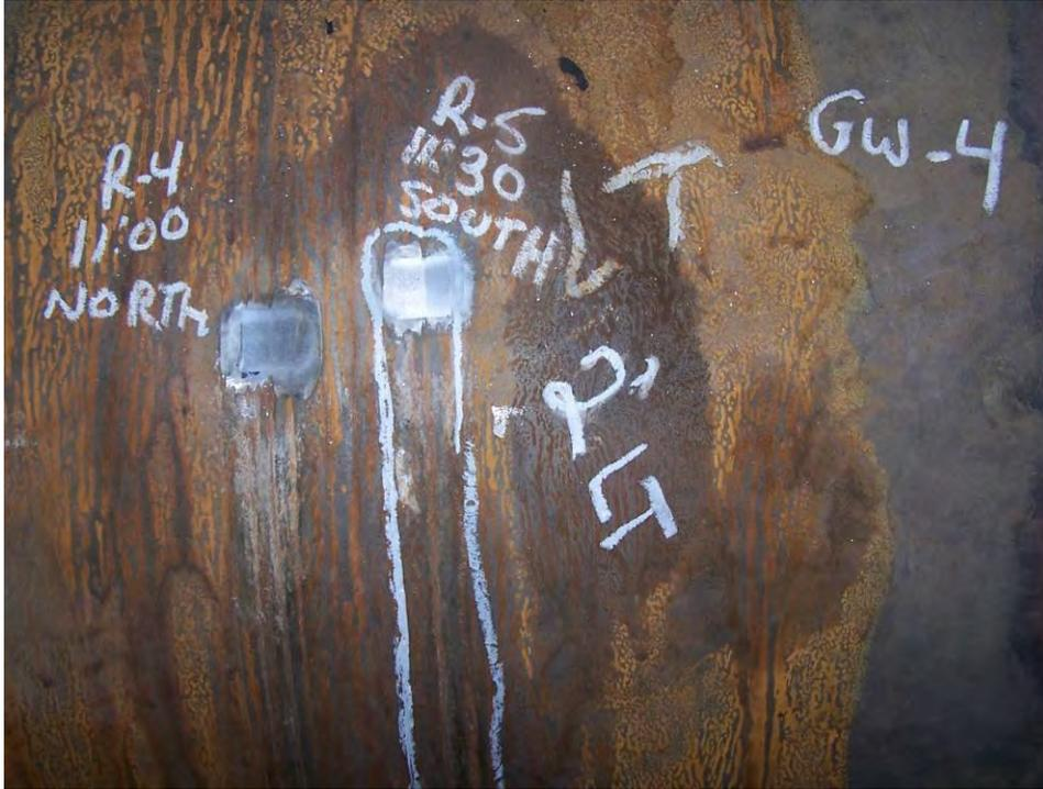
Fig. 56. Photographs of the indications in girth weld No. GW-4 on the Lower Finishing Superheater Outlet header.
