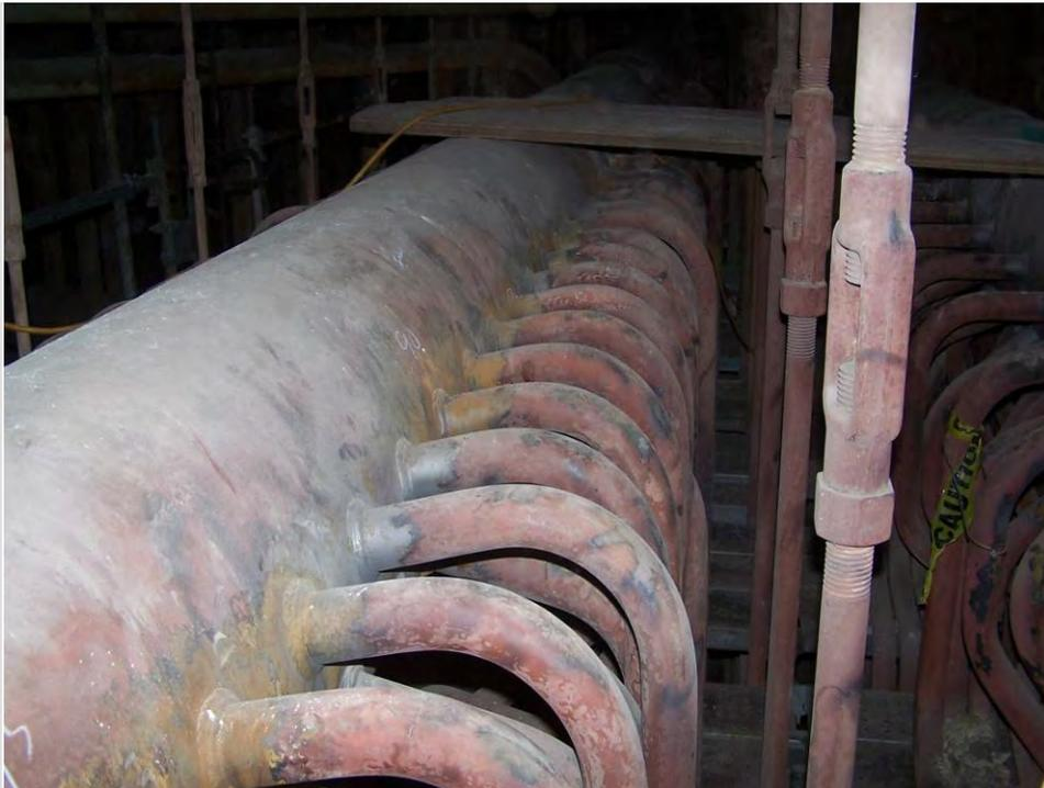
Fig. 2. Photographs of the Platen Superheater Inlet header and tubing.
