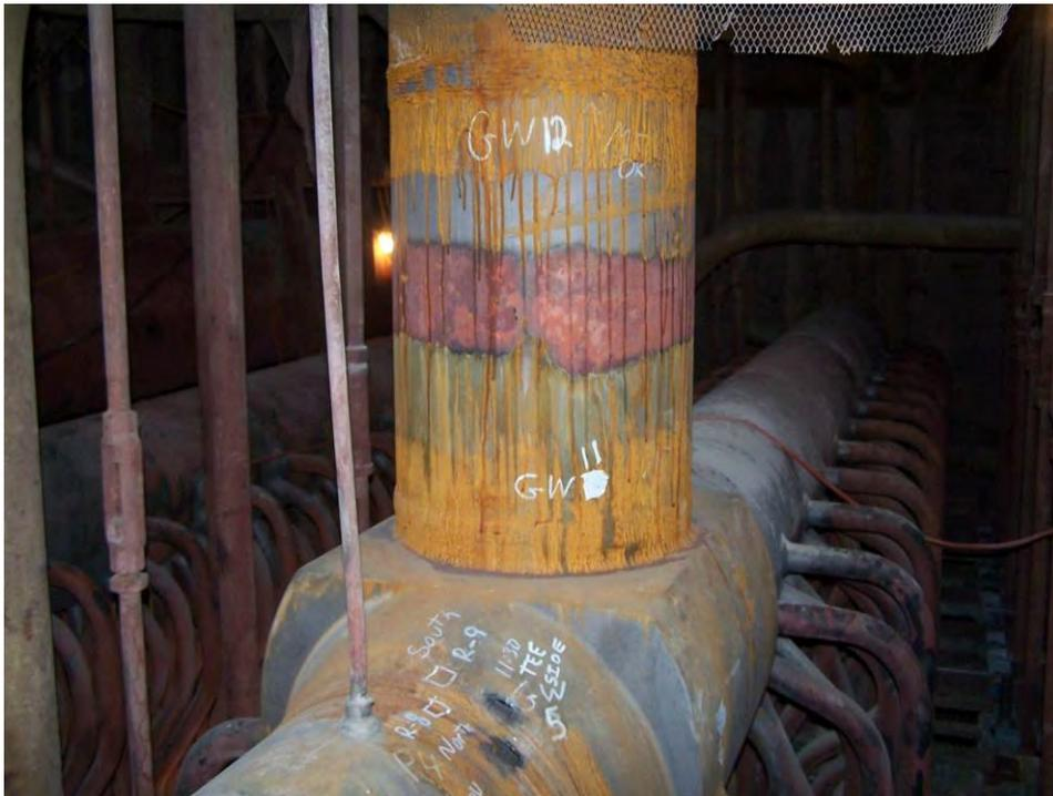
Fig. 14. Photographs of the inspection locations on the Platen Superheater Outlet header.
