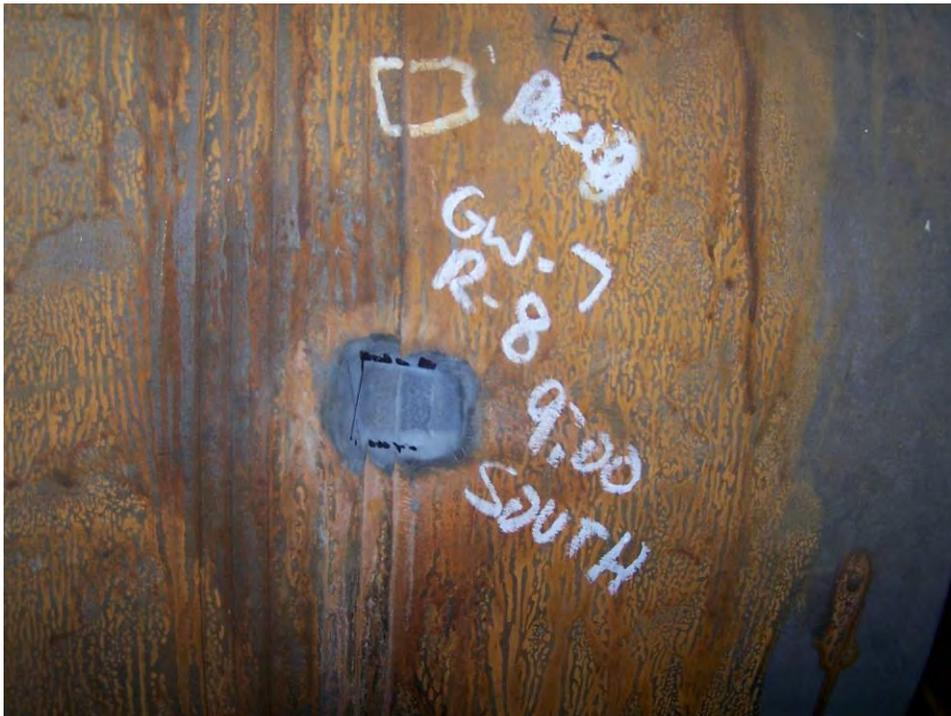
Fig. 51. Photographs of the inspection locations on the Upper Finishing Superheater Outlet header.
